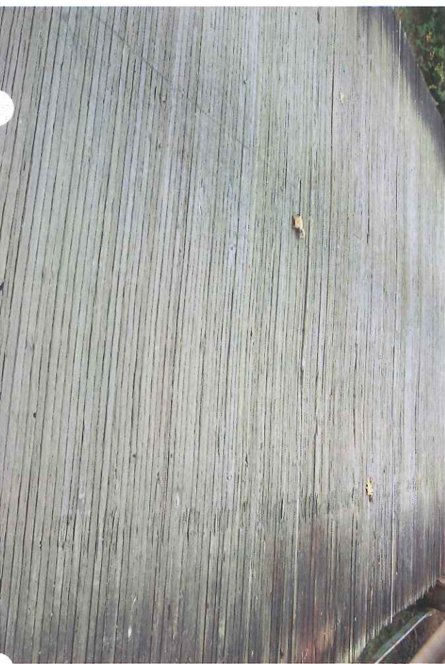
7. View of the wooden deck.
