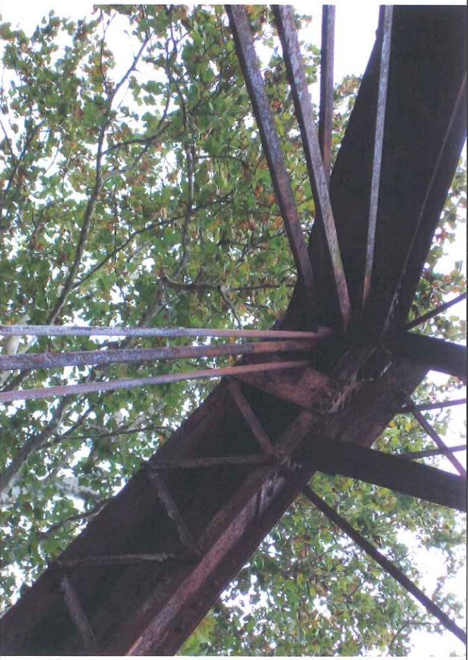
10. View of endpost connection.
