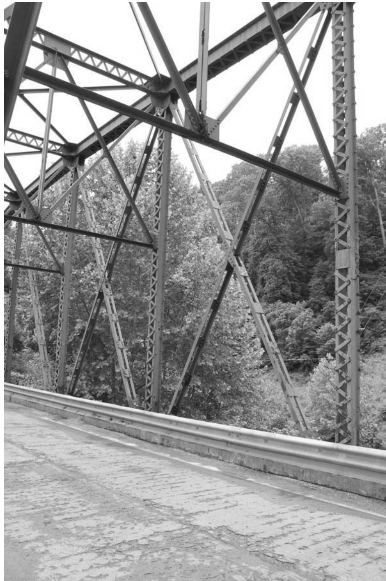
WV_Ritchie County_Cairo Bridge_0009. Detail of joining the diagonal and counter-diagonal members, facing S.
