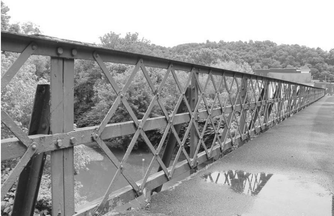
WV_Ritchie County_Cairo Bridge_0012. Detail of the bridge railing, facing SE.
