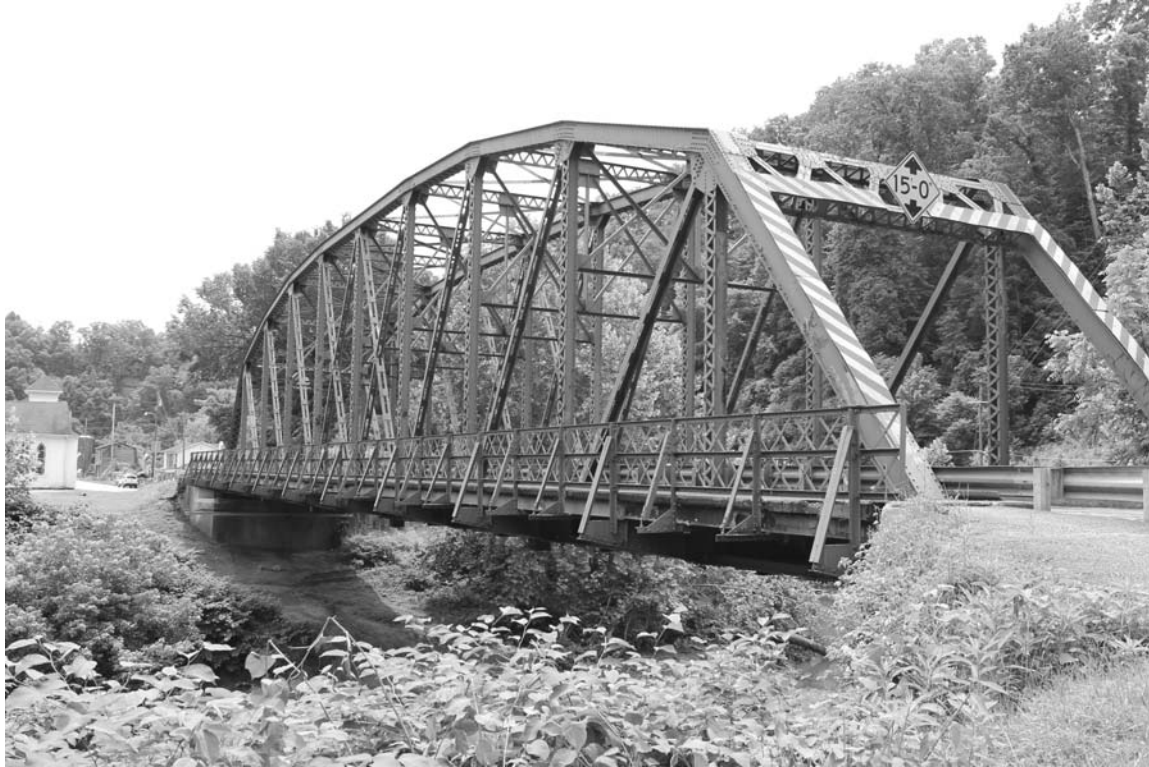
WV_Ritchie County_Cairo Bridge_0001. Elevation view, facing SE.
