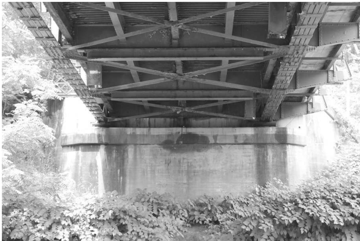
WV_Ritchie County_Cairo Bridge_0013. Southeast abutment and wingwall, facing SE.
