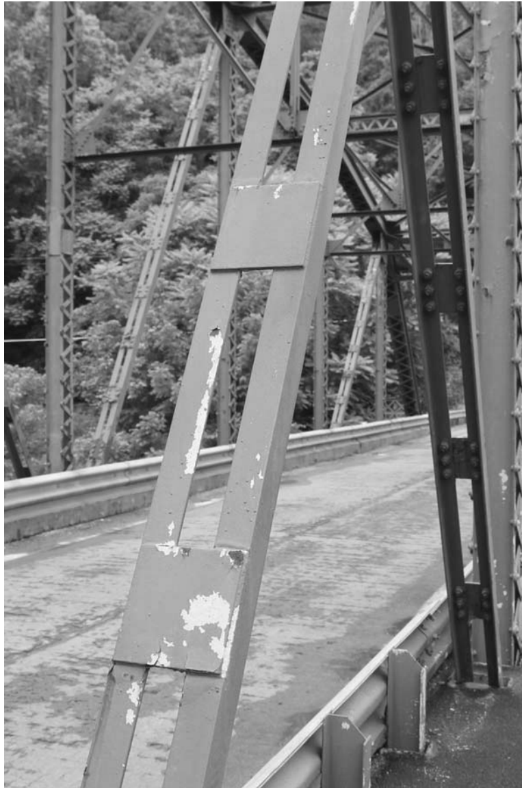
WV_Ritchie County_Cairo Bridge_0008. Detail of welded stay plates on a diagonal member, facing NW.
