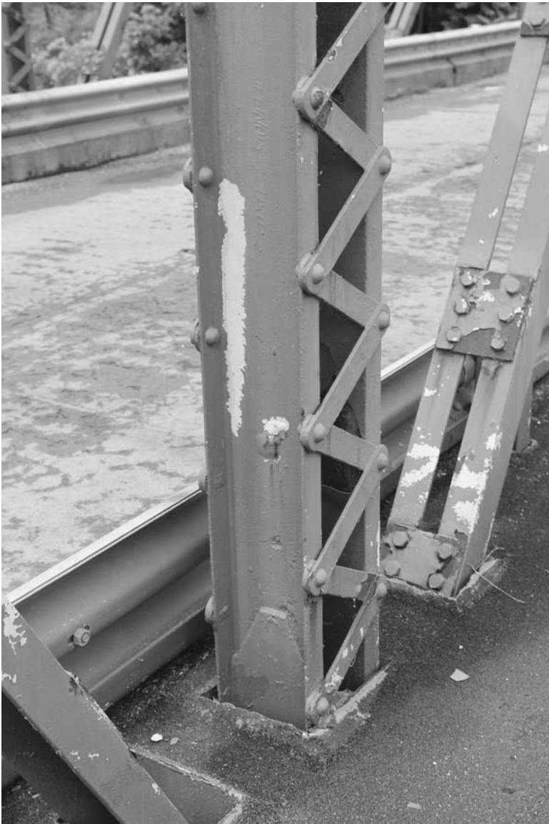
WV_Ritchie County_Cairo Bridge_0016. Representative image of a steel plate welded to a vertical, facing NW.
