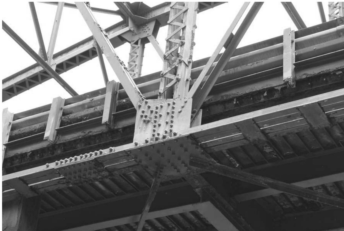
WV_Ritchie County_Cairo Bridge_0010. Lower chord panel point connection, facing N.
