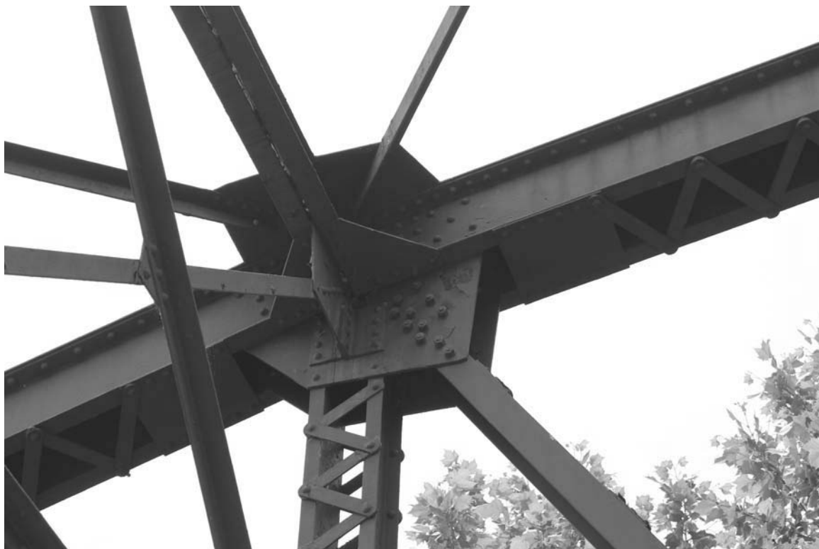
WV_Ritchie County_Cairo Bridge_0015. Upper chord panel point connection showing rivets and bolts, facing S.
