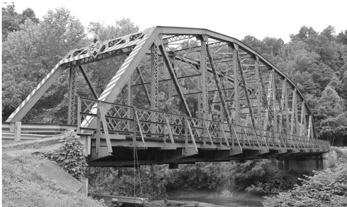
WV_Ritchie County_Cairo Bridge_0002. Elevation view, facing NW.
