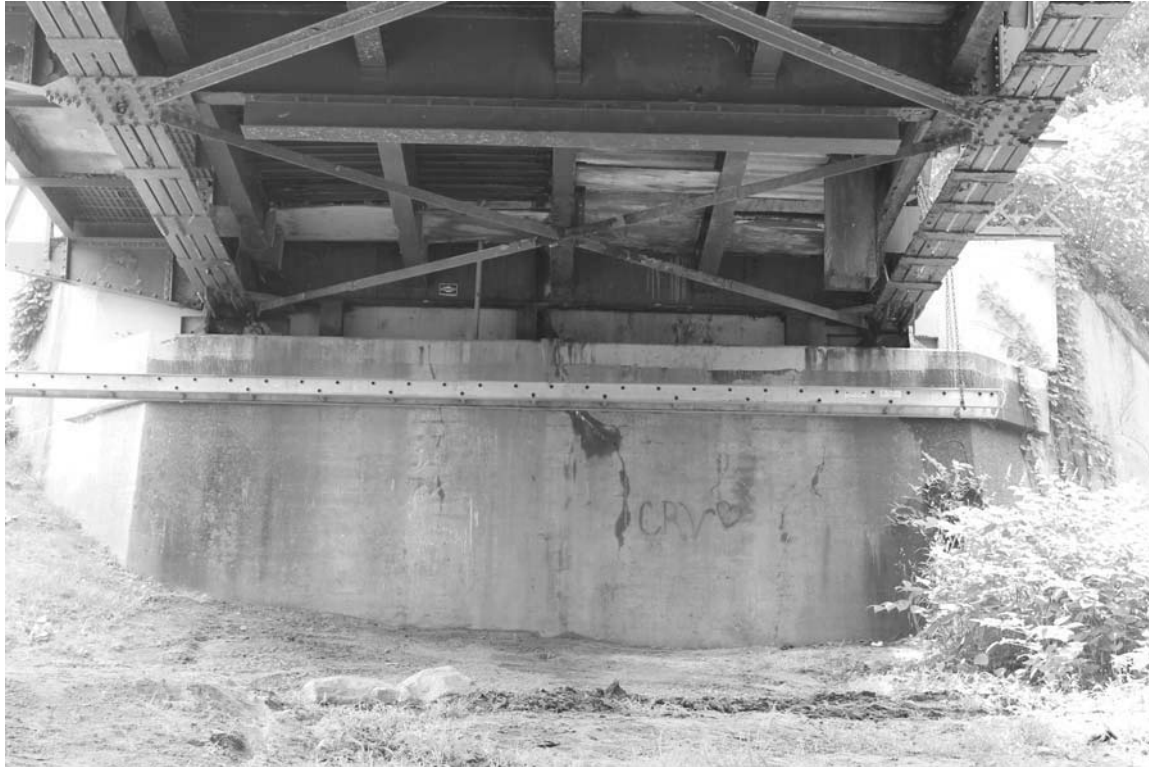
WV_Ritchie County_Cairo Bridge_0014. Northwest abutment and wingwall, facing NW.
