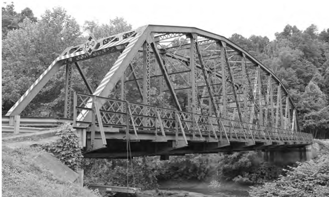
WV_Ritchie County_Cairo Bridge_0002. Elevation view, facing W.
