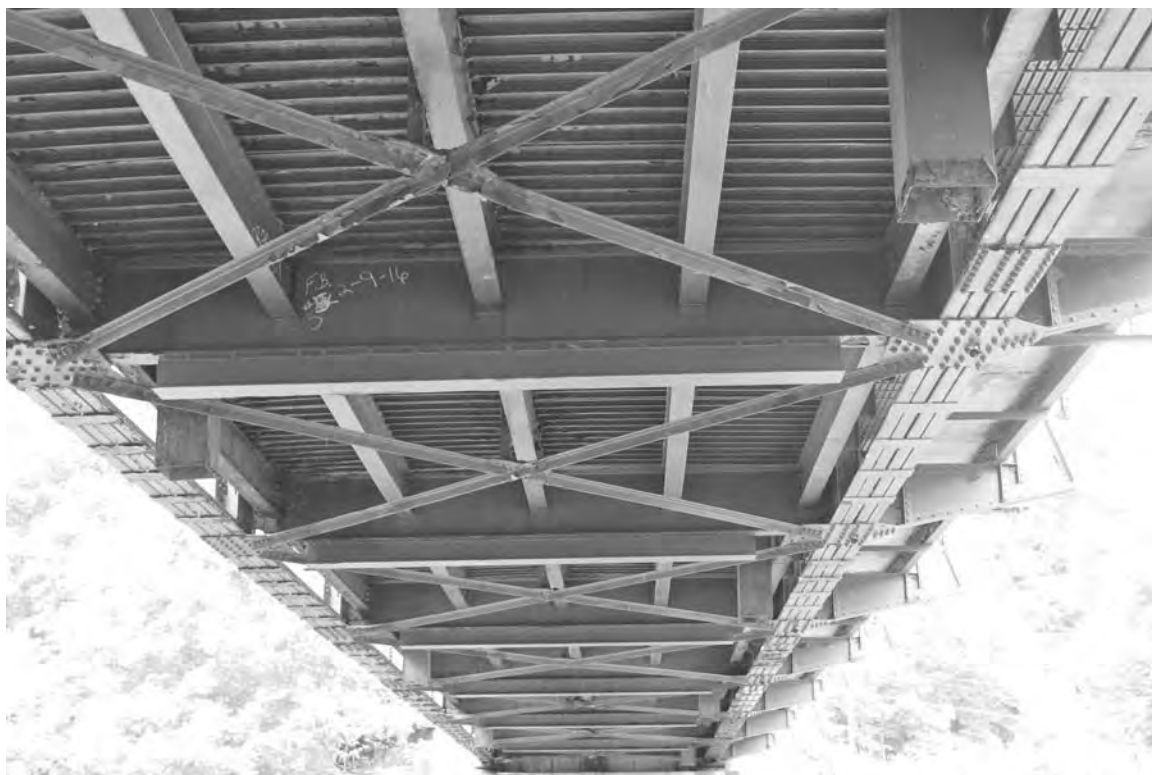
WV_Ritchie County_Cairo Bridge_0011. Underside of the bridge showing lower chords and supplemented floorbeams, facing NW.
