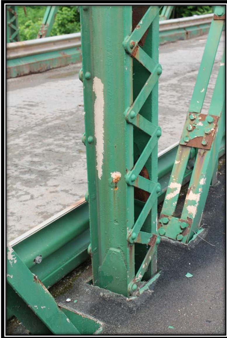
WV_Ritchie County_Cairo Bridge_0016. Representative view of a steel plate welded to a vertical, facing west.
