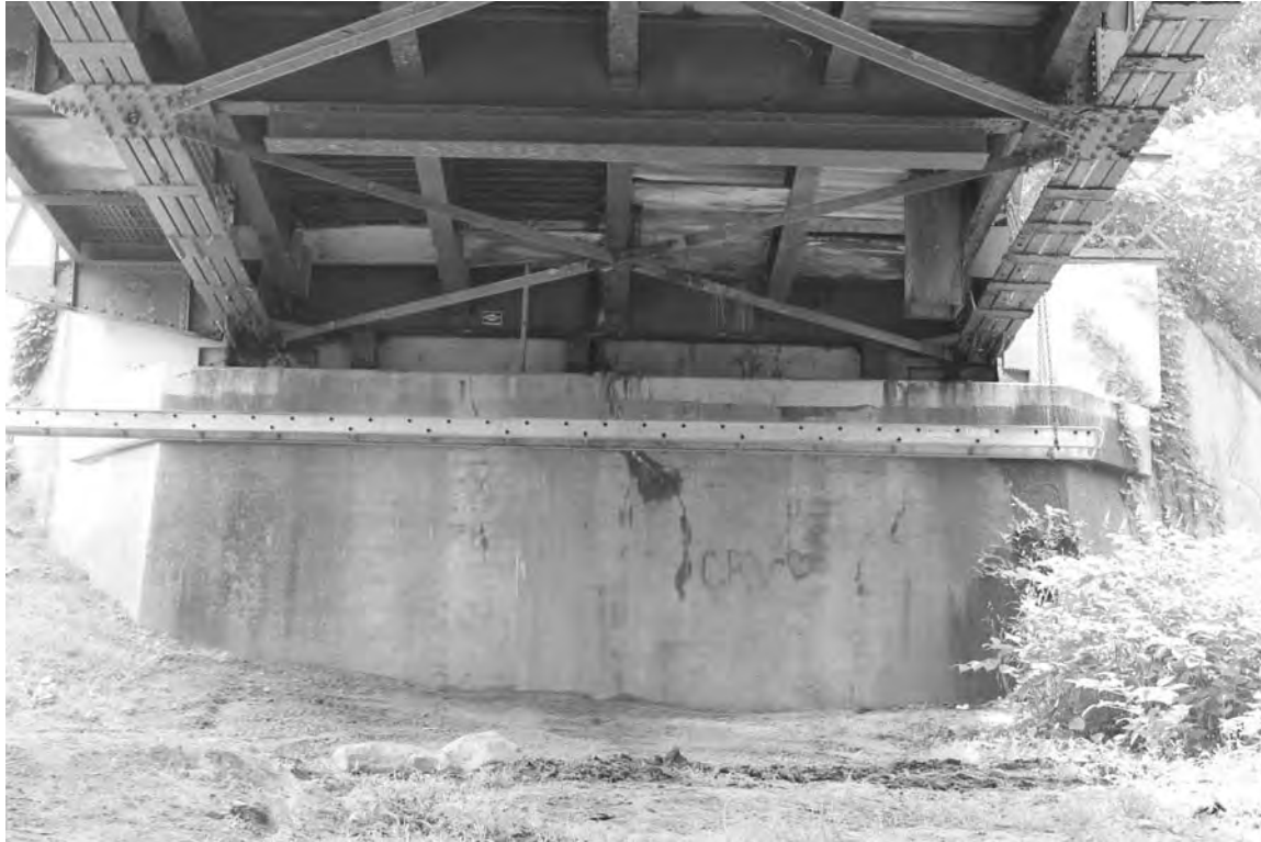
WV_Ritchie County_Cairo Bridge_0014. Southeast abutment and wingwall, facing SE.
