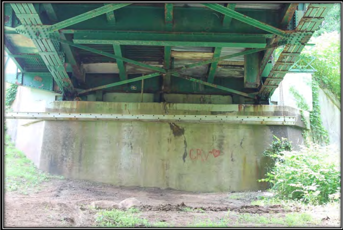
WV_Ritchie County_Cairo Bridge_0014. Southeast abutment and wingwall, facing southeast.
