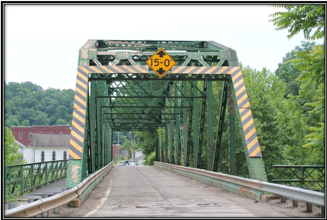
WV_Ritchie County_Cairo Bridge_0006. Through view, facing southeast.
