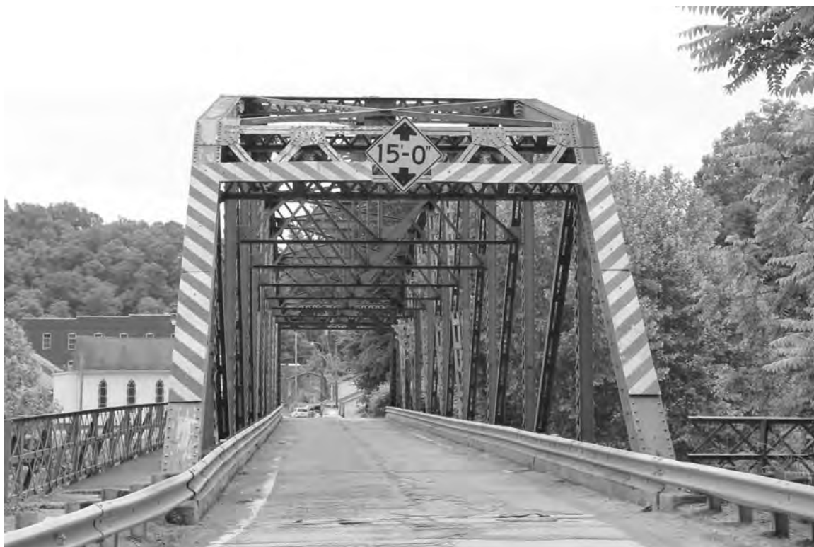
WV_Ritchie County_Cairo Bridge_0006. Through view, facing SE.
