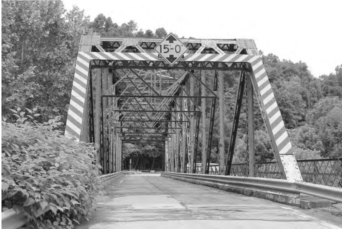
WV_Ritchie County_Cairo Bridge_0005. Through view, facing NE.
