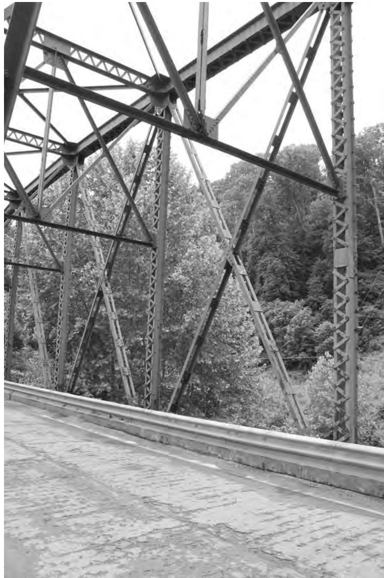
WV_Ritchie County_Cairo Bridge_0009. Detail of where the diagonal and counter-diagonal join, facing S.
