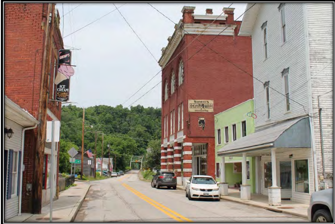
WV_Ritchie County_Cairo Bridge_0003. View of the bridge from the Cairo Historic District, facing northwest.
