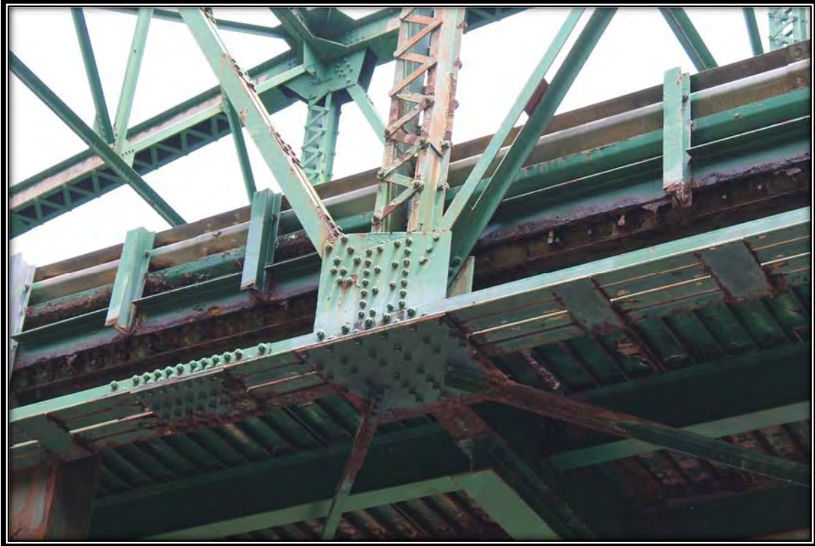
WV_Ritchie County_Cairo Bridge_0010. Lower chord panel point, facing north.
