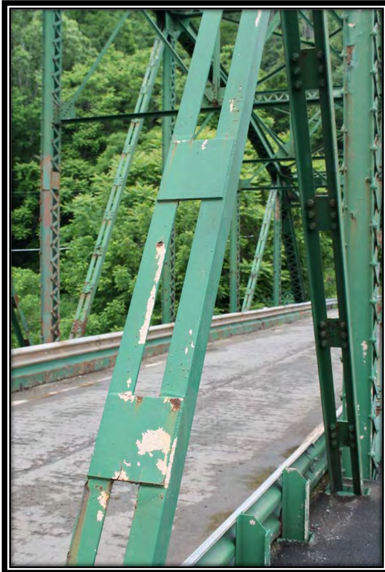
WV_Ritchie County_Cairo Bridge_0008. Detail of welded stay plates on a diagonal member, facing northwest.
