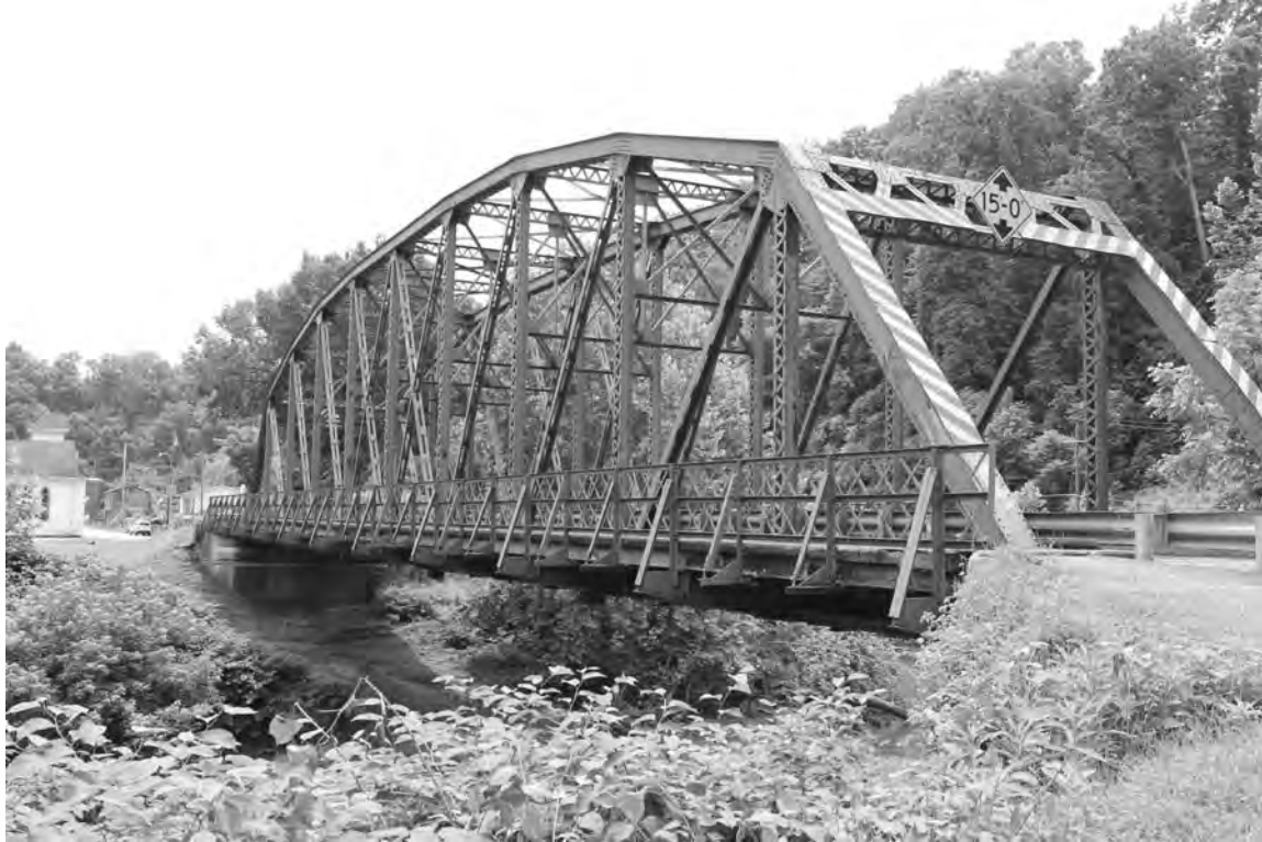
WV_Ritchie County_Cairo Bridge_0001. Elevation view, facing SE.
