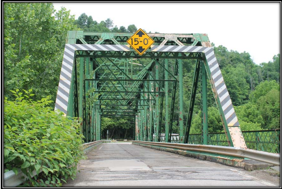
WV_Ritchie County_Cairo Bridge_0005. Through view, facing northeast.
