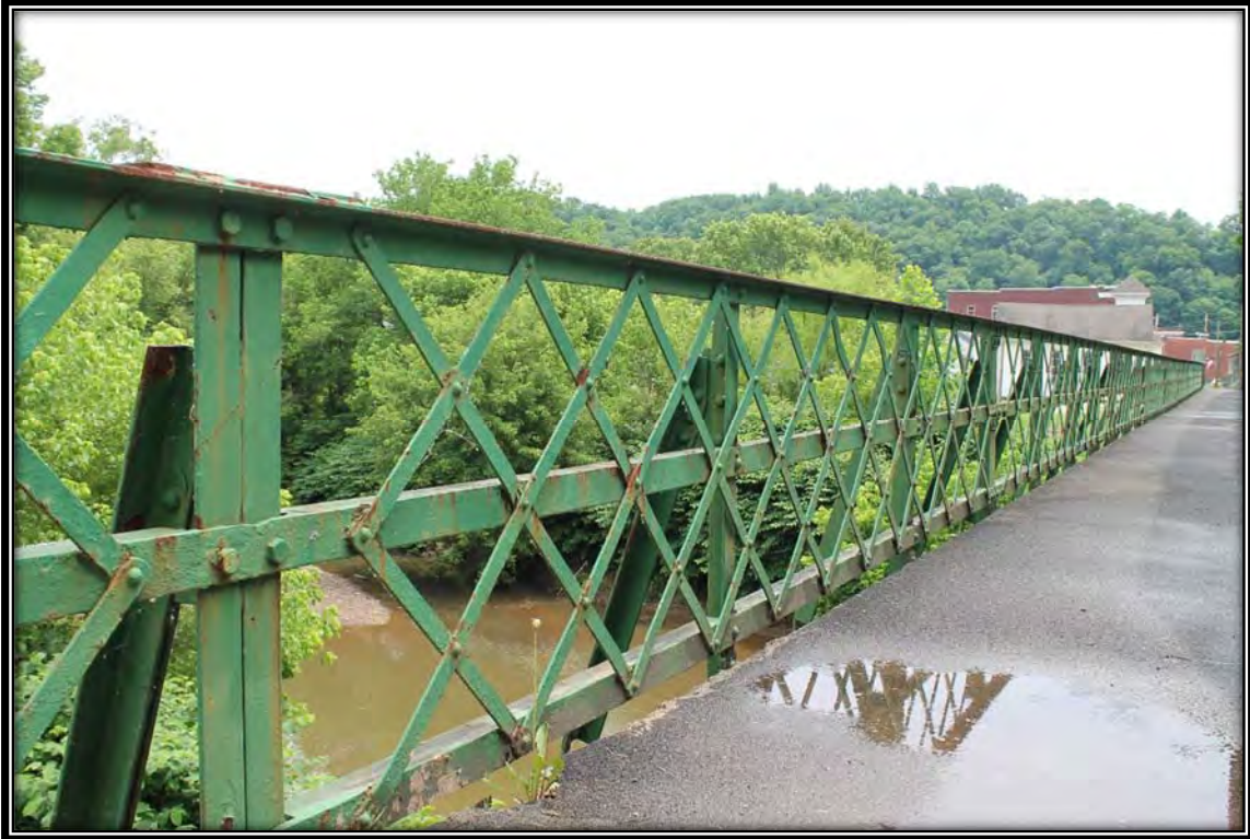
WV_Ritchie County_Cairo Bridge_0012. Detail of the bridge railing, facing southeast.
