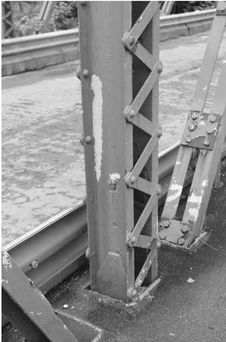
WV_Ritchie County_Cairo Bridge_0016. Representative view of a steel plate welded to a vertical, facing W.
