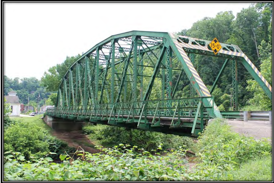
WV_Ritchie County_Cairo Bridge_0001. Elevation view, facing southeast.
