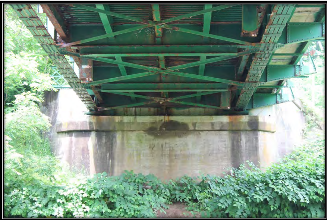
WV_Ritchie County_Cairo Bridge_0013. Northwest abutment and wingwall, facing northwest.
