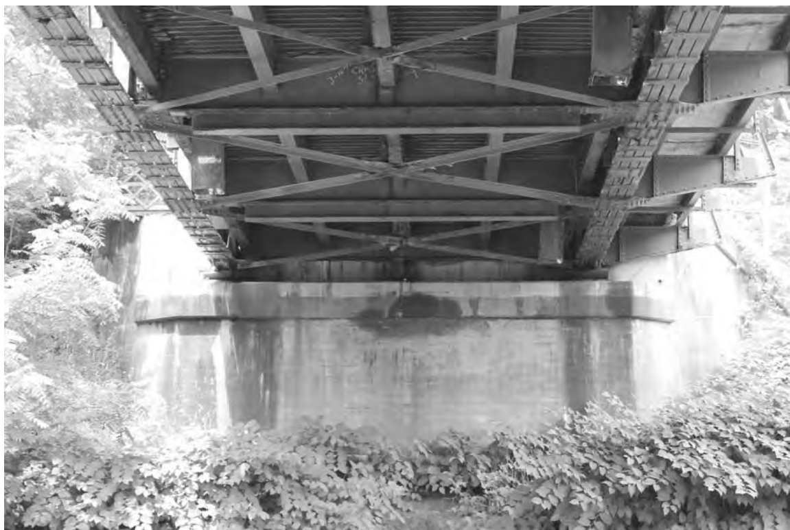
WV_Ritchie County_Cairo Bridge_0013. Northwest abutment and wingwall, facing NW.
