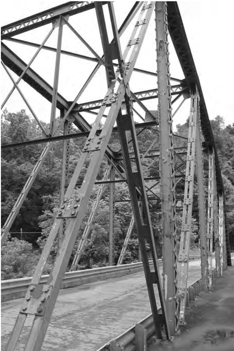
WV_Ritchie County_Cairo Bridge_0007. Detail of vertical and diagonal members, facing NW.
