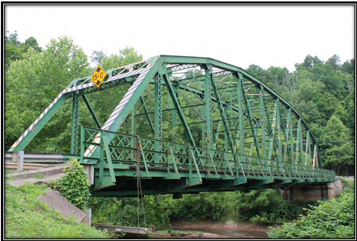
WV_Ritchie County_Cairo Bridge_0002. Elevation view, facing west.
