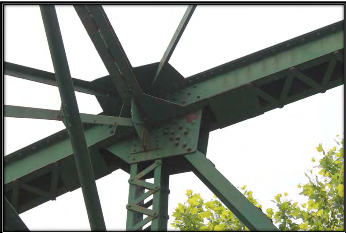
WV_Ritchie County_Cairo Bridge_0015. Upper chord panel point connection, facing south.
