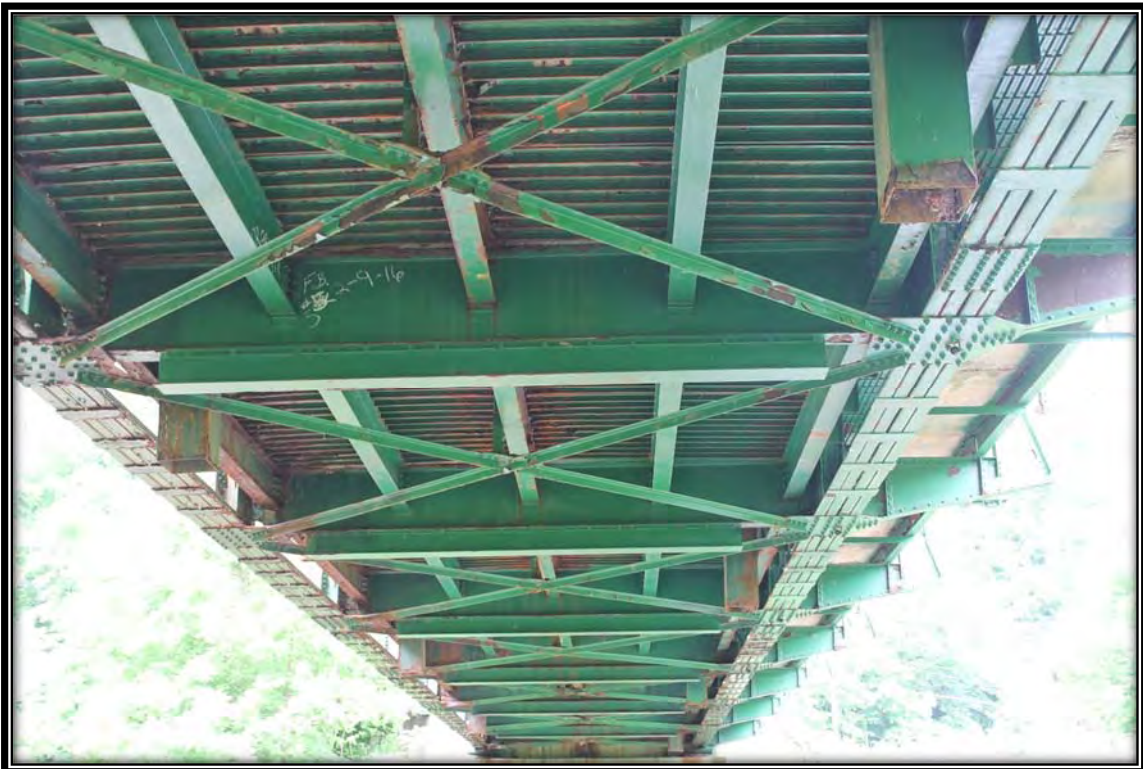
WV_Ritchie County_Cairo Bridge_0011. Underside of the bridge showing lower chords and supplemental floorbeams, facing northwest.
