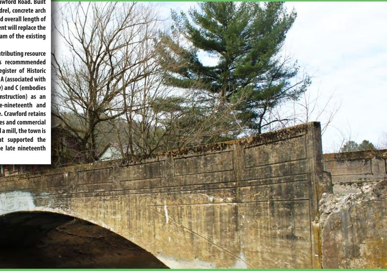
Location: Crosses the West Fork River within the community of Crawford Type: Simple Span, Solid-Spandrel, Concrete Arch Bridge Year constructed: 1923 Length: 75 feet 6 inches Contractor: Unknown
