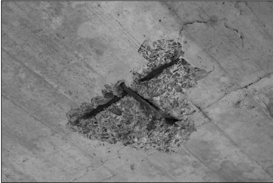
Photo 21. DETAIL OF UNDERSIDE OF ARCH SHOWING CONCRETE DETERIORATION AND EXPOSED METAL REINFORCING BARS, FACING UP (WV_Fayette County_Dunloup Creek Bridge #9_0021).
