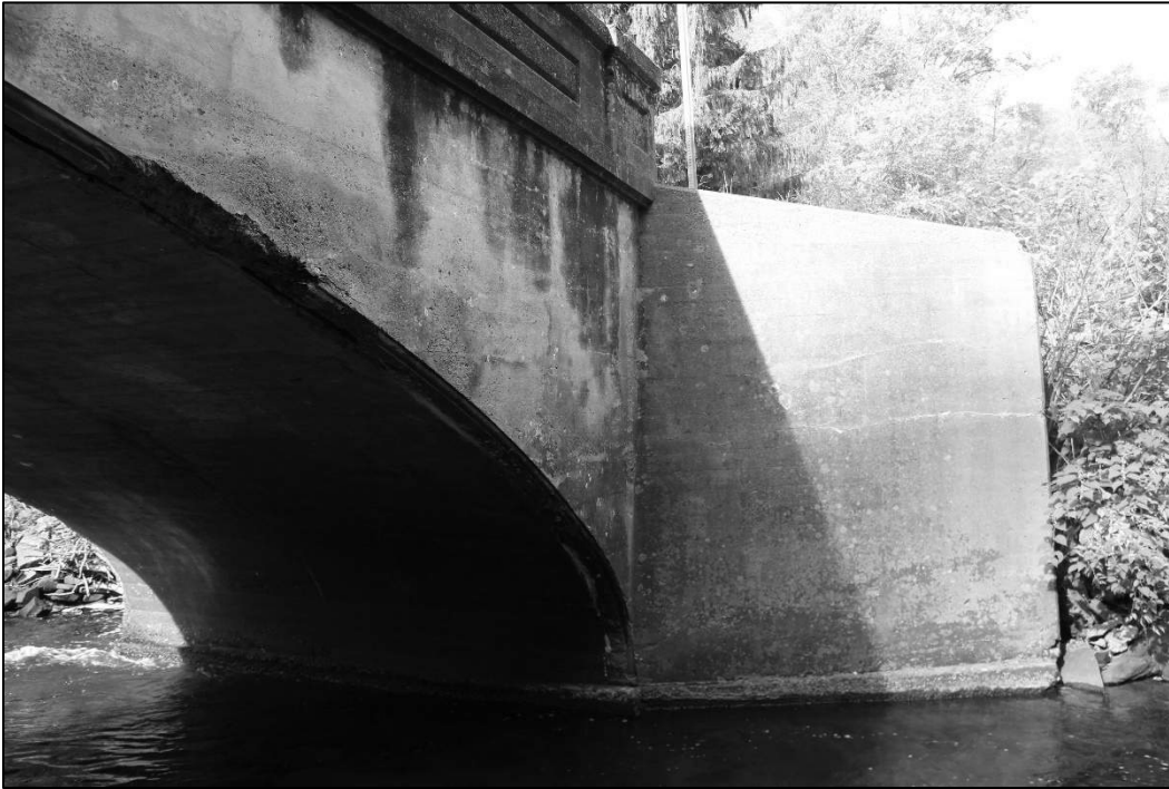
Photo 19. VIEW OF NORTHEASTERN ABUTMENT, SPANDREL WALL, ARCH INTERIOR, AND WINGWALL, FACING WEST (WV_Fayette County_Dunloup Creek Bridge #9_0019).
