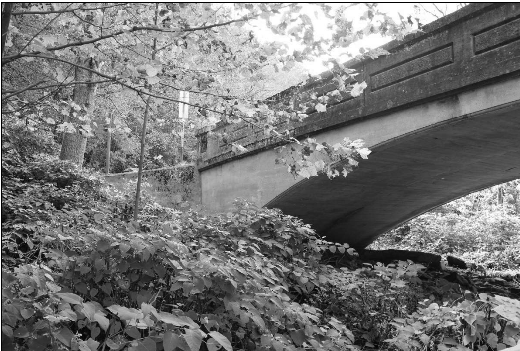
Photo 18. VIEW OF SOUTHWESTERN END OF BRIDGE, SHOWING NORTHEAST ELEVATION OF PARAPET EXTERIOR, SPANDREL WALL, AND ABUTMENT, FACING SOUTH (WV_Fayette County_Dunloup Creek Bridge #9_0018).
