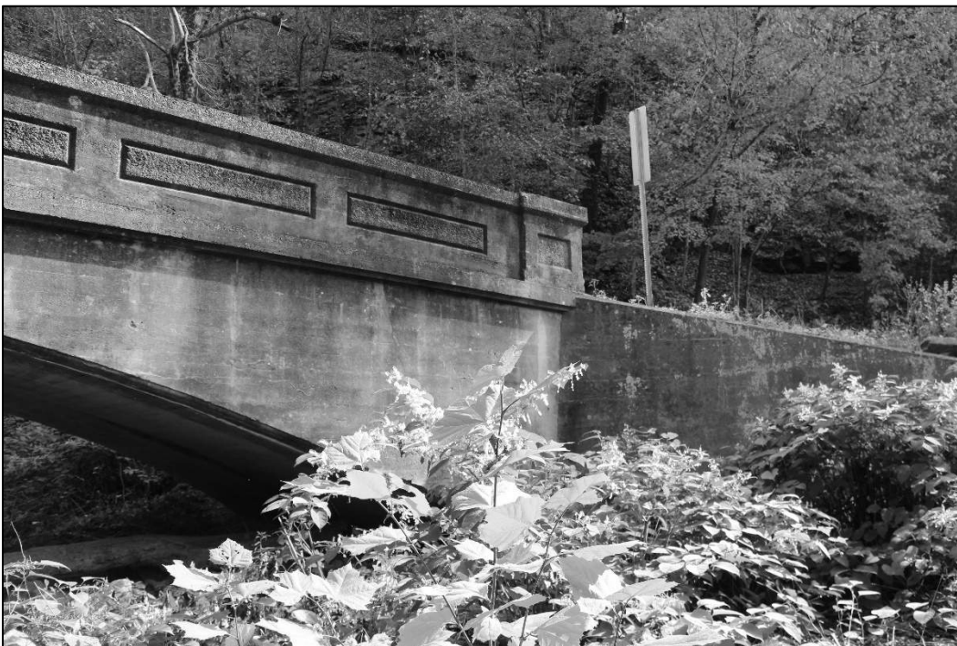
Photo 24. VIEW OF SOUTHEASTERN END OF BRIDGE SHOWING SPANDREL WALL, WINGWALL, AND PARAPET, FACING EAST (WV_Fayette County_Dunloup Creek Bridge #9_0024).
