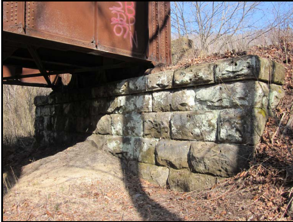
View Northwest of North Abutment (WVDOH March 18, 2014)
