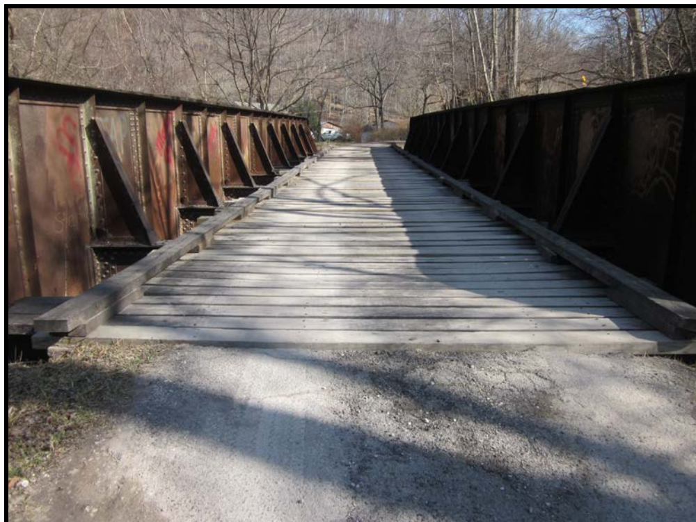
View Northeast, Deck from South End (WVDOH March 18, 2014)
