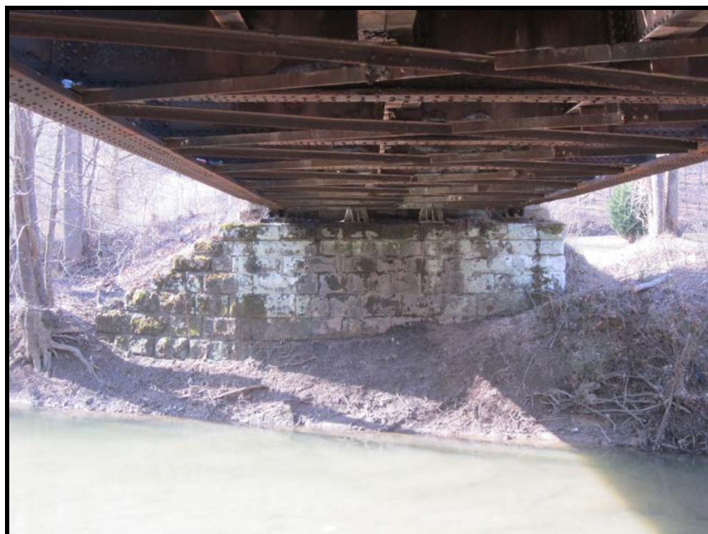
View Southwest, Toward South Abutment (WVDOH March 18, 2014)
