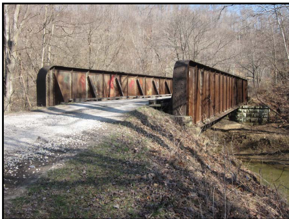
View Northwest, South Approach and East Elevation (WVDOH March 18, 2014).
