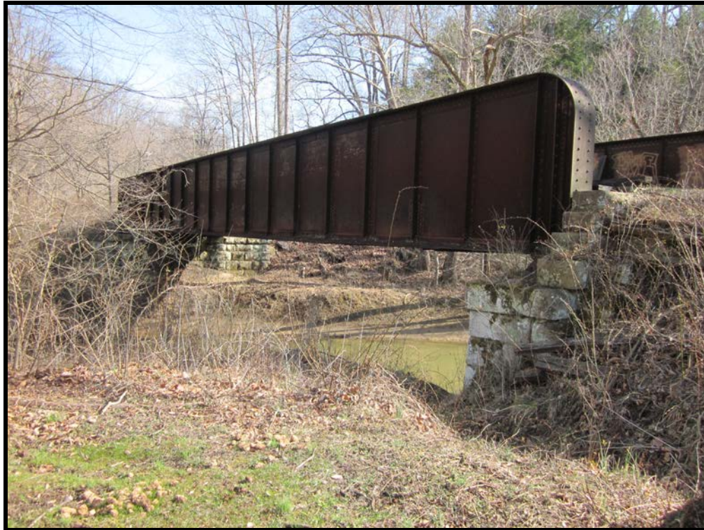
View Northeast, West Elevation (WVDOH March 18, 2014)
