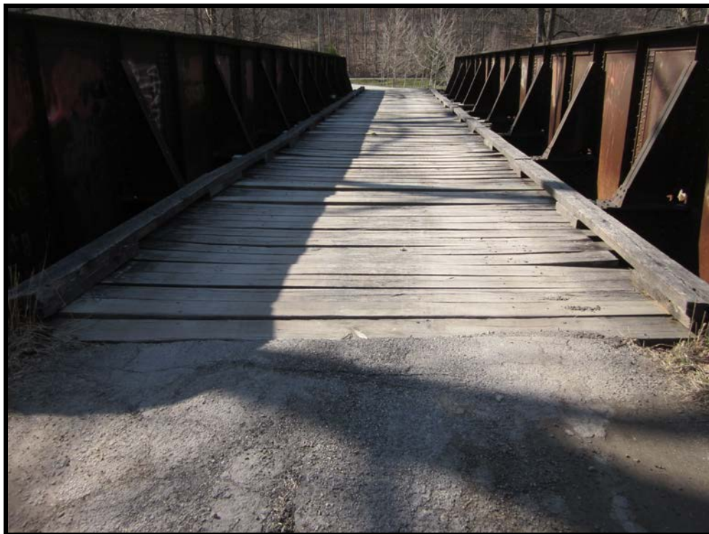
View Southwest, Deck from North End (WVDOH March 18, 2014)
