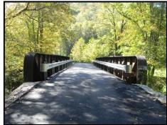
for the new stringers to rest on. Section of lateral bracing that required removal for the deck repairs were replaced as necessary. Guardrails were affixed to the inward-facing sides of the girders.
