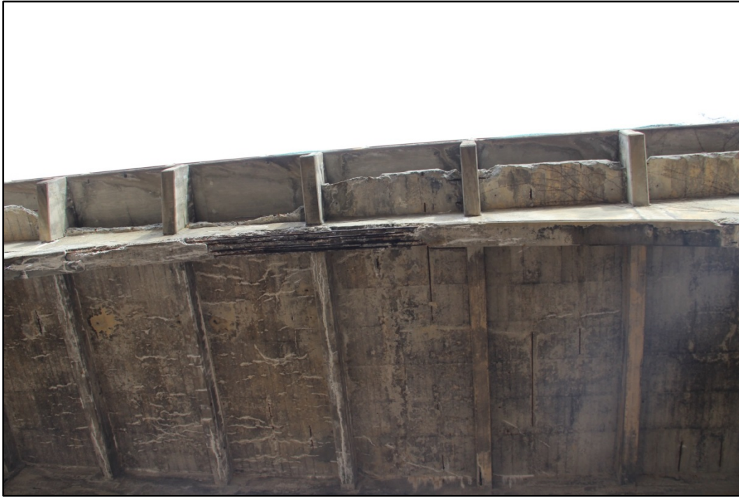
Photo 13: Detail of underside of span 3, facing up. Note exposed reinforcing bars on girder; remnants of original sidewalk are visible in right half of photo. WV_Marion County_Fourth Street Bridge-0013
