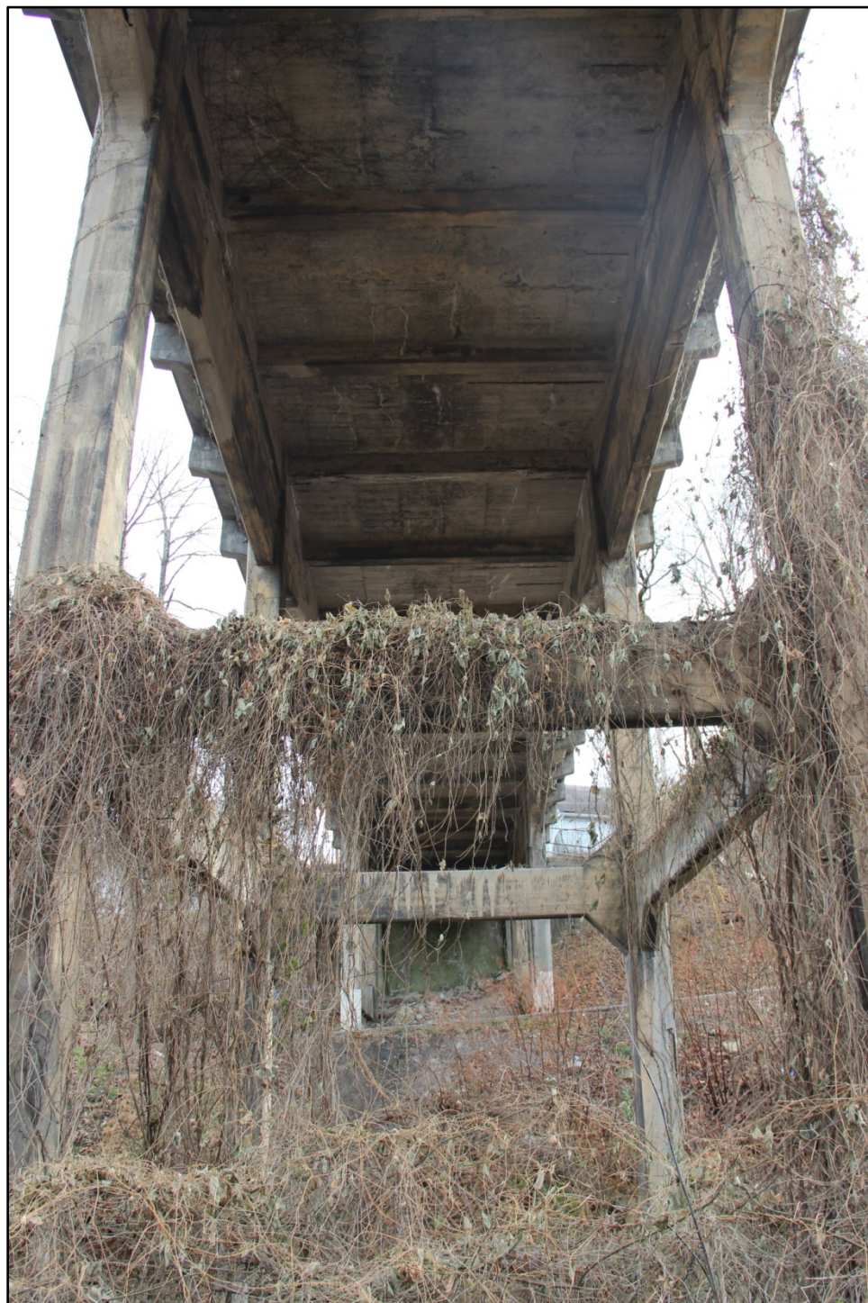
Photo 11: View of underside of bridge deck and bent details at span 4, facing SE. WV_Marion County_Fourth Street Bridge-0011
