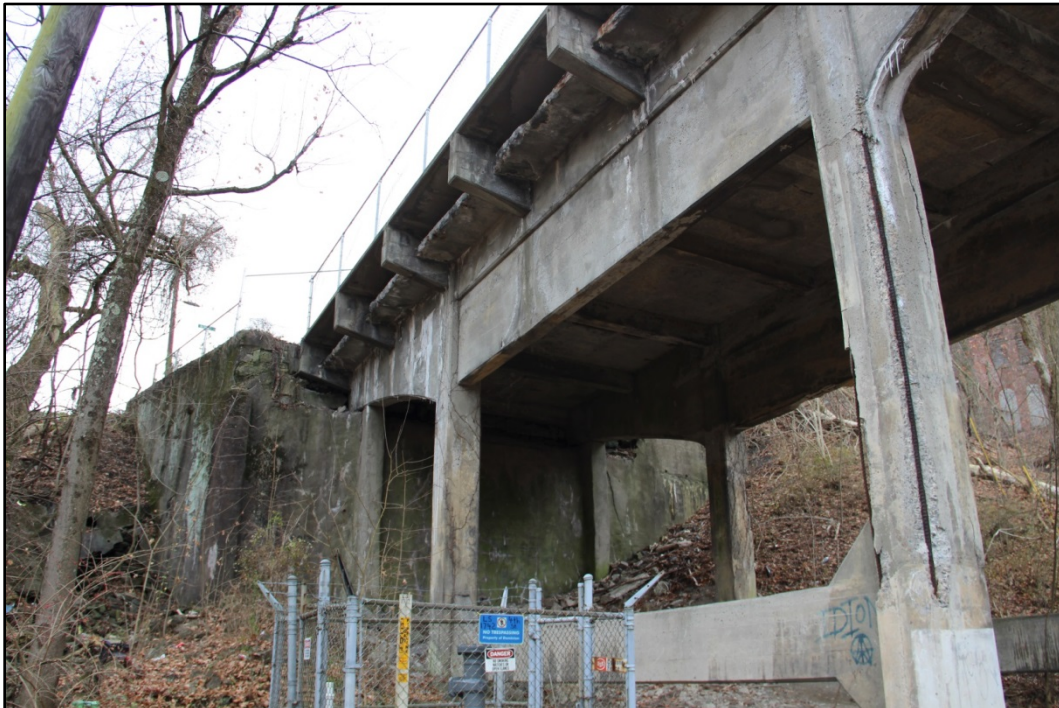
Photo 20: NE side of bridge, spans 6-7, facing S. WV_Marion County_Fourth Street Bridge-0020
