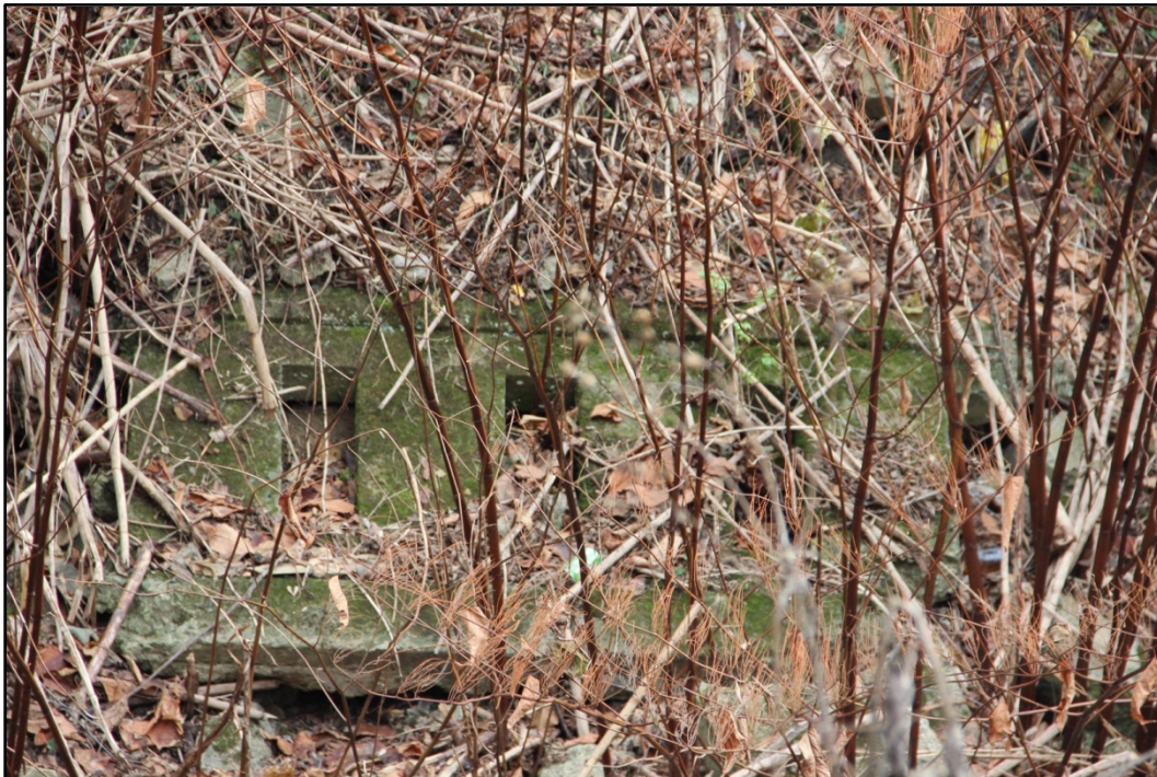
Photo 14: Section of original concrete railing that has fallen off bridge. WV_Marion County_Fourth Street Bridge-0014
