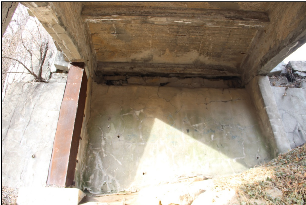
Photo 8: SE side of abutment at NW end of bridge, facing NW. Note concrete encasement. WV_Marion County_Fourth Street Bridge-0008
