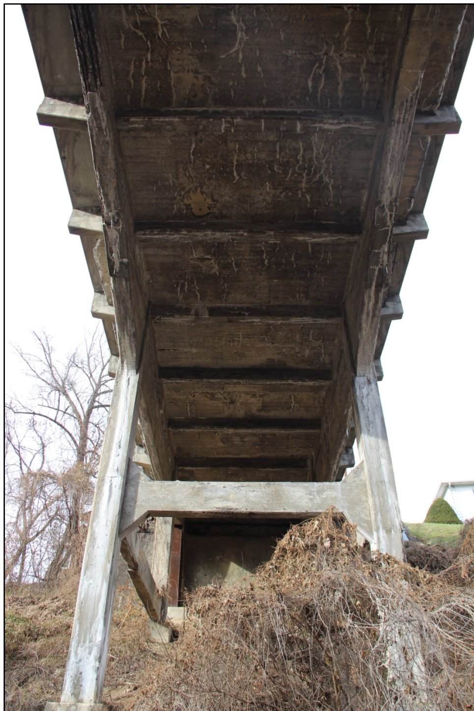
Photo 10: View of underside of bridge deck and bent details, span 3, facing NW. WV_Marion County_Fourth Street Bridge-0010
