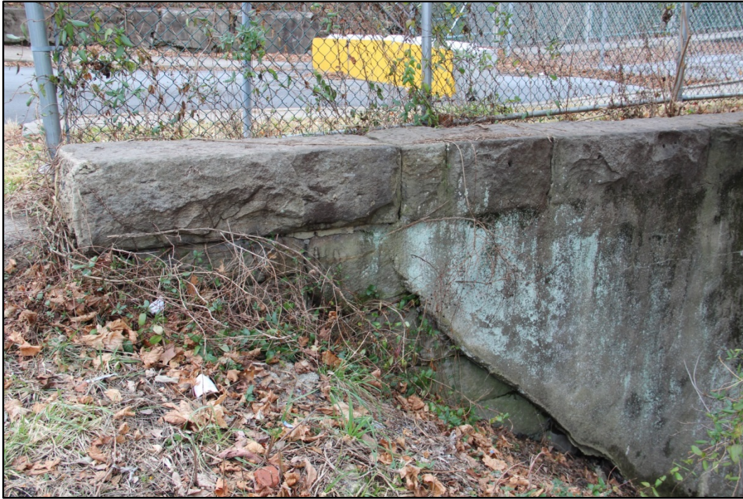
Photo 23: Detail of stone coping on NE side of SE abutment, facing W. WV_Marion County_Fourth Street Bridge-0023
