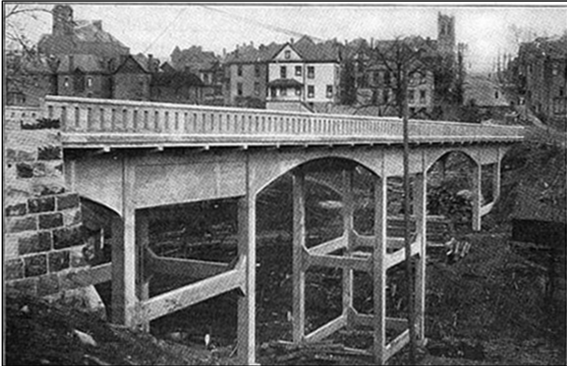
Photo 26: Early view of Fourth Street Bridge, showing SW side, facing E. Source: Engineering News , Vol. 73 No. 16, page 791 (April 22, 1915).
