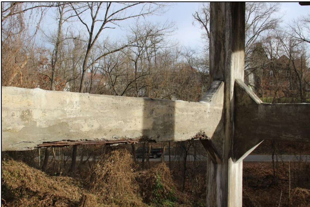
Photo 16: Detail of horizontal braces on span 3 column bents, facing E. WV_Marion County_Fourth Street Bridge-0016
