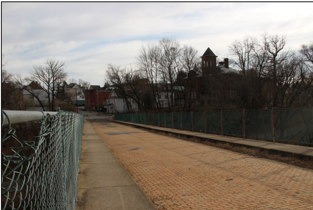
Photo 6: Bridge deck showing sidewalks and fence, which are modern replacements, NW end of bridge, facing S. Note that original sidewalk was at same level as roadway. WV_Marion County_Fourth Street Bridge-0006
