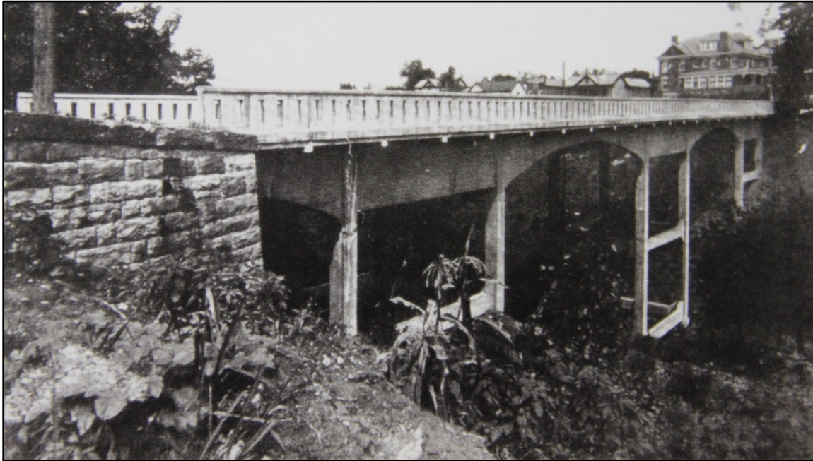
Photo 28: 1921 view of Fourth Street Bridge, showing NE side, facing W. Source: Marion County Historical Society.
