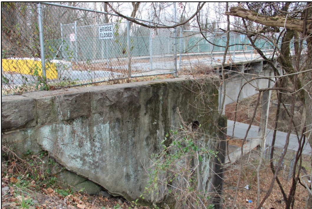
Photo 24: NE side of SE abutment, showing concrete veneer, facing W. WV_Marion County_Fourth Street Bridge-0024
