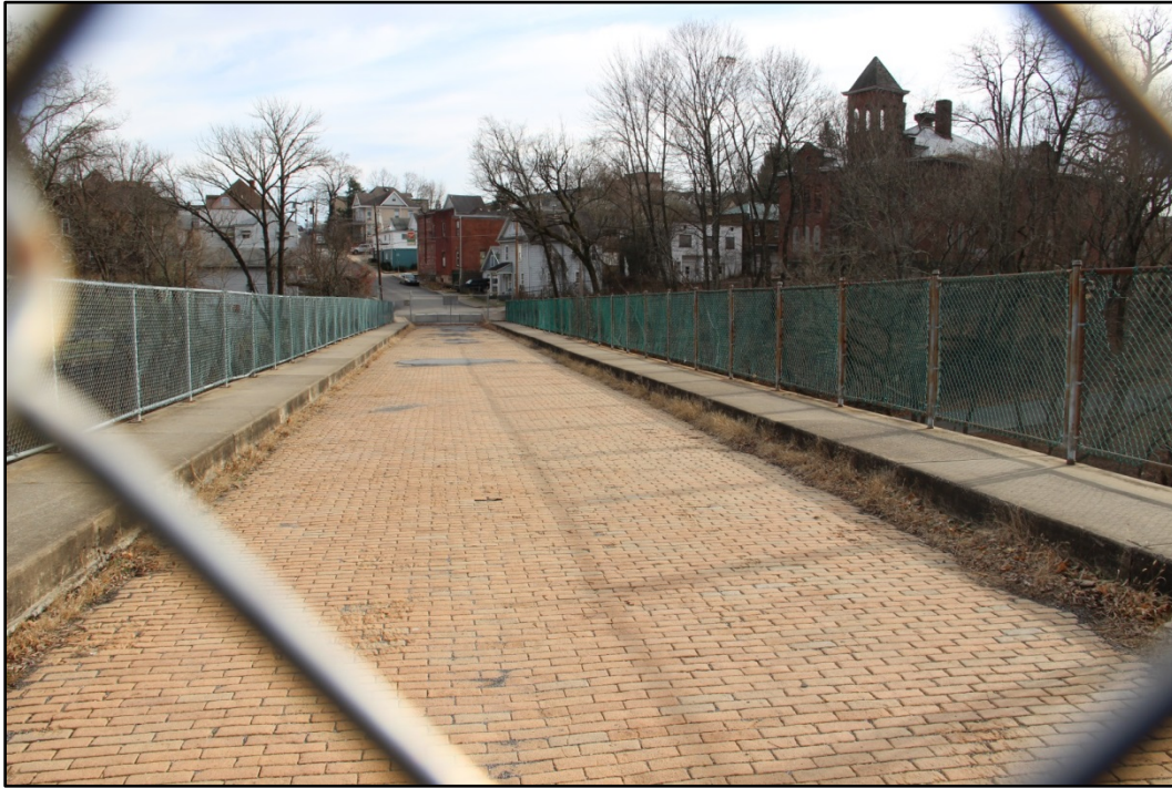
Photo 5: Bridge deck showing brick pavement, NW end, facing SE. WV_Marion County_Fourth Street Bridge-0005
