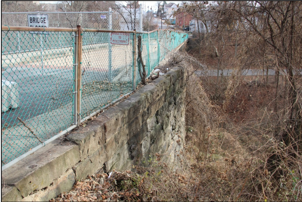
Photo 7: SW side of abutment at NW end of bridge, facing SE. WV_Marion County_Fourth Street Bridge-0007
