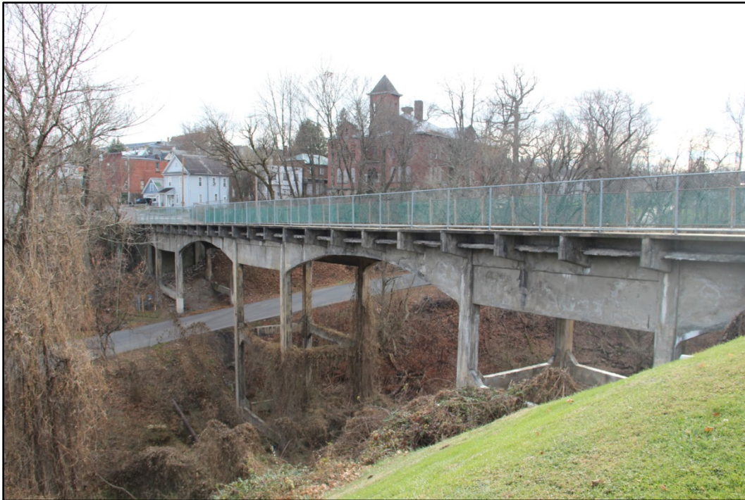
Photo 1: NE side of bridge, facing S.
