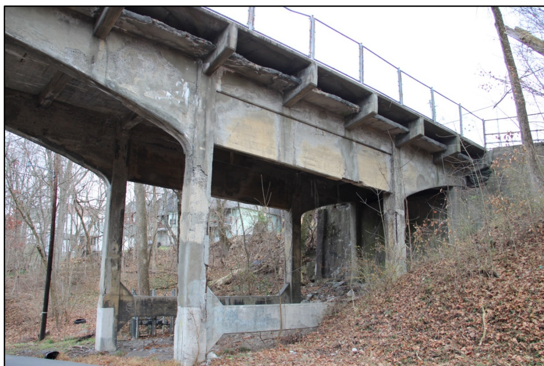
Photo 18: SW side of bridge, spans 5-7, facing E. WV_Marion County_Fourth Street Bridge-0018
