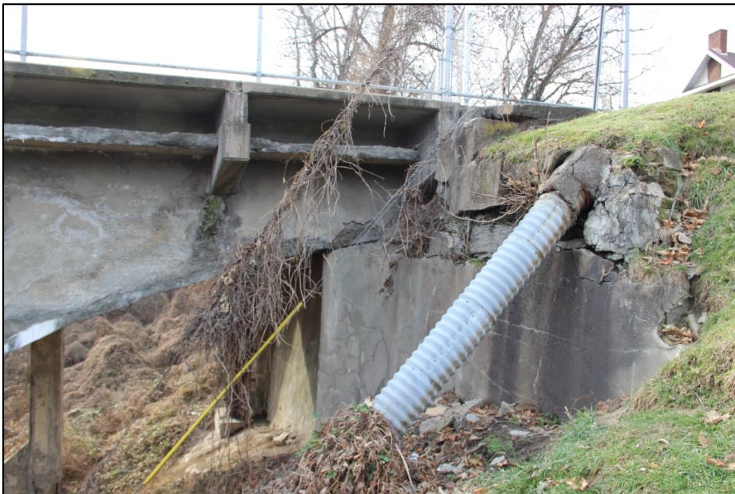
Photo 4: Detail of span 1 and NW abutment, NE side of bridge, facing NW. WV_Marion County_Fourth Street Bridge-0004
