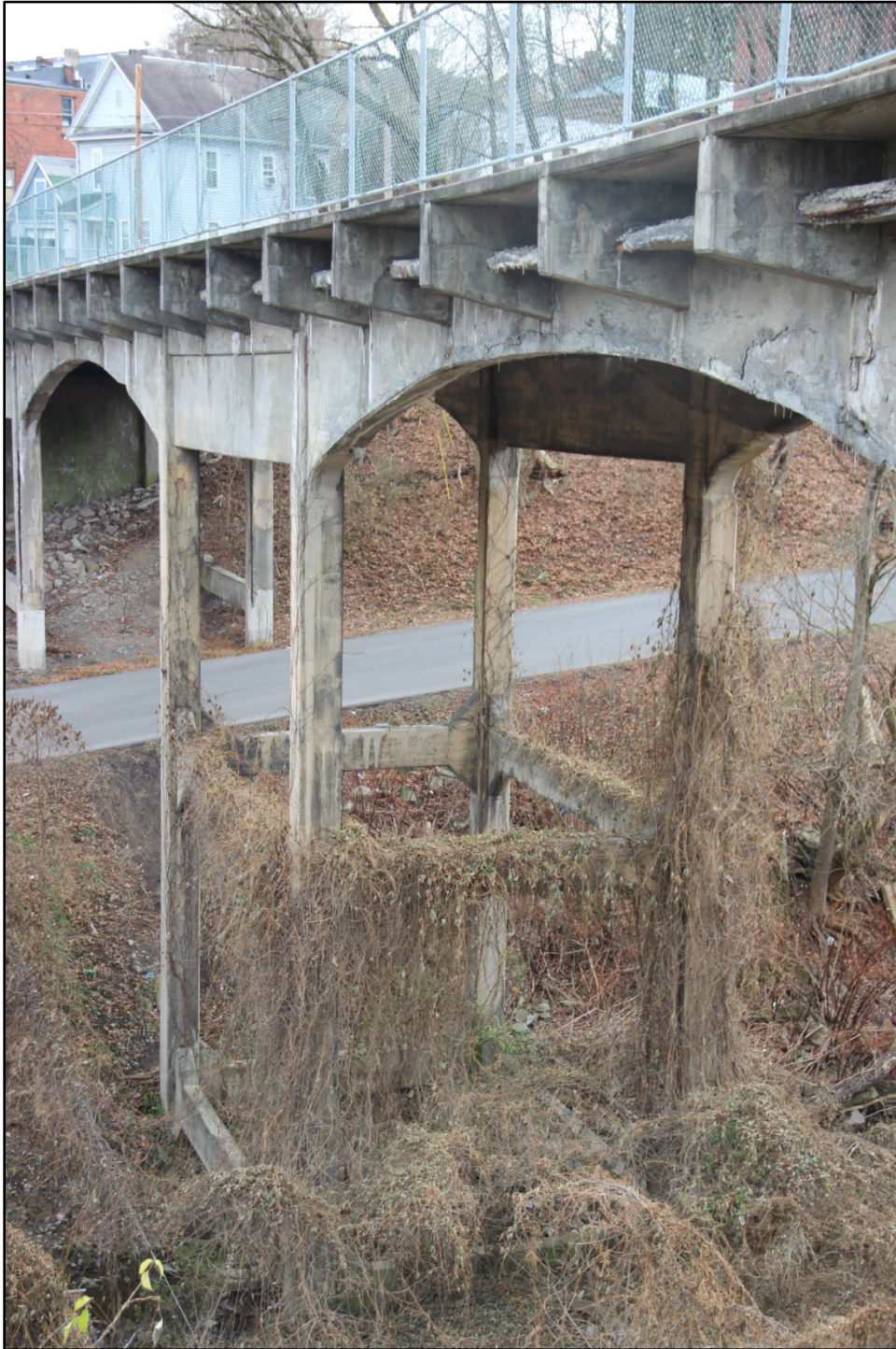
Photo 2: Detail of span 3-5, NE side of bridge, facing S. WV_Marion County_Fourth Street Bridge-0002
