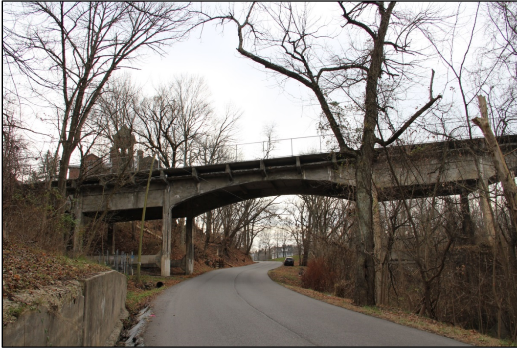
Photo 21: Overview of NE side of bridge from Benoni Avenue, showing spans 4-6, facing SW. WV_Marion County_Fourth Street Bridge-0021
