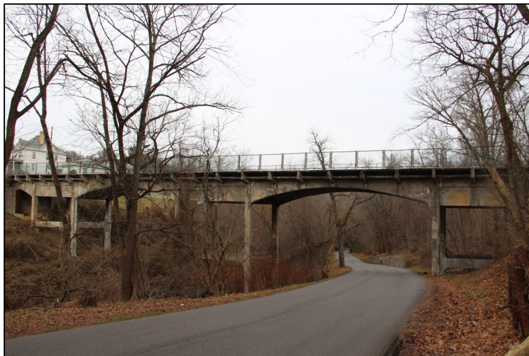
Photo 17: Overview of SW side of bridge from Benoni Avenue, facing NE. WV_Marion County_Fourth Street Bridge-0017
