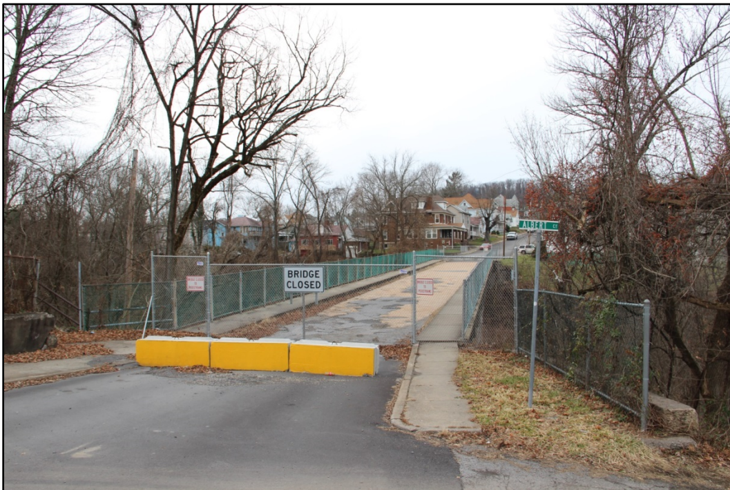
Photo 22: Overview of SW end of bridge from Fourth Street, facing NW. WV_Marion County_Fourth Street Bridge-0022
