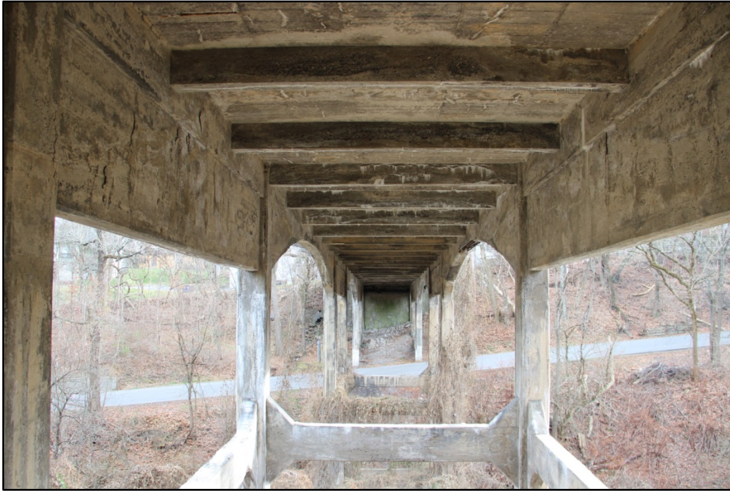
Photo 9: View of underside of bridge deck and column and beam details at span 2, NW end, facing SE. WV_Marion County_Fourth Street Bridge-0009
