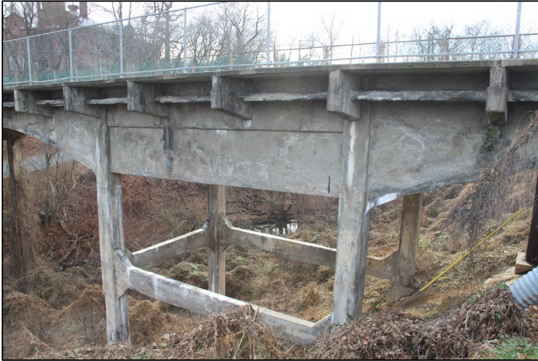
Photo 3: Detail of span 2, NE side of bridge, facing S. WV_Marion County_Fourth Street Bridge-0003
