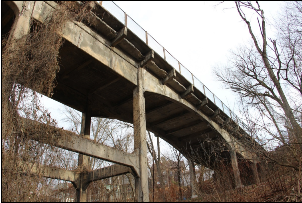
Photo 15: Overview of SW side of bridge, spans 4-7, facing E. WV_Marion County_Fourth Street Bridge-0015
