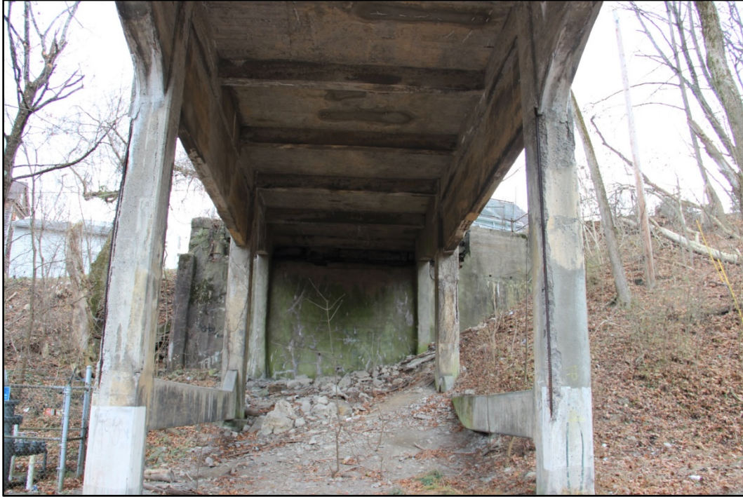
Photo 19: Underside of span 7, showing concrete column bents, girders, and deck, facing S. WV_Marion County_Fourth Street Bridge-0019
