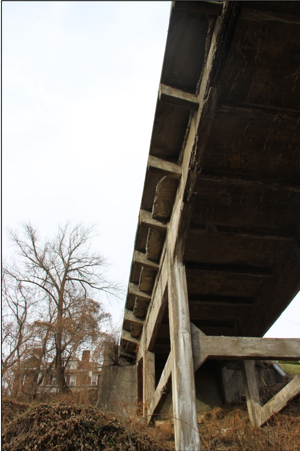
Photo 12: View of sidewalk brackets and concrete girders in spans 1-3, facing NW. WV_Marion County_Fourth Street Bridge-0012
