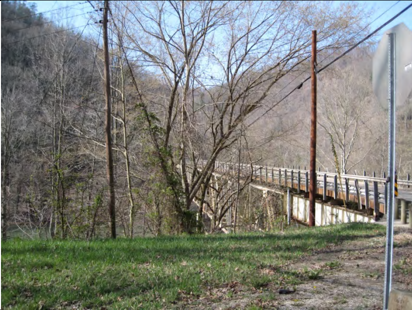
17. Upstream side of bridge from north bank.
