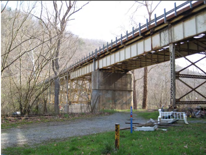
3. Girder spans on south end of bridge.
