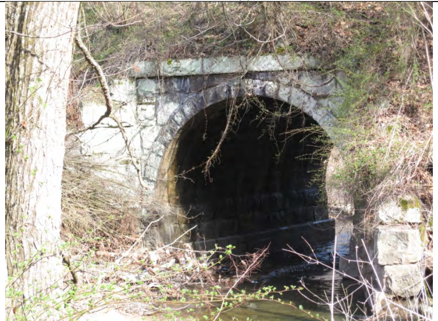
20. Railroad culvert for Middle Creek on south bank.
