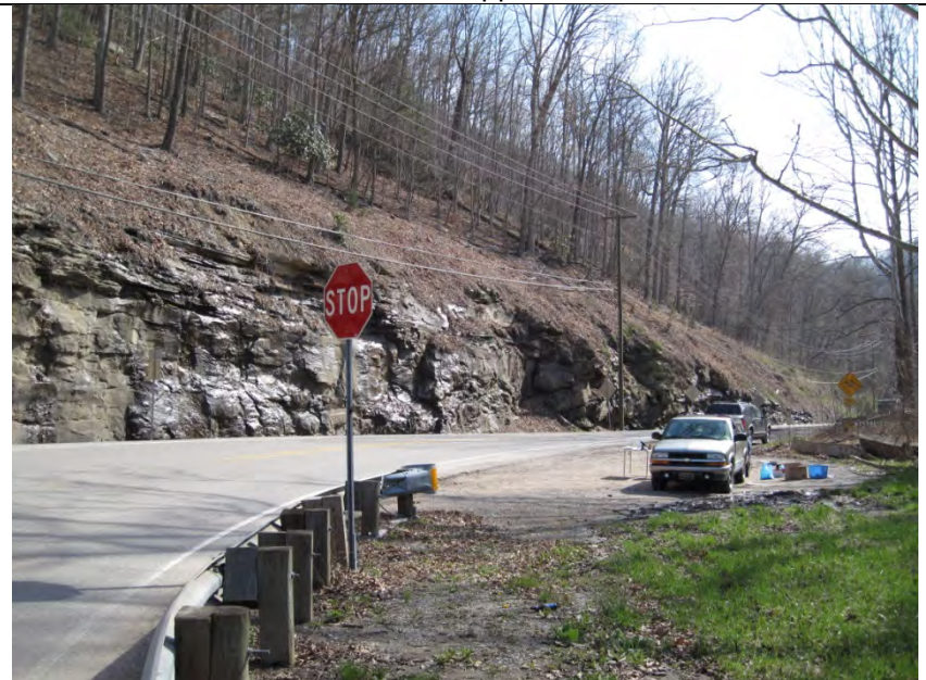
16. Project environs at north end of bridge looking east.
