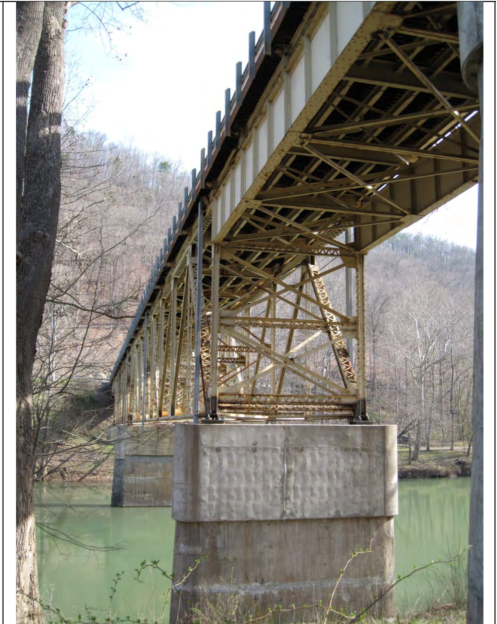
10. Downstream side of bridge from south bank.
