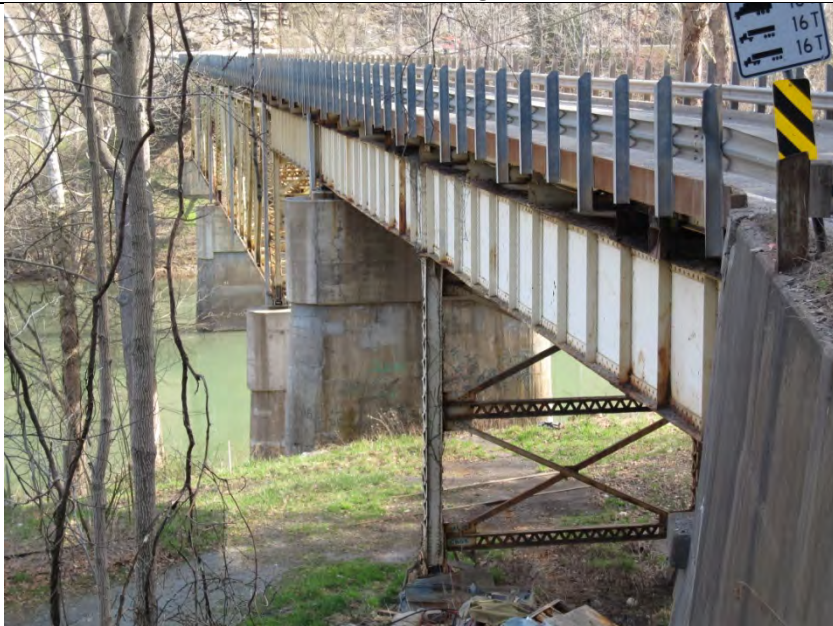
19. Downstream side of bridge from south approach.
