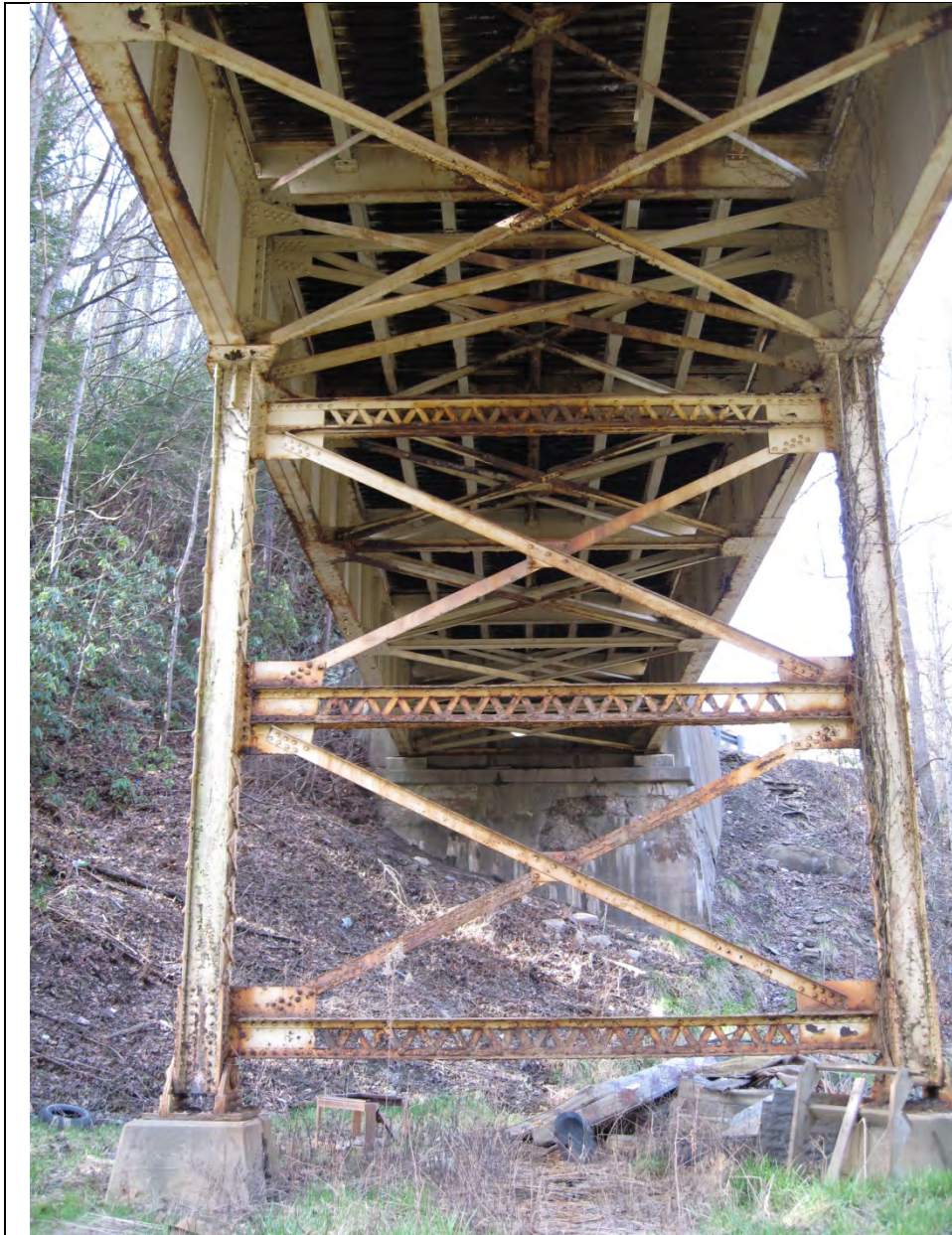
9. Girder spans and bent at south end of bridge.
