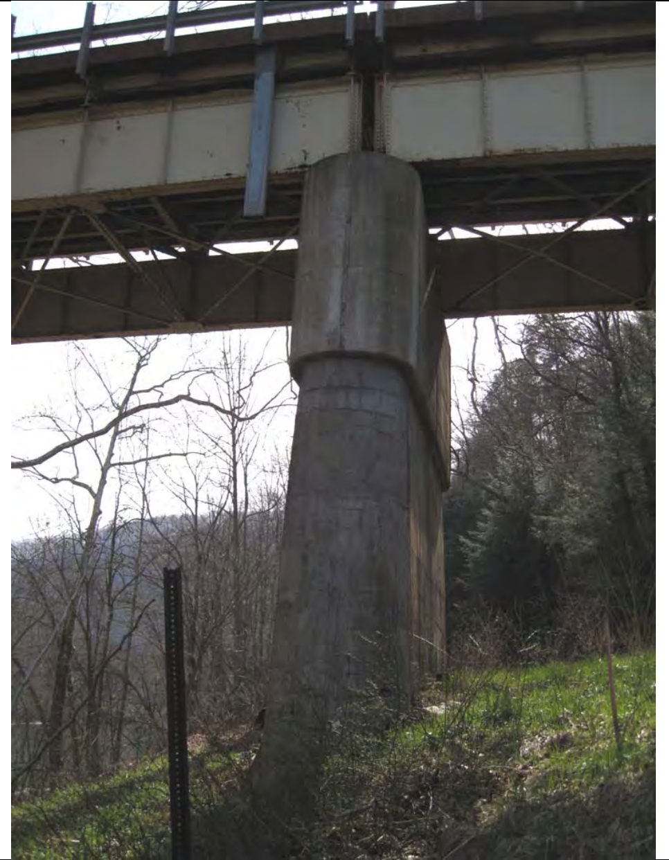
12. Pier at girder spans, south bank.
