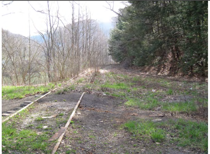
4. Rail lines under bridge on south bank looking east.
