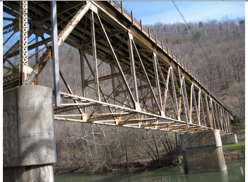
8. View of upstream side of deck truss from south bank.
