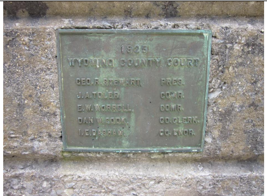
12. Plaque on West End of South (Downstream) Railing. View Southeast
