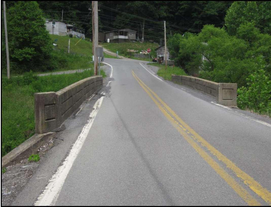
Milam Arch Bridge – East Approach. View NW (WVDOH 6-12-2017).
