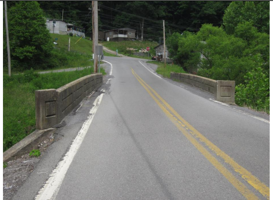
10. East Approach. View Southwest.
