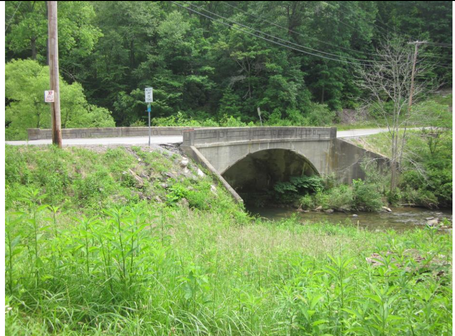
4. South (Downstream) Elevation. View Northeast
