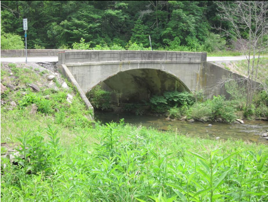
3. South (Downstream) Elevation. View Northeast
