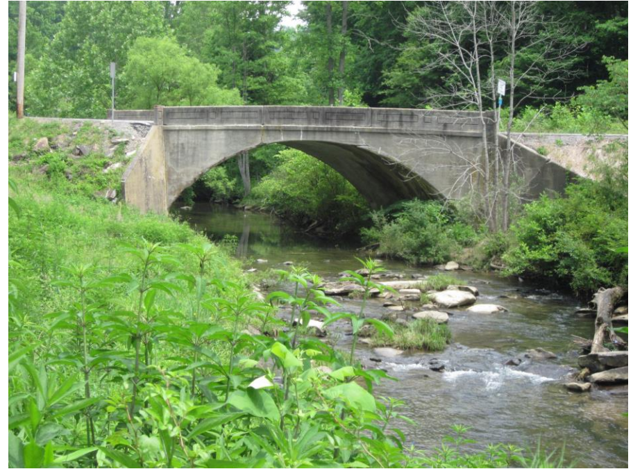
2. West (Downstream) South (Downstream) Elevation. View Northeast
