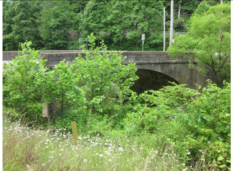
6. North (Upstream) Elevation. View Southeast
