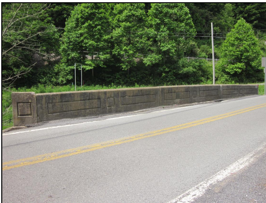
Milam Arch Bridge – South Parapet Railing. View SW (WVDOH 6-12-2017).
