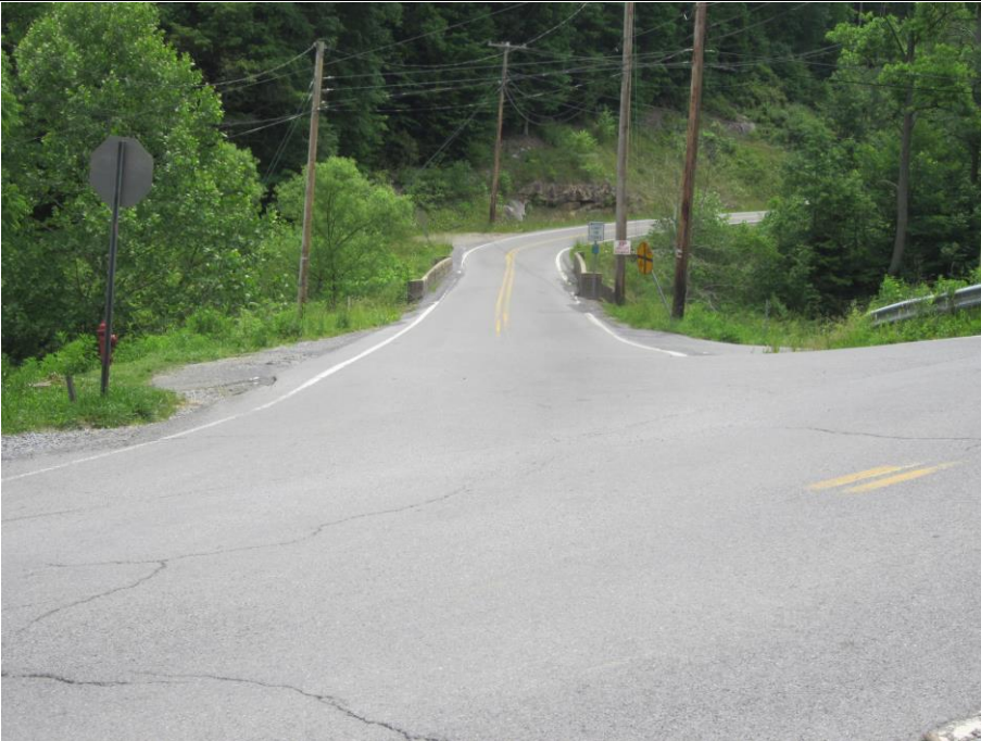
7. West Approach. View Northeast
