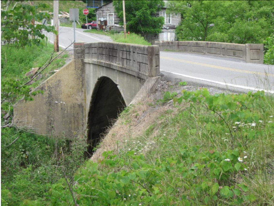
5. South (Downstream) Elevation & East Approach. View Southwest
