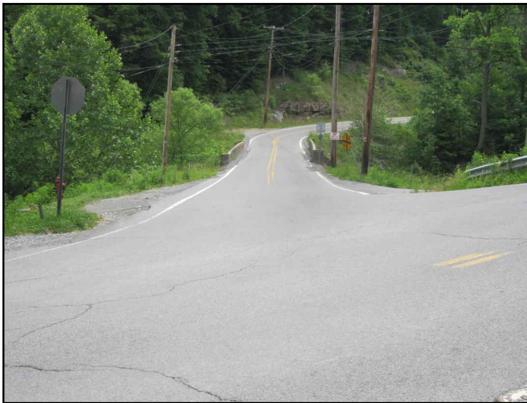
Milam Arch Bridge – West Approach, taken from County Rt 1. View SE (WVDOH 6-12-2017).
