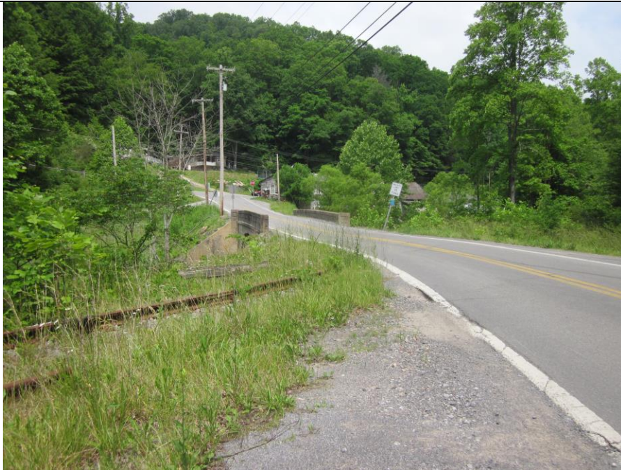
9. East Approach. View Southwest
