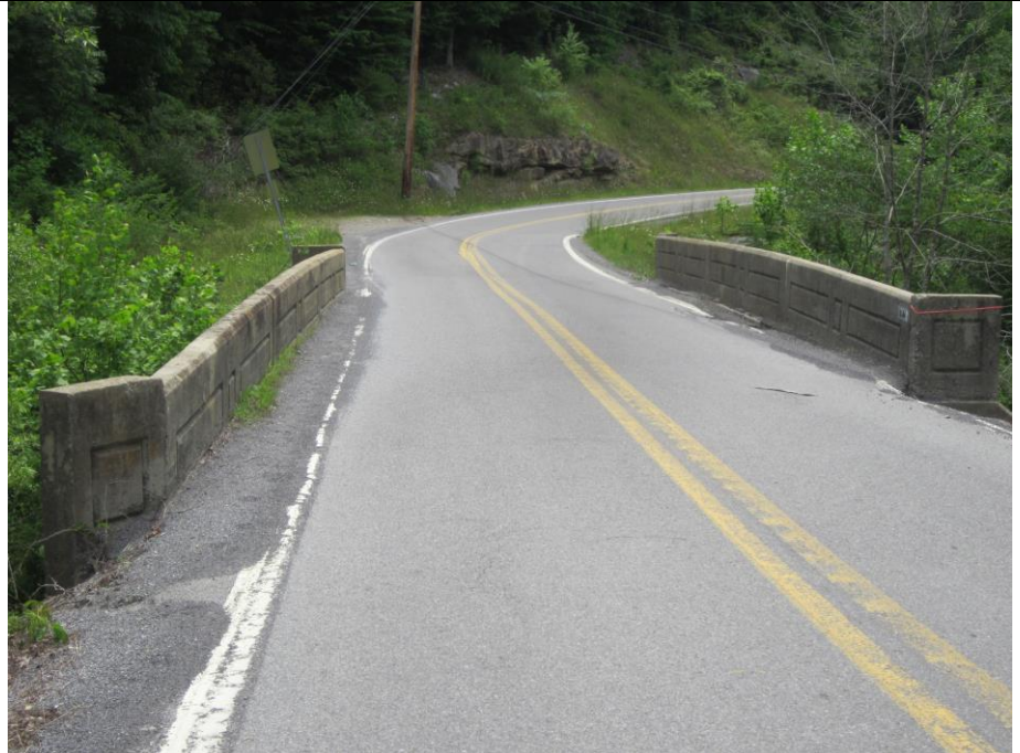
8. West Approach. View Northeast
