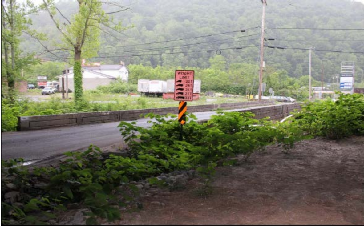
Photograph 1. Mt. Gay Deck Arch Bridge, LG-0758/LG-0764, Facing Northwest
