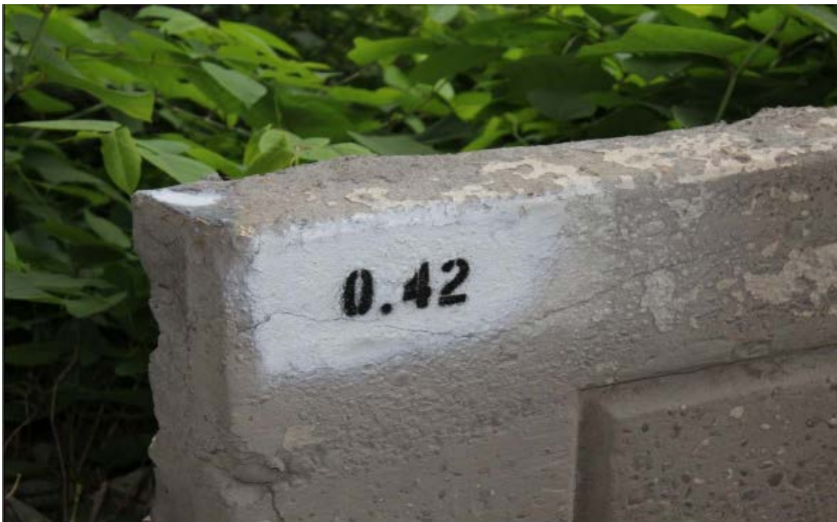
Photograph 10. Mt. Gay Deck Arch Bridge, LG-0758/LG-0764, Mile Marker Facing West
