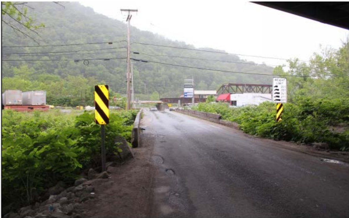
Photograph 2. Mt. Gay Deck Arch Bridge, LG-0758/LG-0764, Facing North
