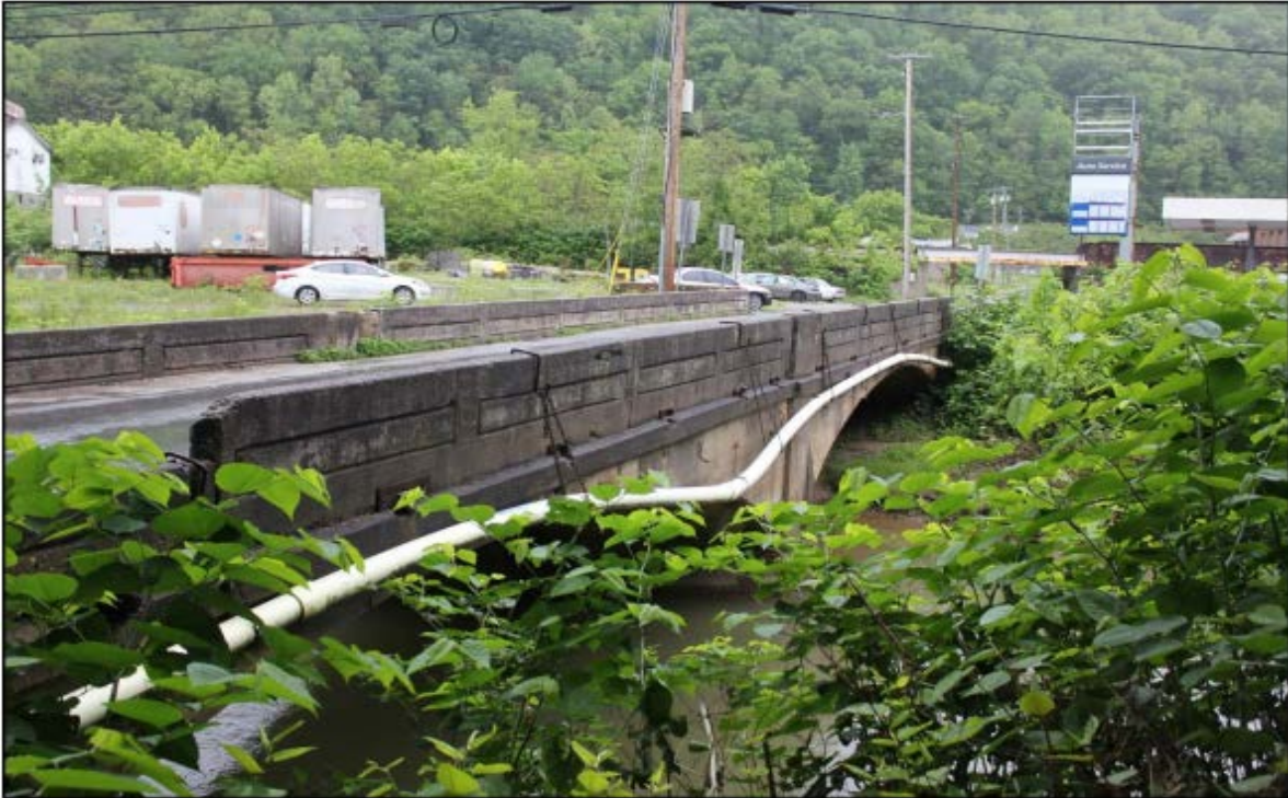
Photograph 5. Mt. Gay Deck Arch Bridge, LG-0758/LG-0764, Former Sidewalk Facing Northwest
