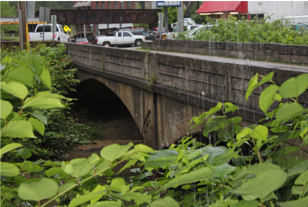
Photograph 8. Mt. Gay Deck Arch Bridge, LG-0758/OG-0764, View Spandrel Wall and Pier, Facing Northeast
