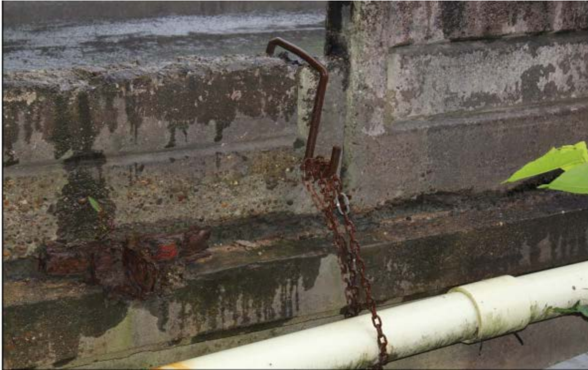
Photograph 9. Mt. Gay Deck Arch Bridge, LG-0758/LG-0764, Sidewalk Support and Hook Facing West
