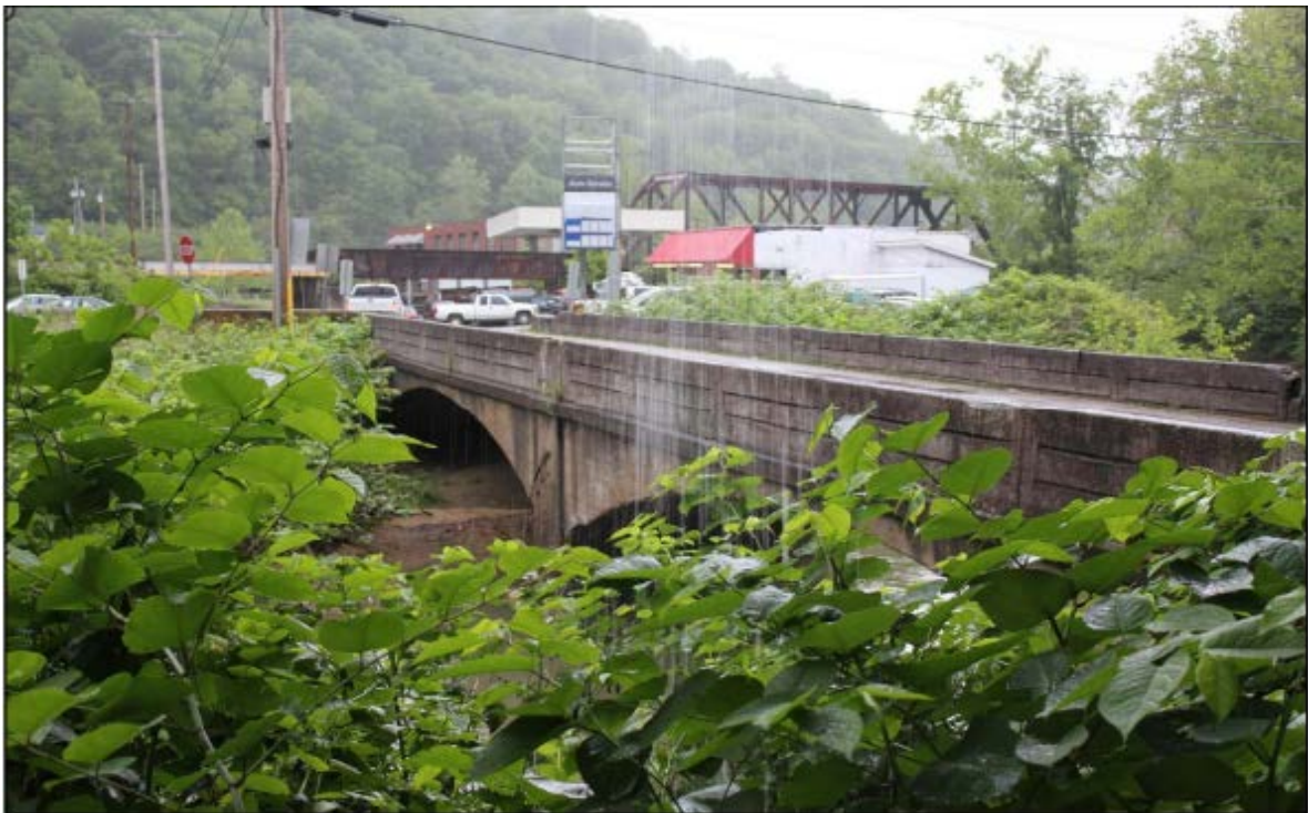
Photograph 4. Mt. Gay Deck Arch Bridge, LG-0758/LG-0764, Facing Northeast
