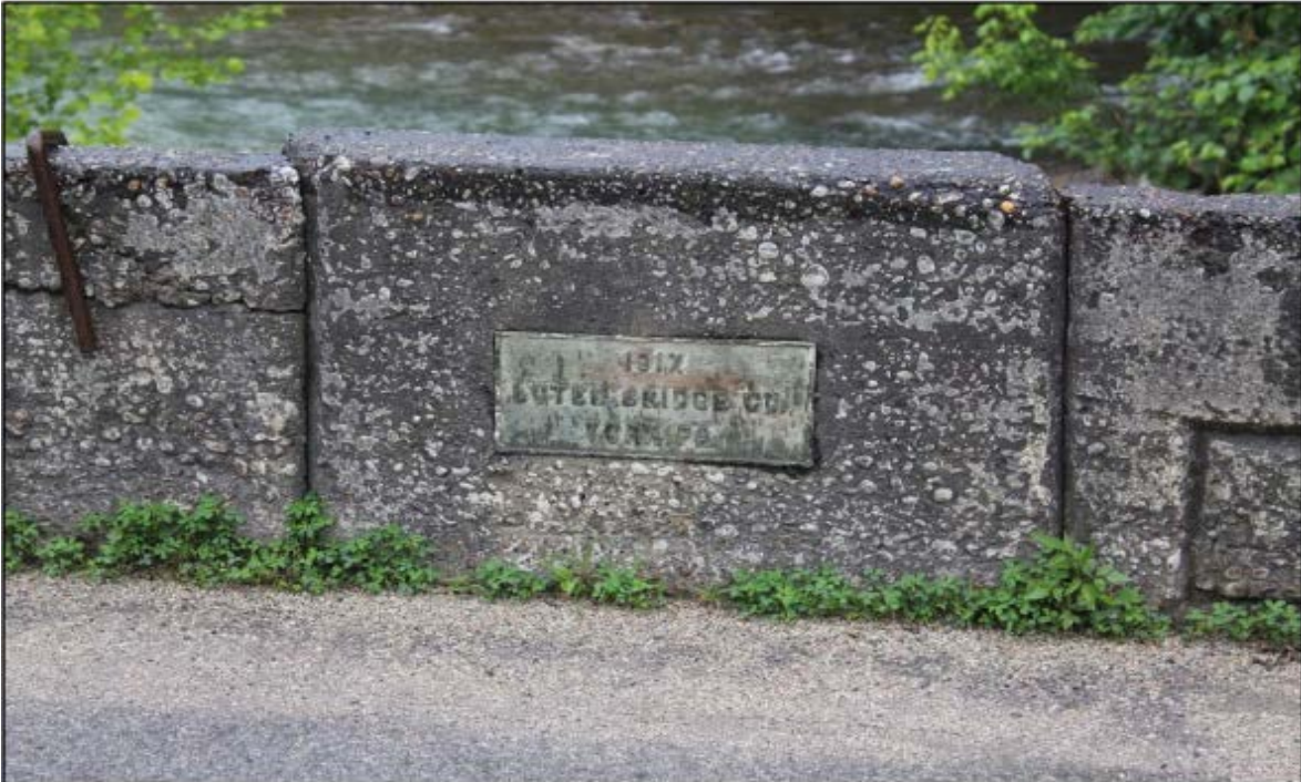
Photograph 7. Mt. Gay Deck Arch Bridge, LG-0758/LG-0764, Facing East
