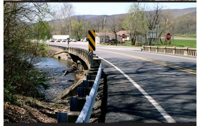
New Creek Bridge is located on US Route 50, just south of Keyser in Mineral County. The bridge was constructed in 1931 by Harmon Brothers Construction Company and consists of three simple reinforced concrete T-beams supported by concrete abutments and two concrete piers. The bridge is 133 feet long and highly skewed.
