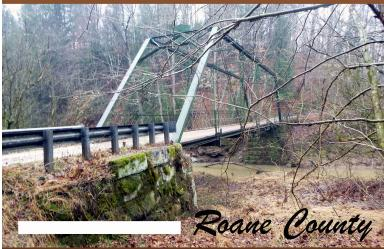
The Pocatalico River Road Truss Bridge is located in Roane County and carries County Route 34 over the Pocatalico River. The Pocatalico River Road Truss Bridge is an 1899 Pratt Truss Bridge with a laminated wood deck, a steel girder substructure, cut stone abutments, and V-Lacing throughout the bridge. The bridge is 103 feet long and 12 feet wide. The main members have "Carnegie" stamps, indicating that the metal superstructure was sourced from Carnegie Steel. The bridge
