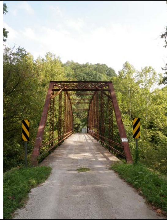
End view looking east
