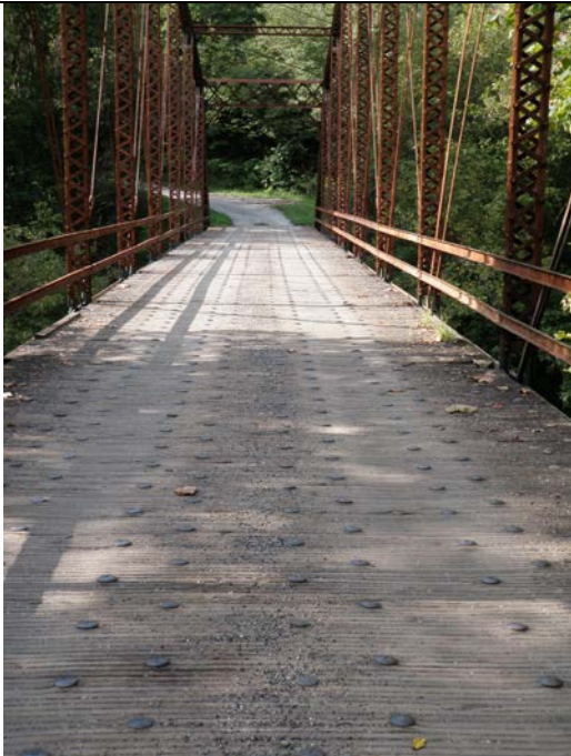
Deck of bridge with dome head bolts
