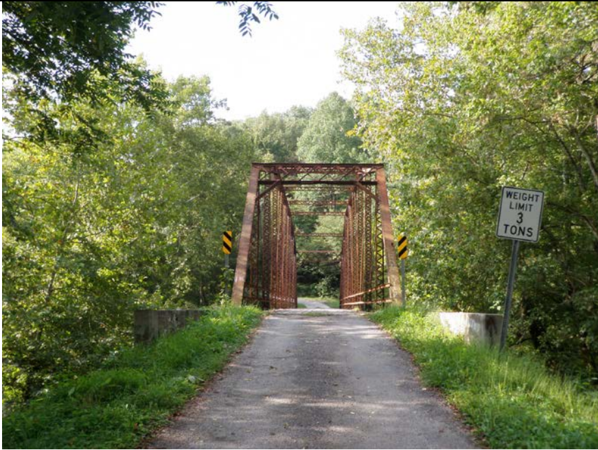
End view looking west
