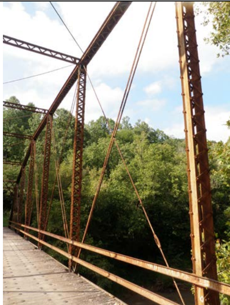
Diagonal bracing
