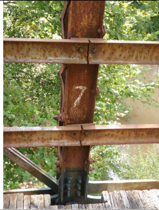
Vertical bracing
