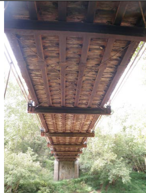
Underside of deck
