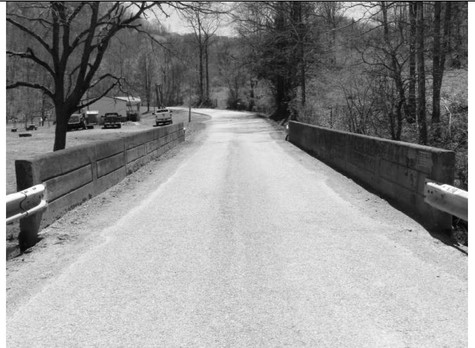
8. North Approach. View Southeast.
