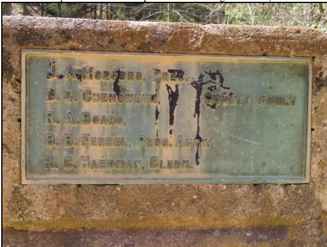
County Commissioner's Plaque at North End of Downstream/West Railing. View SW (WVDOH 4/17/2025)
