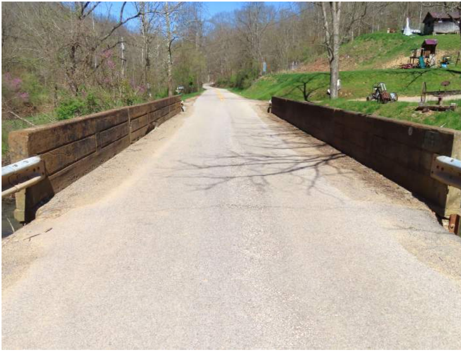
9. South Approach. View Northwest.
