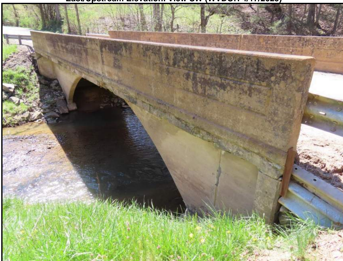
East/Upstream Elevation. View SE (WVDOH 4/17/2025)
