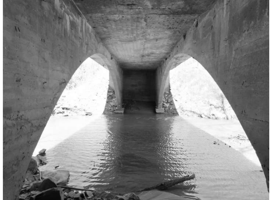
6. Spandrel Walls/Ribs & North Abutment. View Northwest.
