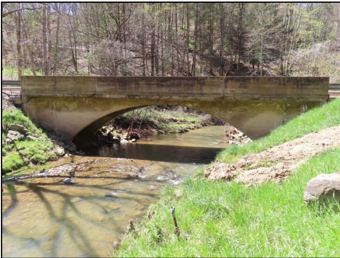
East/Upstream Elevation. View SW (WVDOH 4/17/2025)
