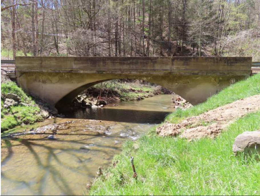
1. East/Upstream Elevation. View Southwest.
