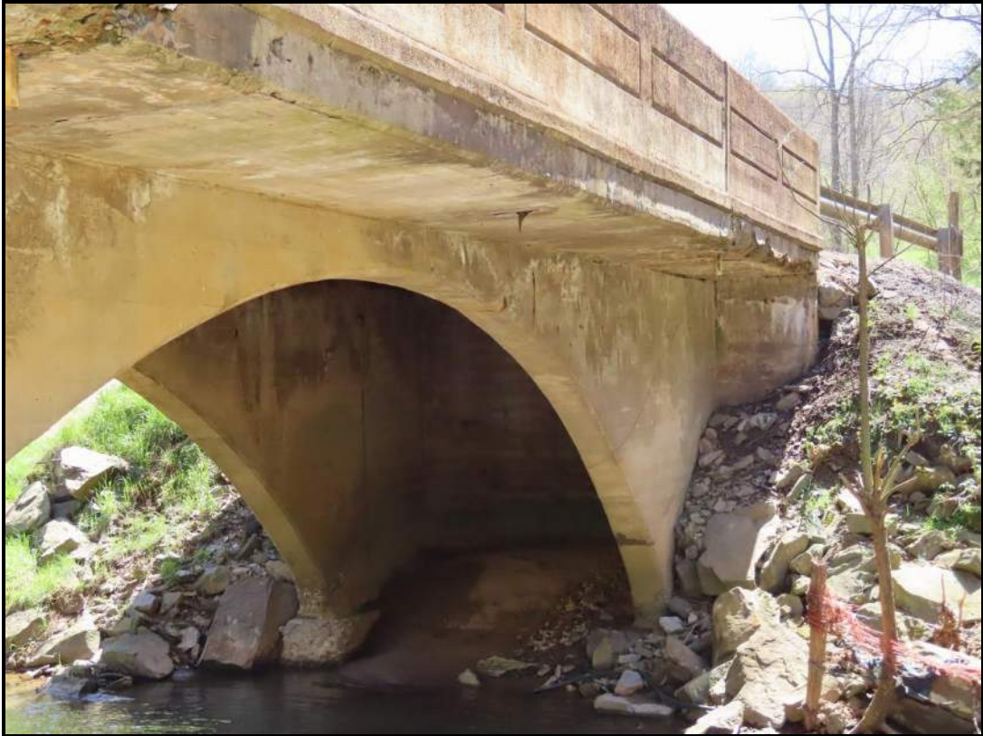
South Abutment, Downstream/West Side. View E (WVDOH 4/17/2025).
