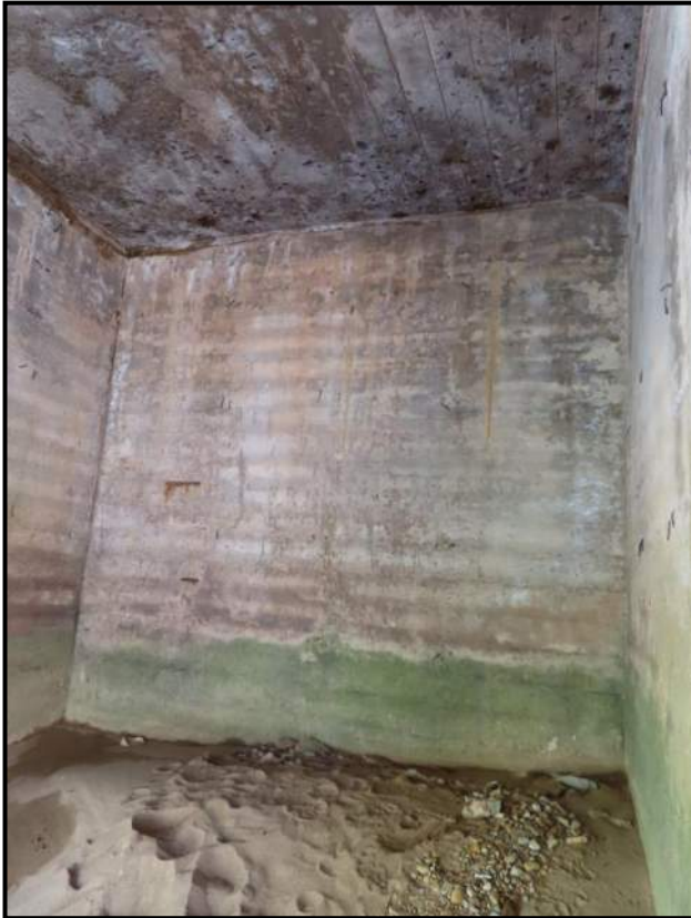
South Abutment Backwall. View SE (WVDOH 4/17/2025)
