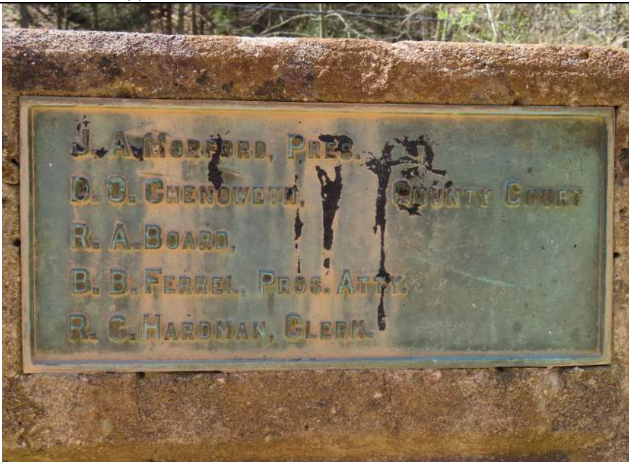
11. County Plaque on Downstream/West Railing. View SW
