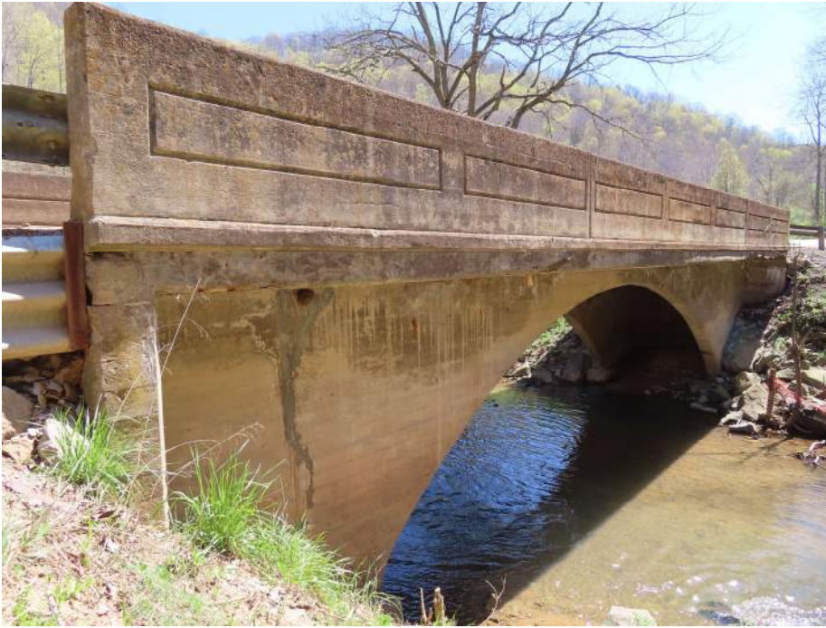
5. West/Downstream Elevation. View Southeast.
