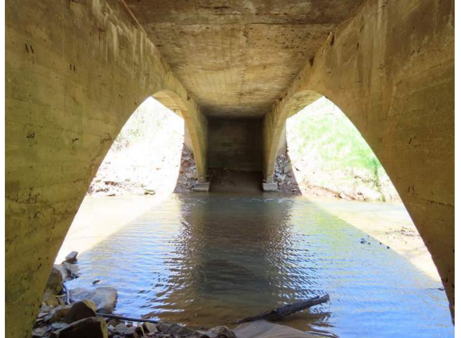
6. Spandrel Walls/Ribs & North Abutment. View Northwest.
