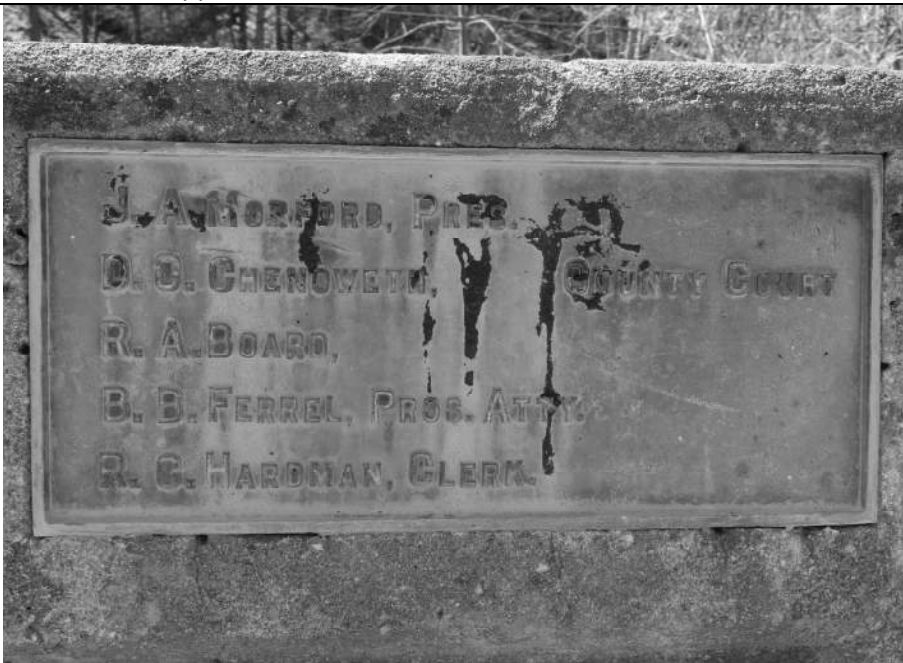
11. County Plaque on Downstream/West Railing. View SW
