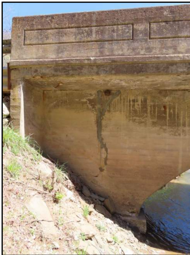
North Abutment, Downstream/West Side. View SW (WVDOH 4/17/2025)
