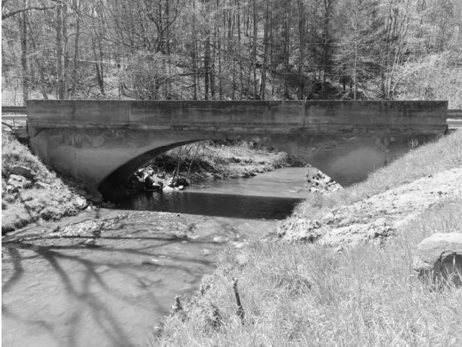
1. East/Upstream Elevation. View Southwest.
