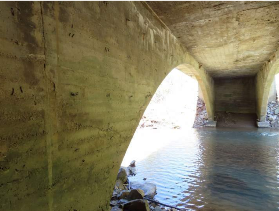
7. West Spandrel Wall/Rib & North Abutment. View Northwest.
