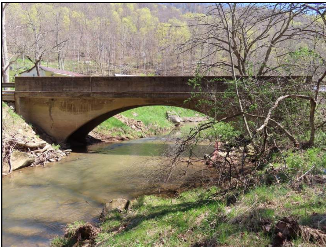
West/Downstream Elevation. View NE (WVDOH 4/17/2025)
