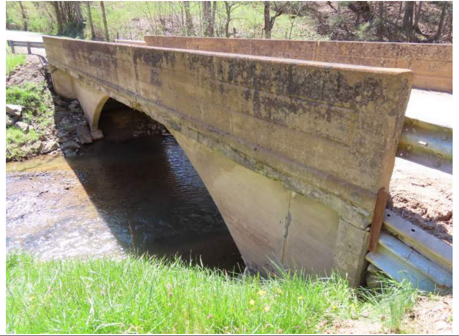
2. East/Upstream Elevation. View Southeast.
