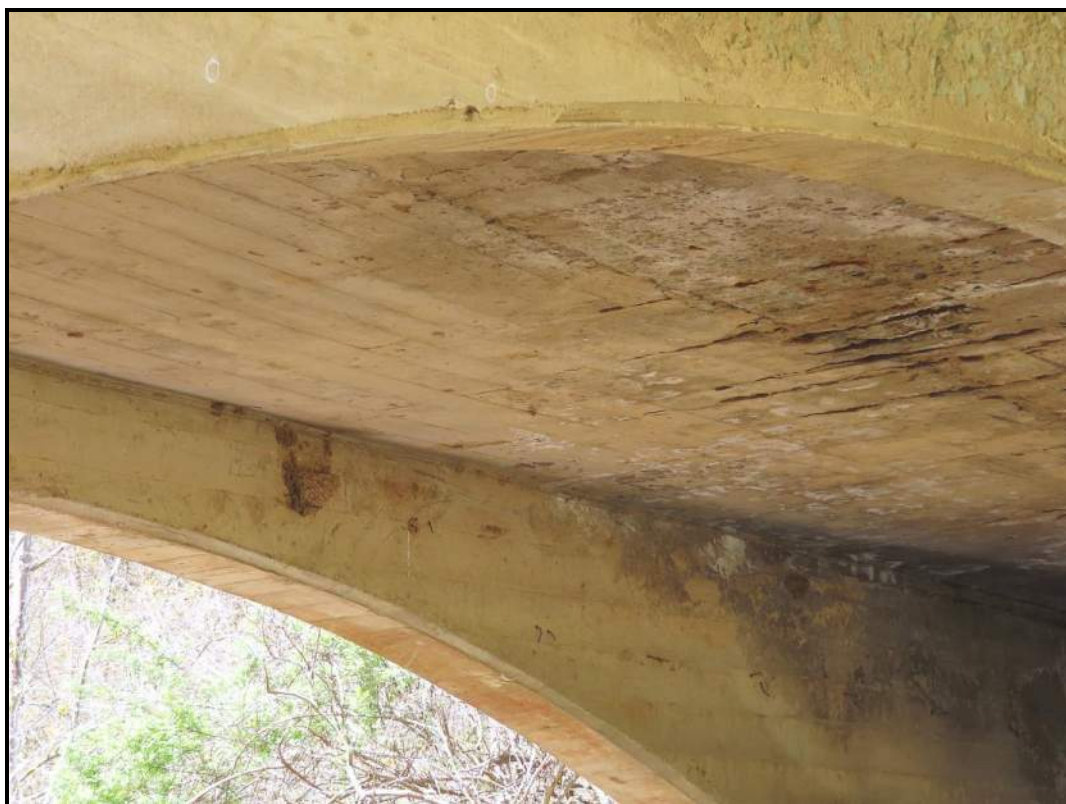
View Highlighting Beveled/Chamfered Edges at Spandrel Arches. View West/Up (WVDOH 4/17/2025)
