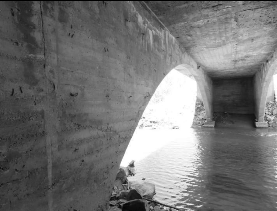
7. West Spandrel Wall/Rib & North Abutment. View Northwest.
