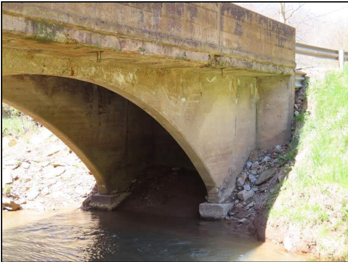
North Abutment, Upstream/East Side. View NW (WVDOH 4/17/2025)
