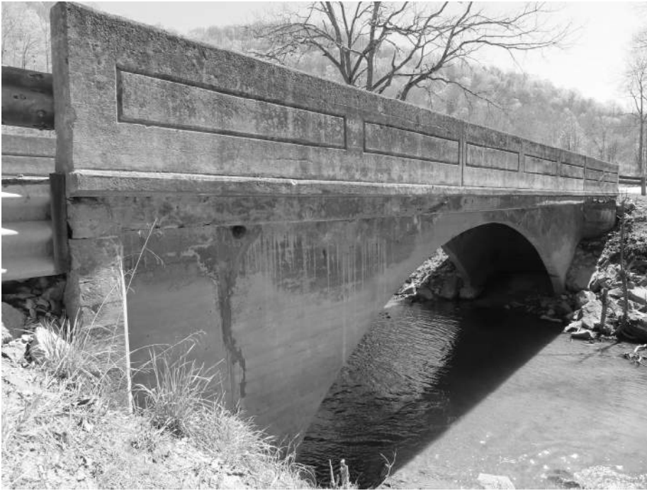
5. West/Downstream Elevation. View Southeast.
