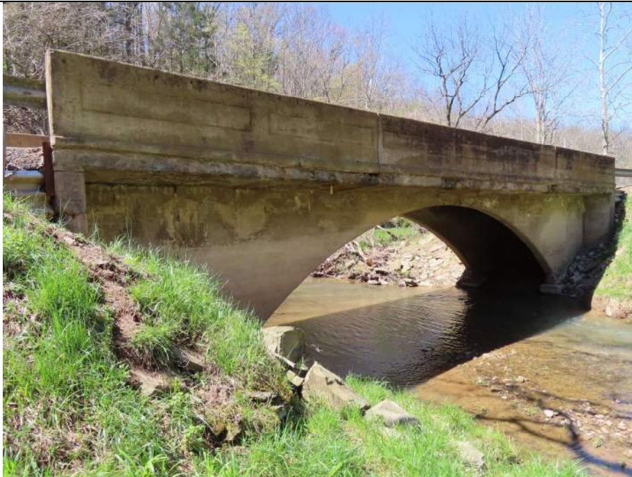
3. East/Upstream Elevation. View West/Northwest.
