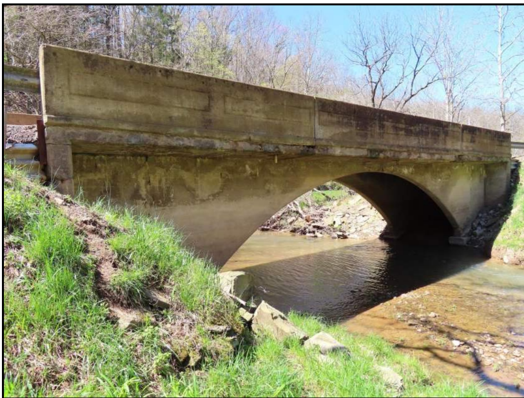
East/Upstream Elevation. View WNW (WVDOH 4/17/2025)
