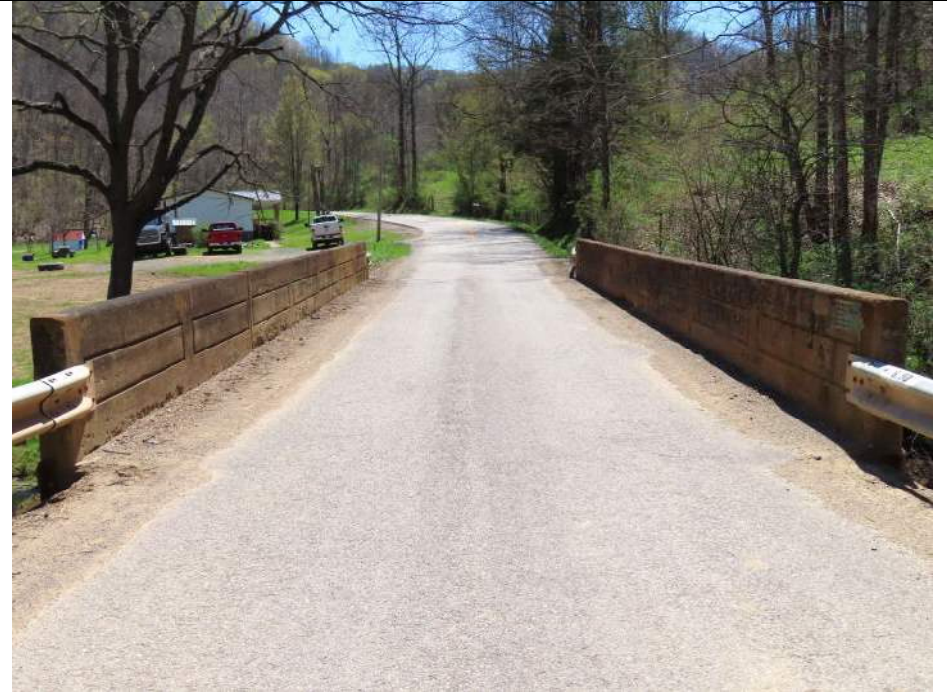
8. North Approach. View Southeast.
