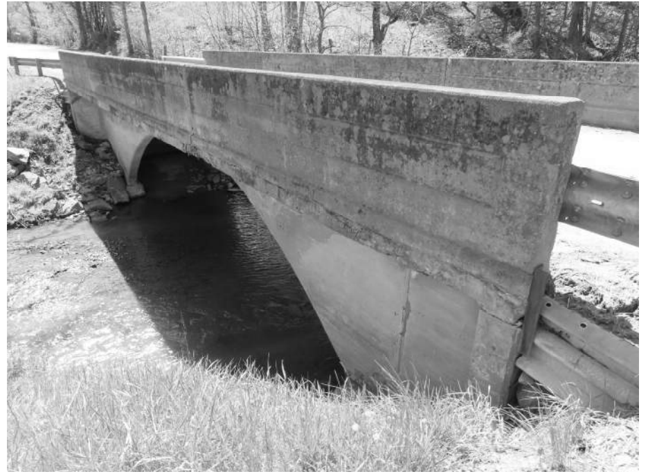
2. East/Upstream Elevation. View Southeast.
