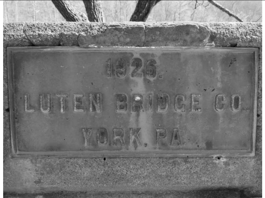
10. Bridge Builder's Plaque on Upstream/East Railing. View Northeast.
