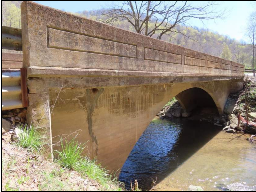
West/Downstream Elevation. View SE (WVDOH 4/17/2025)
