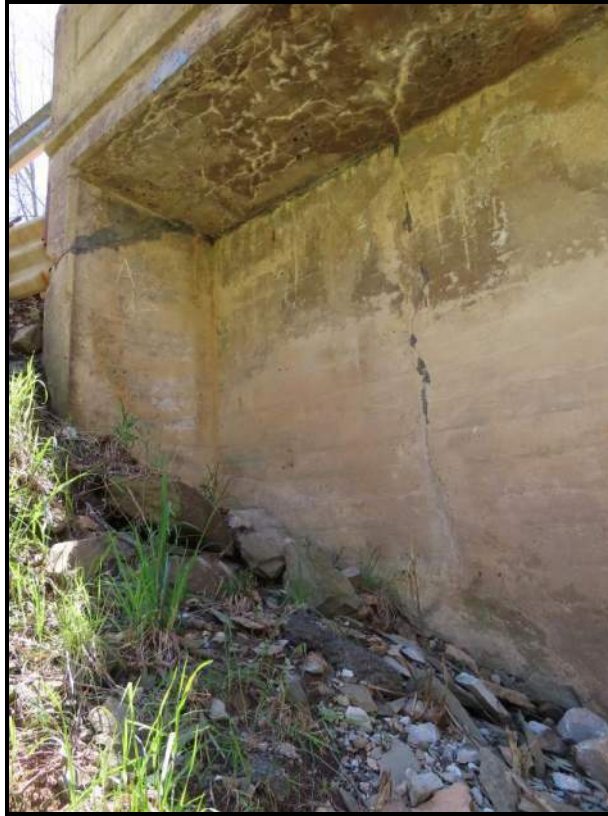
South Abutment, Upstream/East Side. View SSE (WVDOH 4/17/2025).
