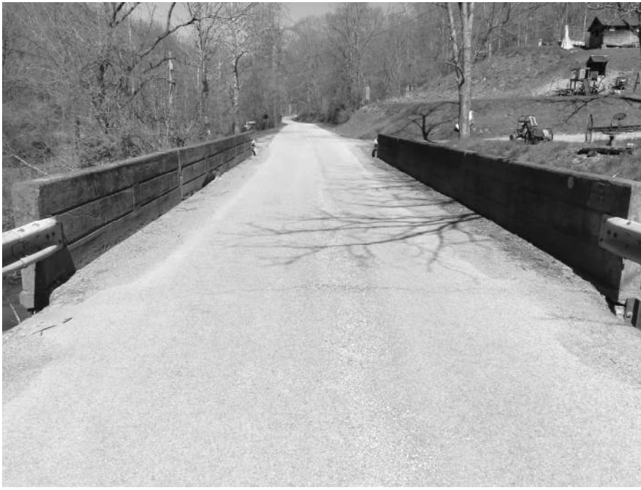
9. South Approach. View Northwest.
