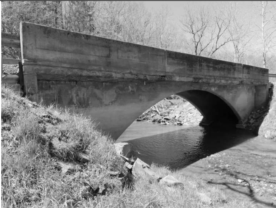
3. East/Upstream Elevation. View West/Northwest.
