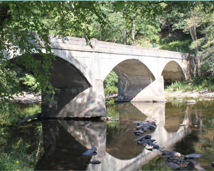
**Location:** County Route 9/3, over Shavers Fork of the Cheat River **Type:** Spandrel Filled Simple Reinforced Concrete Deck Arch Spans
