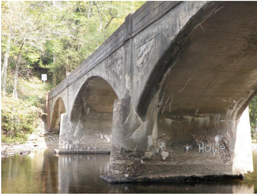
3. Deterioration and Cavities Located on Pier 2 (South Pier), View North
