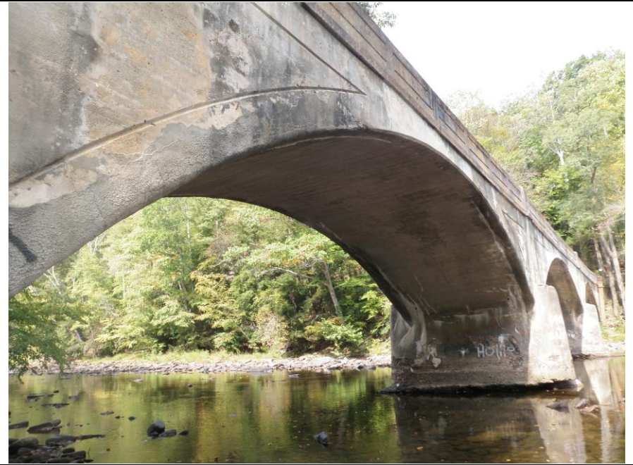
6. Underside of North Arch, Taken from East Side, View Northwest
