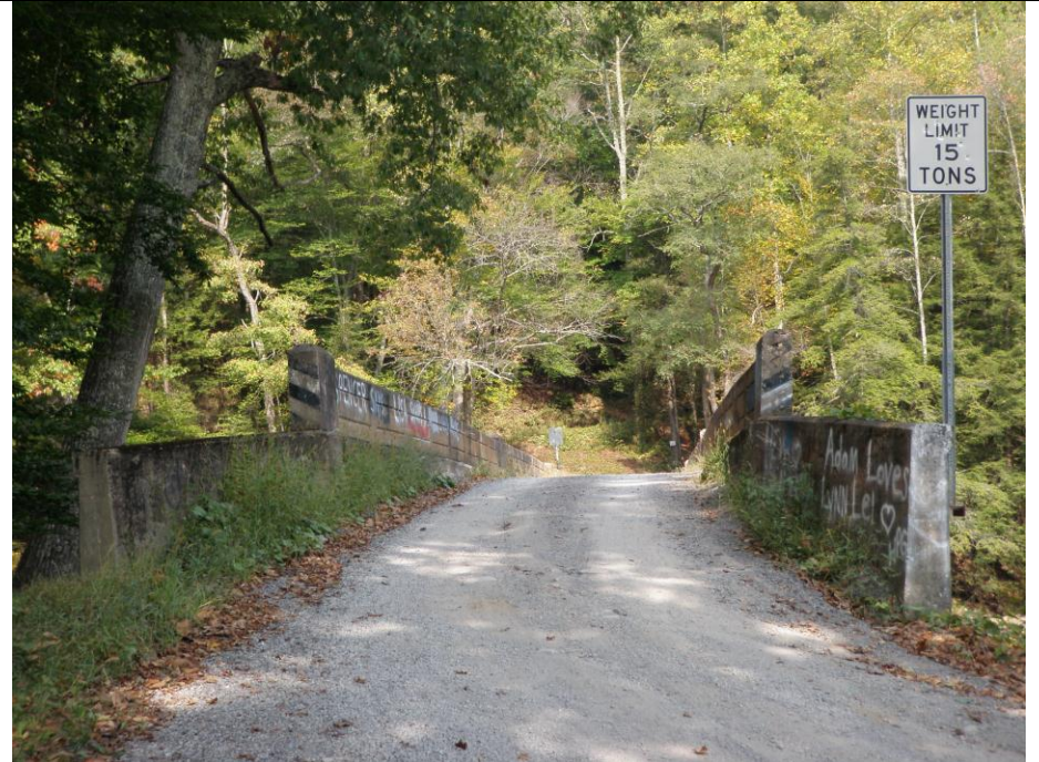
2. End View Looking West Along CR 9/3
