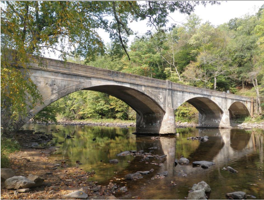
1. East Elevation Looking Upstream, View West
