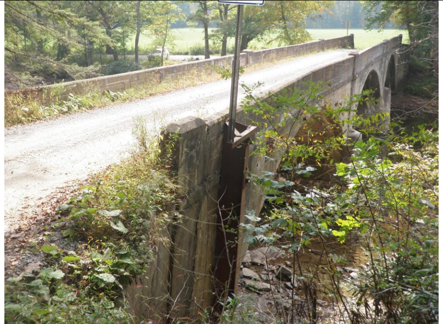
8. Northwest Corner Showing North Entry and West Elevation, View SE
