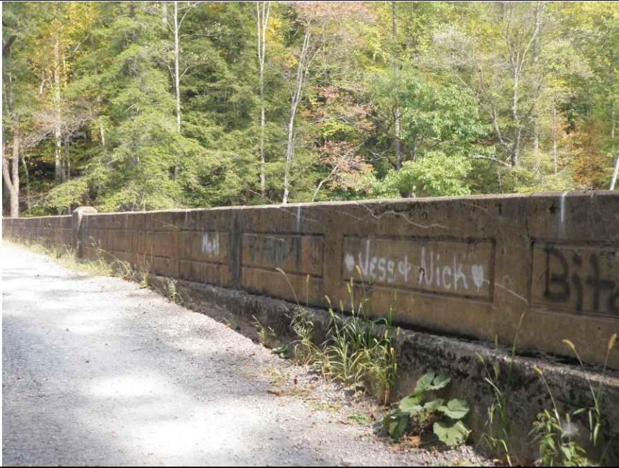
9. East Rail/Parapet, Taken from South Entry (CR 9/3 Side), View North
