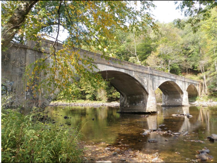
5. East Elevation Looking Upstream, View West
