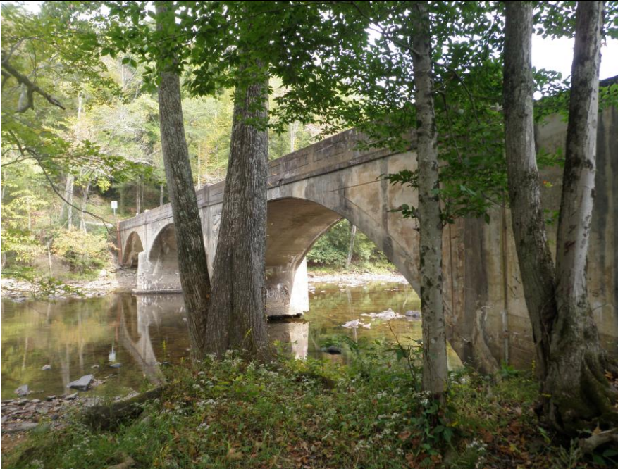
7. West Elevation Looking Downstream, View North
