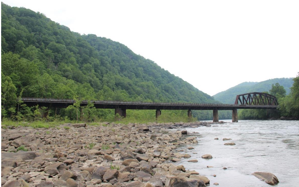
Photo 1: Overall view of east elevation of bridge showing, left to right piers seven through one and spans eight through one, facing northwest.
