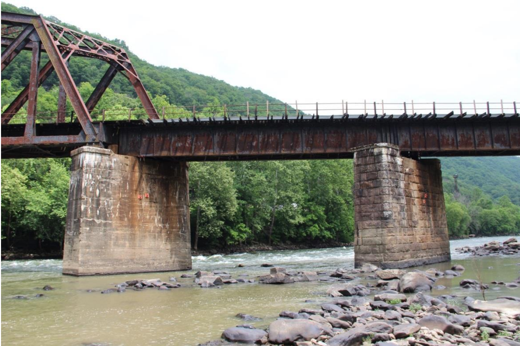
Photo 6: Substructure units: pier one (1915-1916) and pier two (ca. 1890) and superstructure unit: girder span two (center), west elevation, facing southeast.
