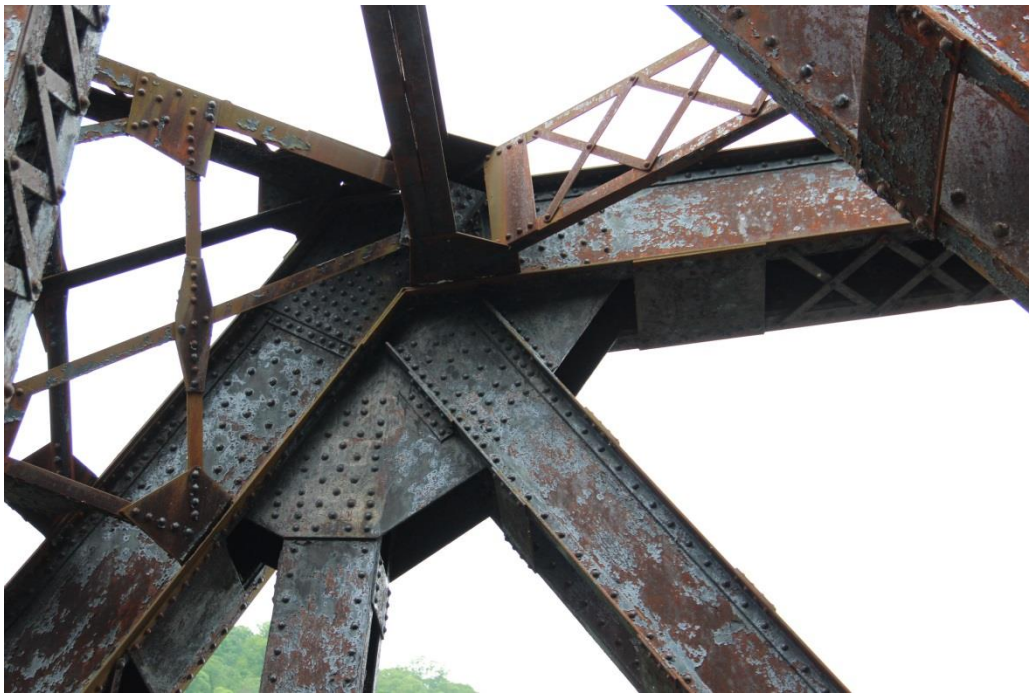
Photo 27: Detail of inner side of west profile of main Warren truss span showing gusset plate connections of top chord, and vertical and diagonal members, facing west.
