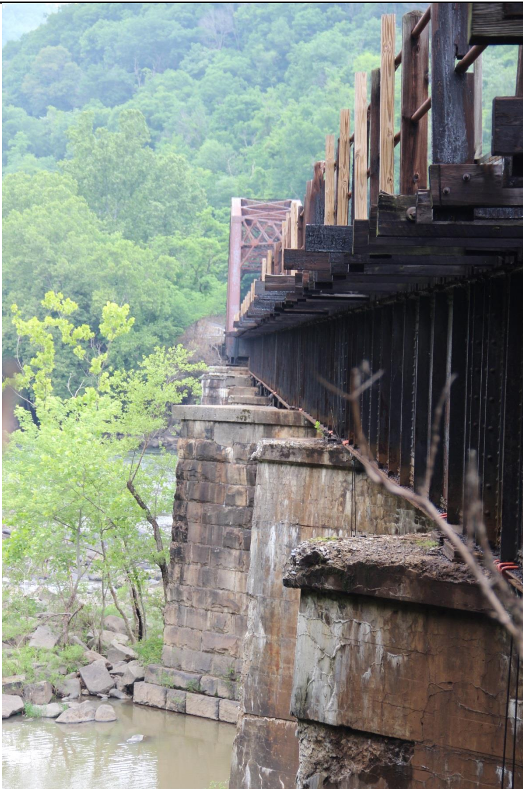
Photo 12: Detail of piers seven (1915-1916), six (1915-1916), and five (ca. 1890), west elevation, facing north.
