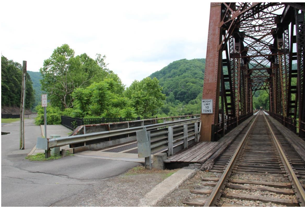
Photo 2: North end of bridge, facing south.
