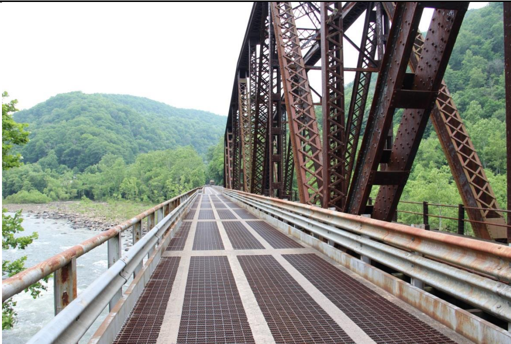
Photo 30: Roadway deck along truss span one, facing south.
