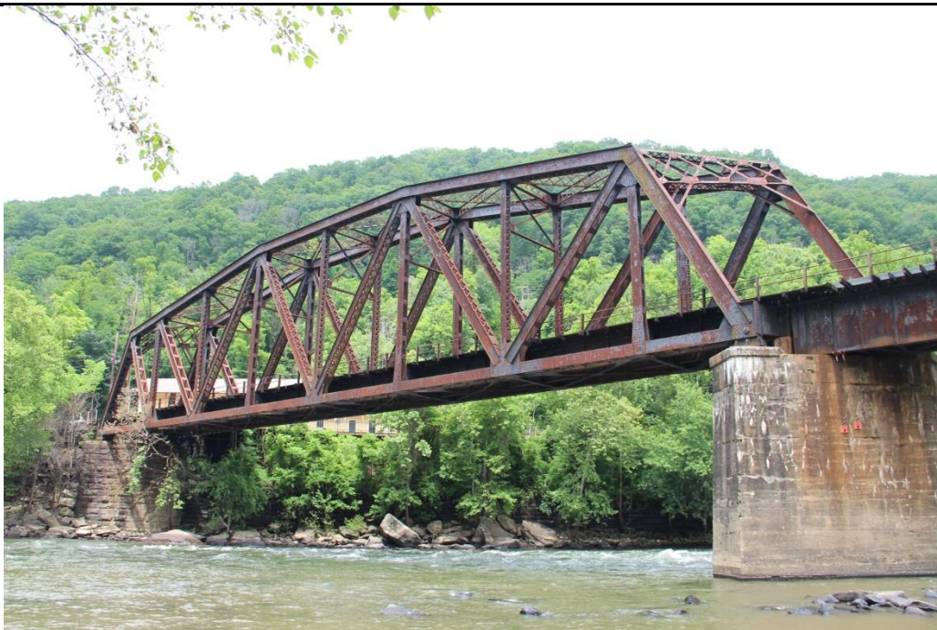
Photo 24: West profile of main Warren truss span, showing skewed south portal, facing northeast.
