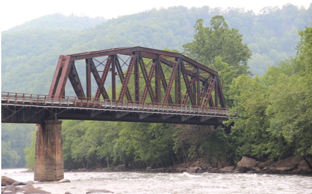
Photo 22: East profile of main Warren truss span, facing northwest.
