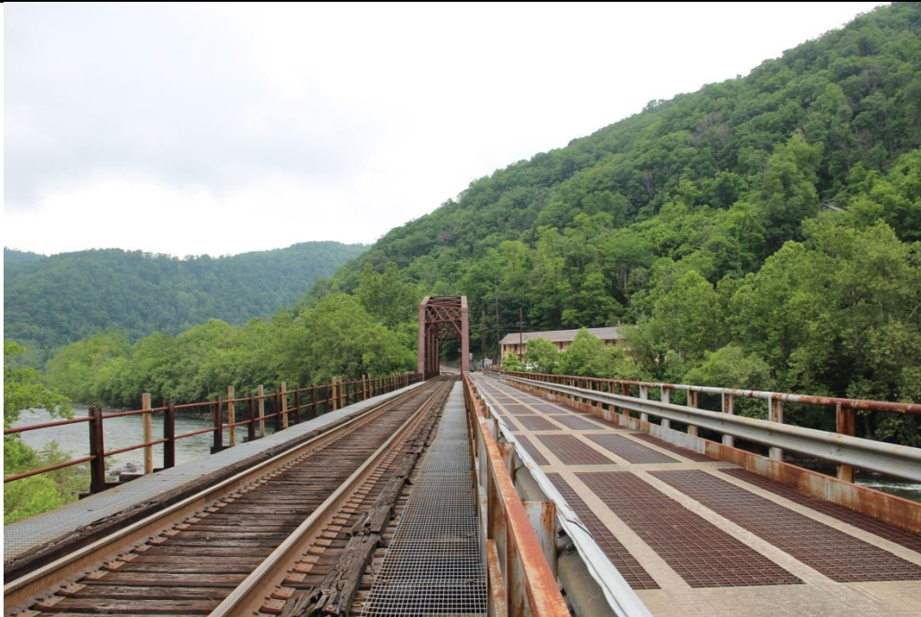
Photo 34: Deck surfaces showing tracks and roadway, facing north.
