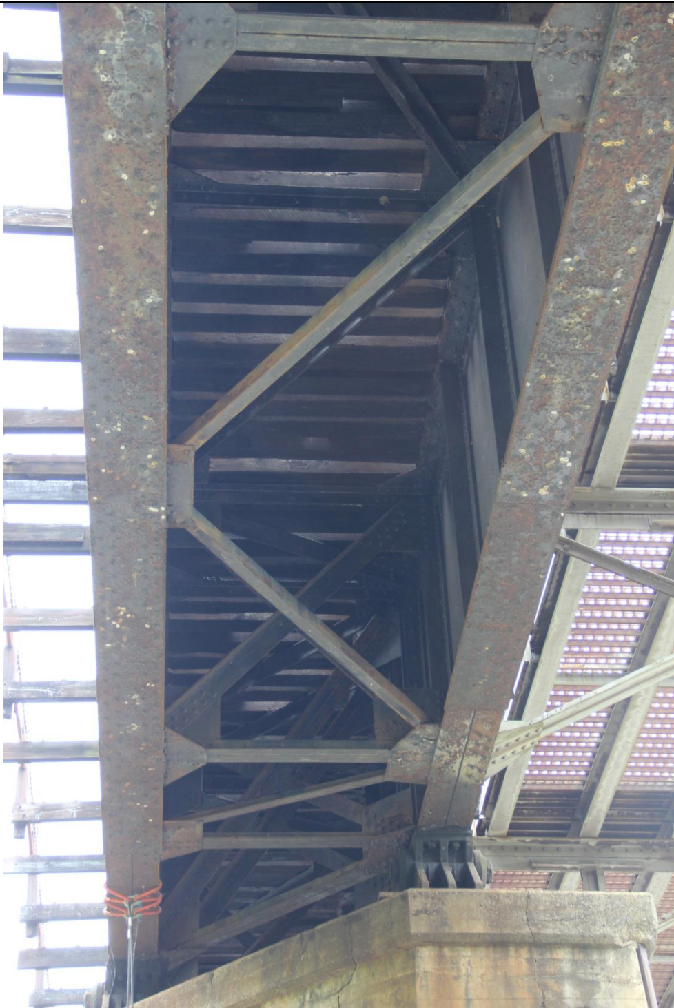
Photo 15: Detail of underside of typical girder span, facing north.
