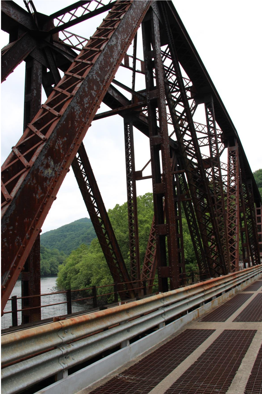
Photo 28: Detail of main Warren span showing lattice braced diagonal members and cross bracing, facing northwest.
