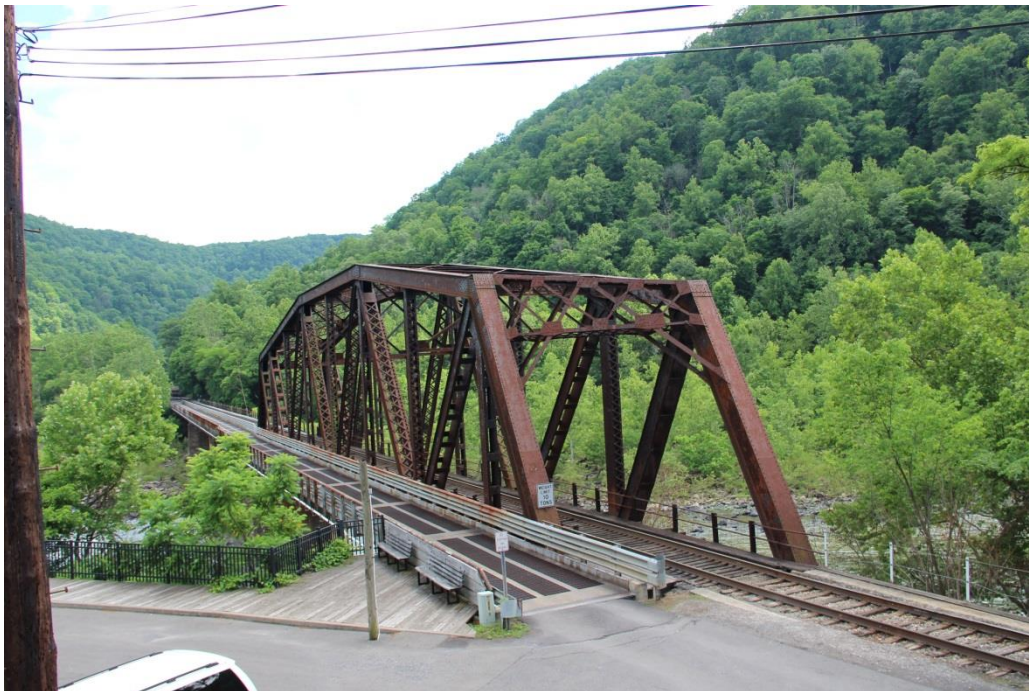
Photo 23: East profile of main Warren truss span, facing southwest.
