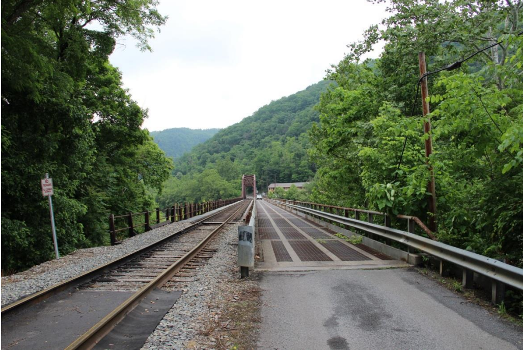
Photo 3: South end of bridge, facing north.
