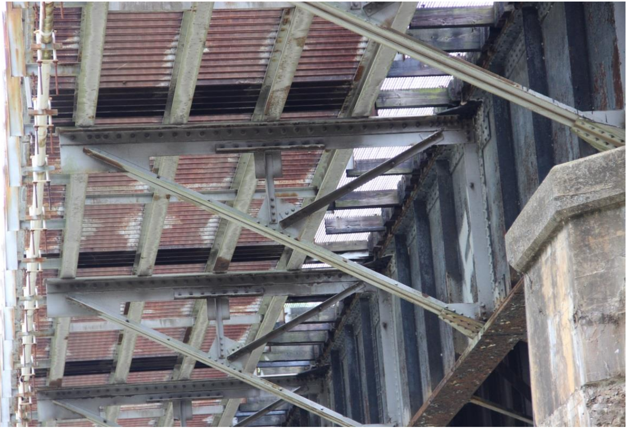
PHOTO 18: DETAIL OF OPEN WEB BRACKETS PROJECTING FROM TYPICAL GIRDER SPAN, FACING SOUTH.
