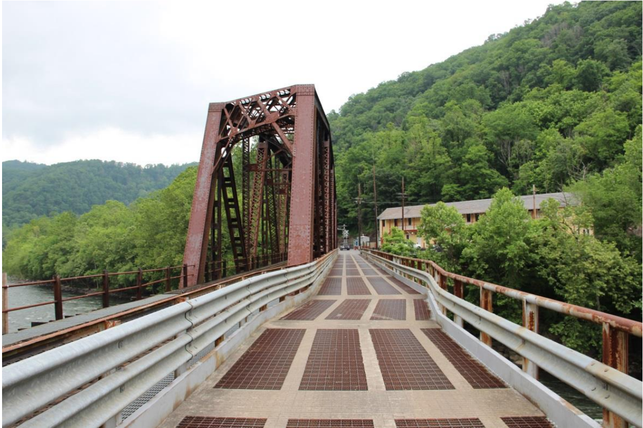
PHOTO 33: ROADWAY DECK SHOWING “BUMP OUT” TRANSITION AREA BETWEEN GIRDER SPANS AND TRUSS SPAN, FACING NORTH.
