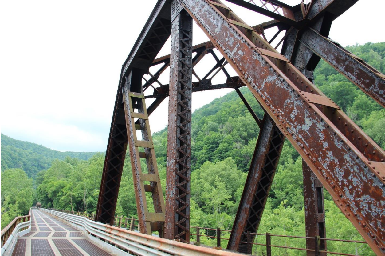
PHOTO 27: DETAIL OF EAST PROFILE OF MAIN WARREN TRUSS SPAN SHOWING TOP CHORD, VERTICAL AND DIAGONAL MEMBERS, AND GUSSET PLATE CONNECTIONS, FACING SOUTHWEST.
