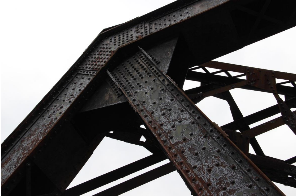
PHOTO 26: DETAIL OF OUTER SIDE OF EAST PROFILE OF MAIN WARREN TRUSS SPAN SHOWING GUSSET PLATE CONNECTIONS OF TOP CHORD AND DIAGONAL MEMBERS, FACING WEST.
