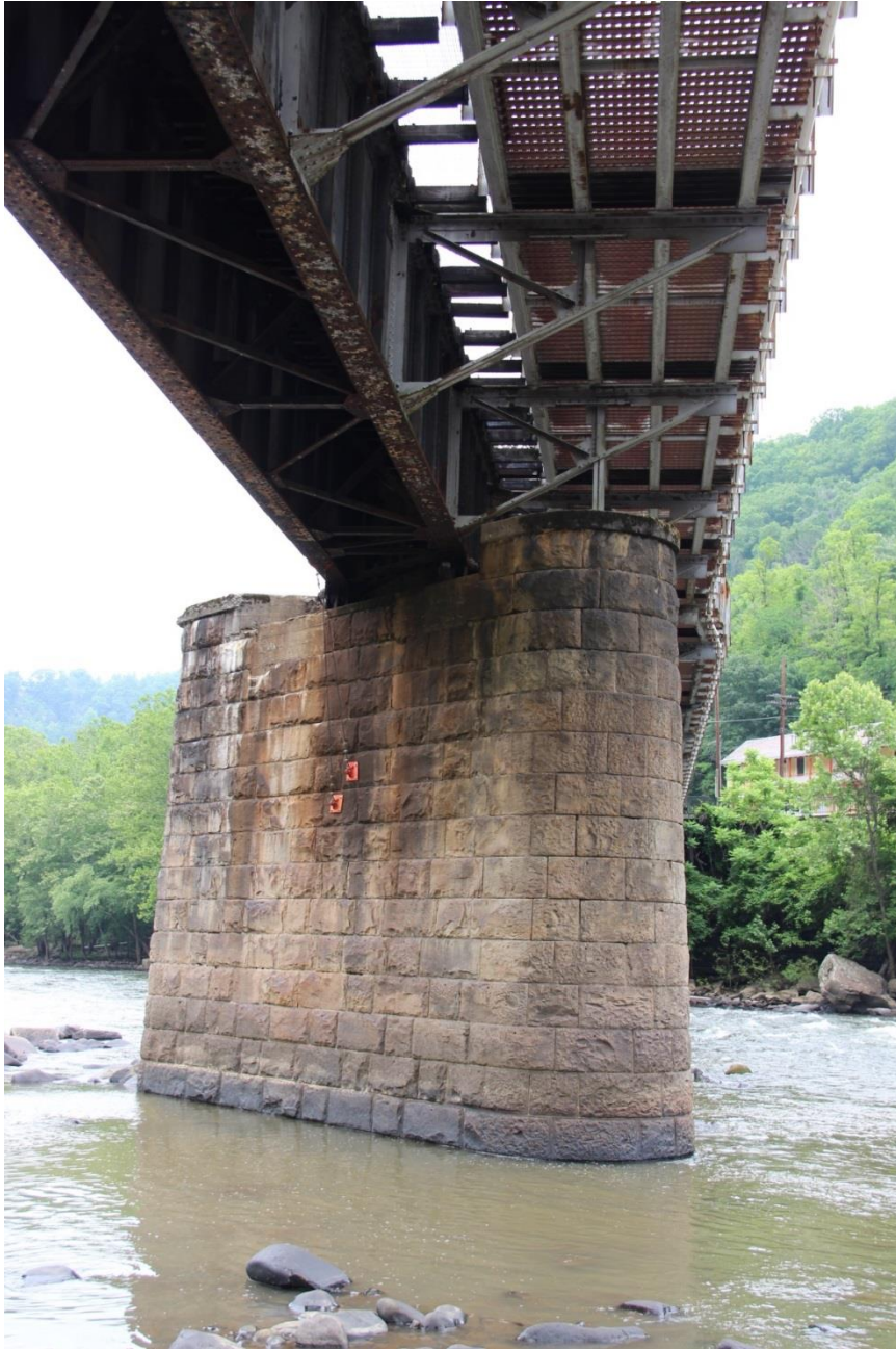
PHOTO 7: DETAIL OF PIER TWO (CA. 1890) SHOWING STONE CONSTRUCTION, FACING NORTH.
