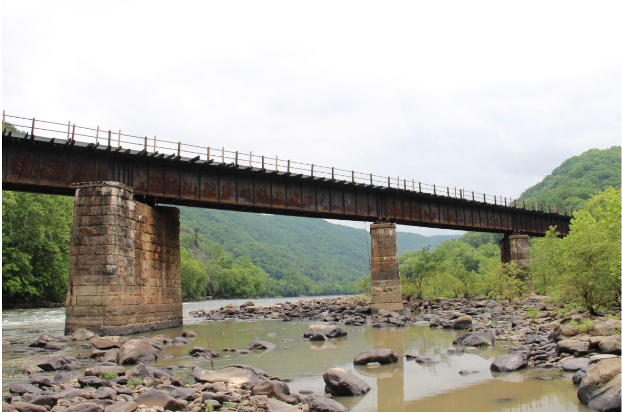
PHOTO 9: SUBSTRUCTURE UNITS: PIER TWO (CA. 1890), PIER THREE (1915-1916), AND PIER FOUR (1915-1916) AND SUPERSTRUCTURE UNITS: GIRDER SPANS THREE AND FOUR, WEST ELEVATION, FACING EAST.
