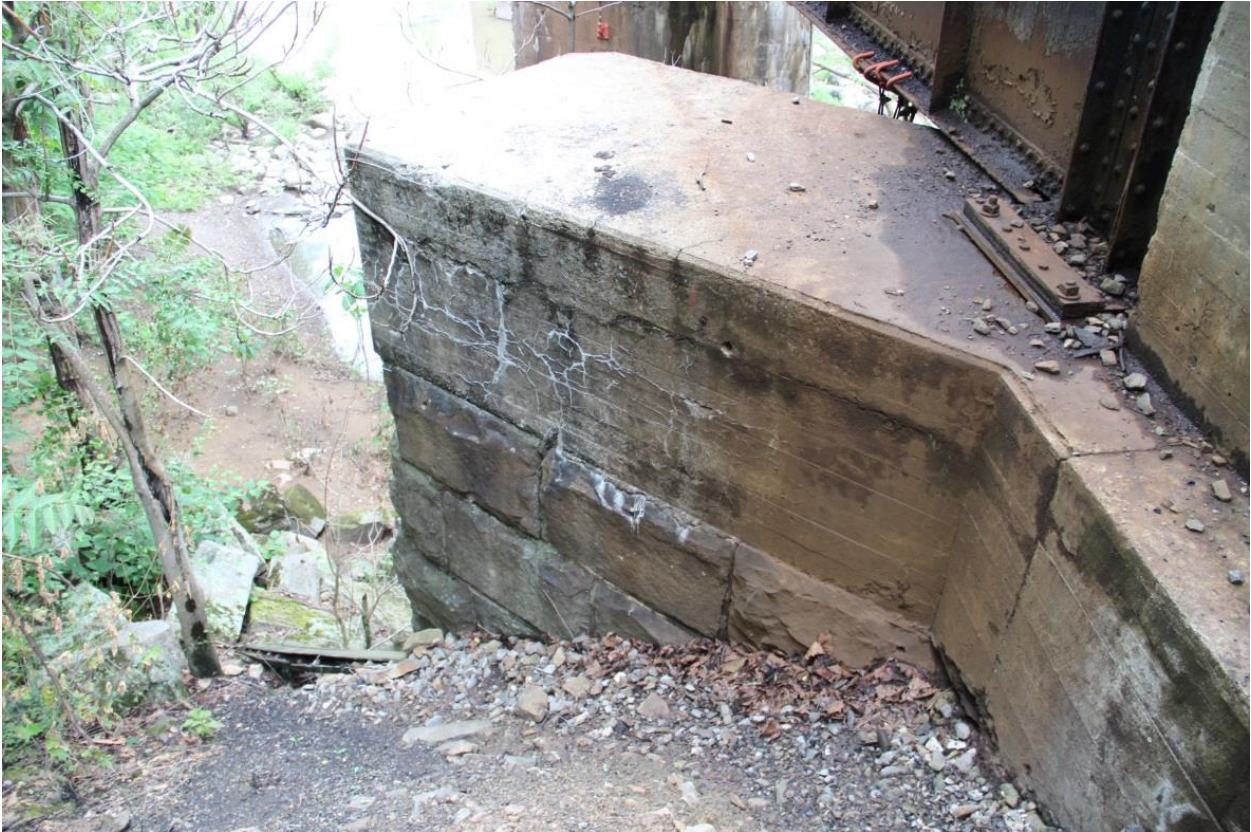
PHOTO 13: SUBSTRUCTURE UNIT: SOUTH STONE ABUTMENT (CA. 1890), SHOWING STONE WING WALL AND POURED CEMENT CAP, FACING NORTH.
