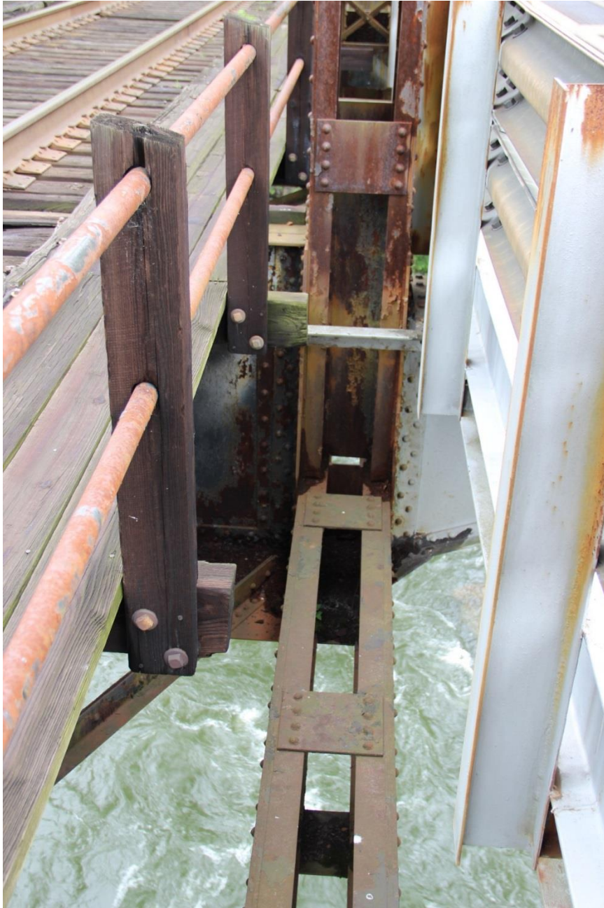
PHOTO 29: DETAIL OF MAIN WARREN TRUSS SPAN SHOWING BOTTOM CHORD AND CONNECTION OF VERTICAL MEMBER, FACING NORTH.
