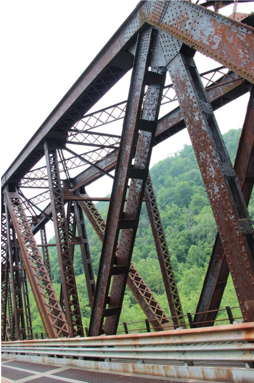
PHOTO 25: DETAIL OF MAIN WARREN TRUSS SPAN SHOWING VERTICAL AND DIAGONAL MEMBERS, TOP CHORD, AND CROSS BRACING, FACING SOUTHWEST.
