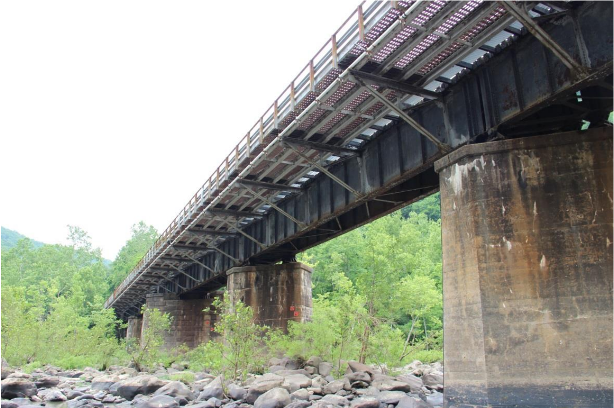
PHOTO 19: CANTILEVERED ROADWAY BETWEEN PIER THREE AND SOUTH ABUTMENT, FACING SOUTH.
