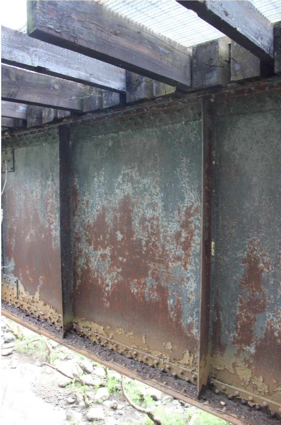
PHOTO 14: DETAIL OF RIVETED PLATE GIRDER IN SPAN 8, FACING NORTHEAST.
