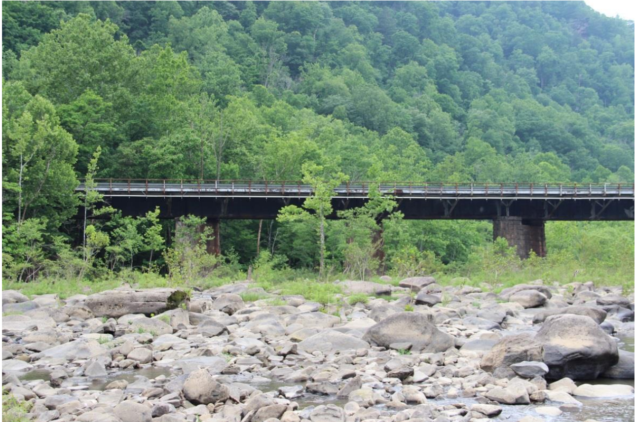
PHOTO 11: SUBSTRUCTURE UNITS: PIER SEVEN (1915-1916), PIER SIX (1915-1916), AND PIER FIVE (CA. 1890) AND SUPERSTRUCTURE UNITS: GIRDER SPANS EIGHT, SEVEN, SIX AND A PORTION OF SPAN FIVE, EAST ELEVATION, FACING WEST.
