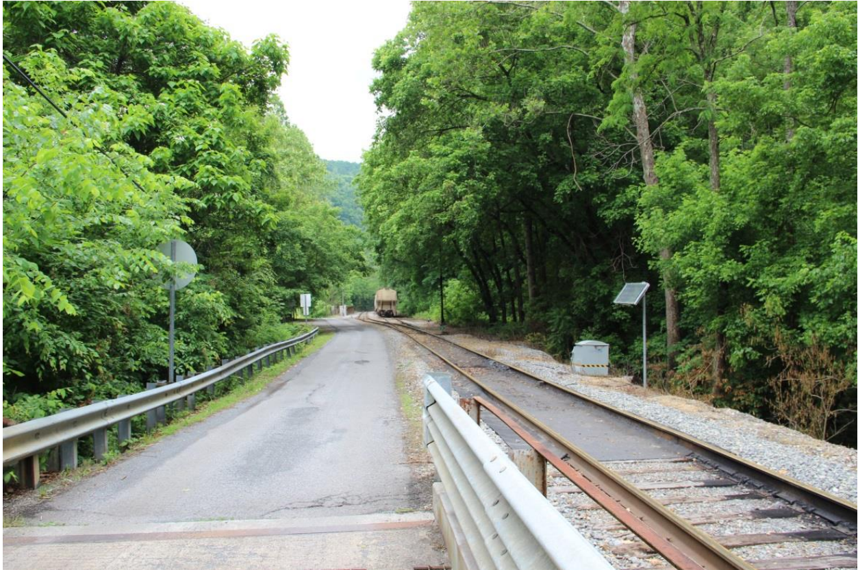
PHOTO 37: FAYETTE COUNTY ROUTE 25/2 AND DUNLOUP BRANCH RAILROAD AT SOUTH END OF BRIDGE, FACING SOUTH.
