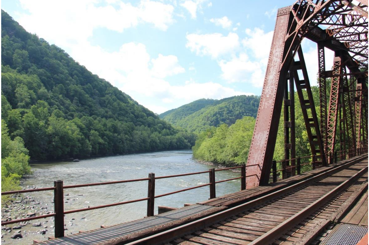
PHOTO 35: STANDARD RAILROAD DESIGN HANDRAIL ALONG WEST SIDE OF BRIDGE, FACING WEST.
