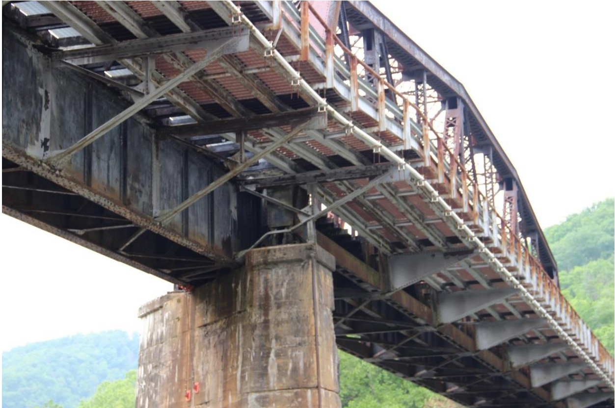
PHOTO 16: CANTILEVERED ROADWAY ALONG EAST ELEVATION OF BRIDGE SHOWING SOLID BRACKETS PROJECTING FROM TRUSS SPAN ONE AND OPEN BRACKETS PROJECTING FROM GIRDER SPAN TWO, FACING NORTHWEST.
