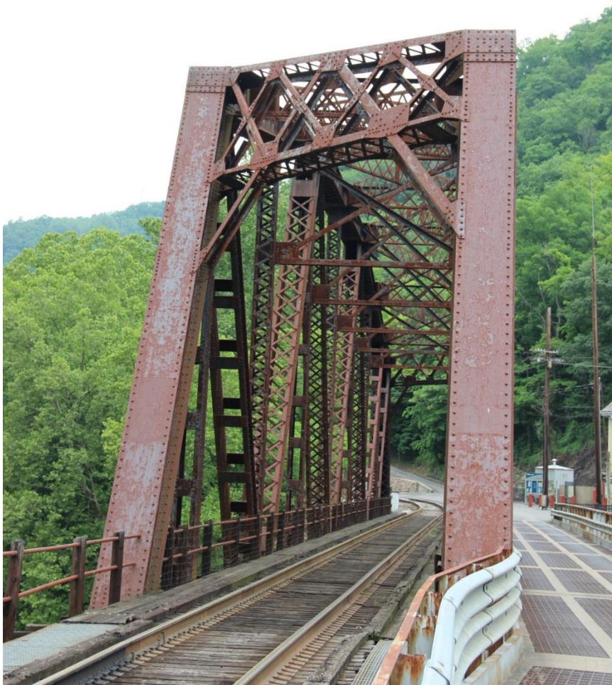
PHOTO 21: SKEWED SOUTH PORTAL OF MAIN WARREN TRUSS SPAN, FACING NORTH.
