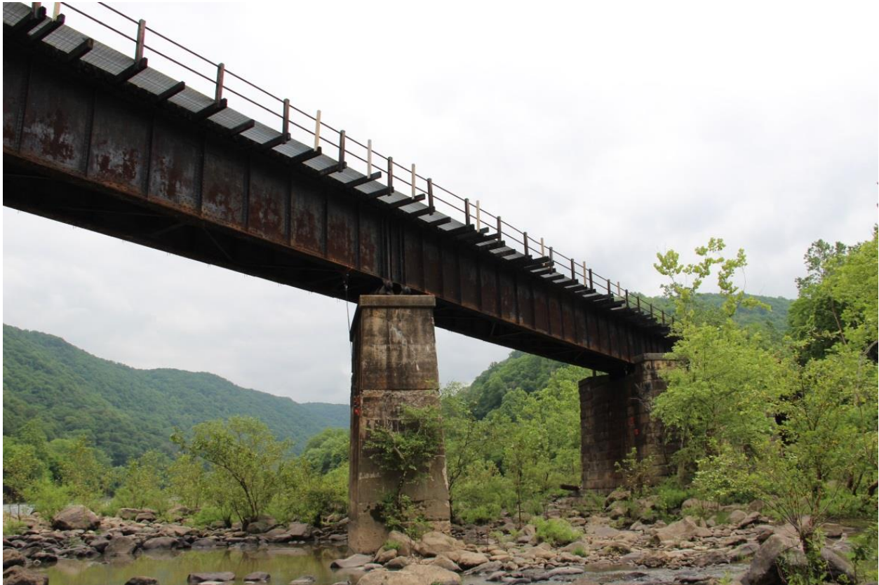
PHOTO 10: SUBSTRUCTURE UNITS: PIER FOUR (1915-1916) AND PIER FIVE (CA. 1890) AND SUPERSTRUCTURE UNITS: GIRDER SPANS FOUR AND FIVE, WEST ELEVATION, FACING SOUTHEAST.
