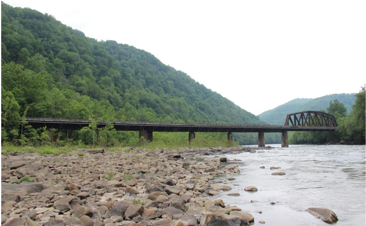
PHOTO 1: OVERALL VIEW OF EAST ELEVATION OF BRIDGE SHOWING, LEFT TO RIGHT, PIERS SEVEN THROUGH ONE AND SPANS EIGHT THROUGH ONE, FACING NORTHWEST.
