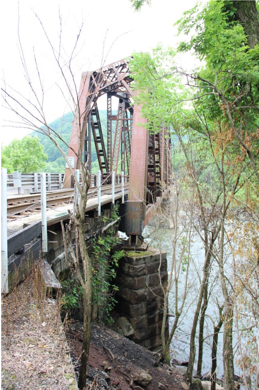
PHOTO 4: SUBSTRUCTURE UNIT: NORTH STONE ABUTMENT (CA. 1890) AND SUPERSTRUCTURE UNIT: WARREN TRUSS SPAN ONE SHOWING NORTH PORTAL, FACING SOUTHEAST.
