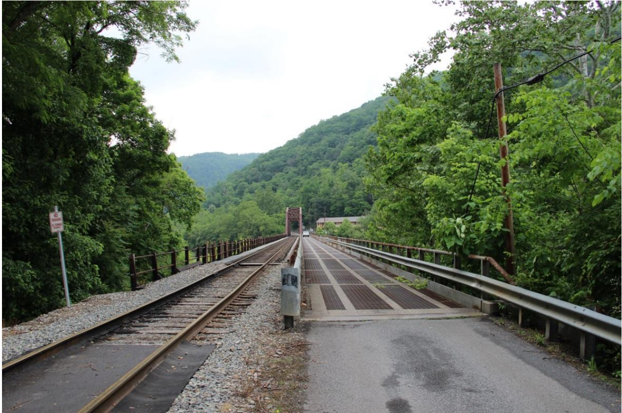
PHOTO 3: SOUTH END OF BRIDGE, FACING NORTH.
