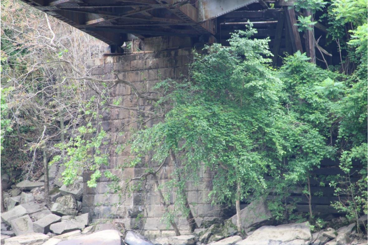
PHOTO 5: SUBSTRUCTURE UNIT: DETAIL OF NORTH STONE ABUTMENT (CA. 1890), FACING NORTHWEST.
