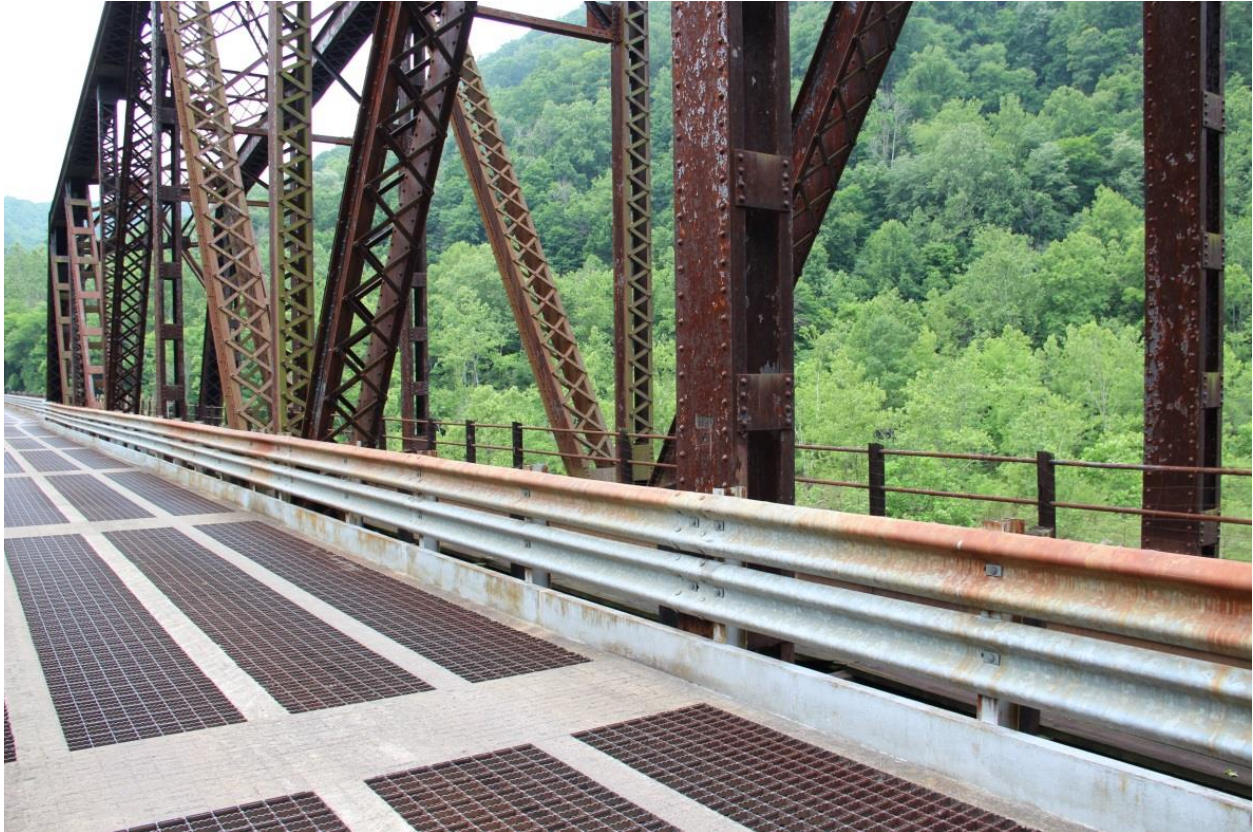
PHOTO 32: DETAIL OF ROADWAY DECK ALONG TRUSS SPAN ONE SHOWING INNER GUARDRAIL, FACING SOUTHWEST.
