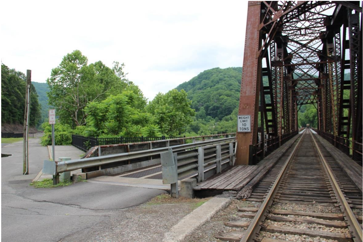
PHOTO 2: NORTH END OF BRIDGE, FACING SOUTH.
