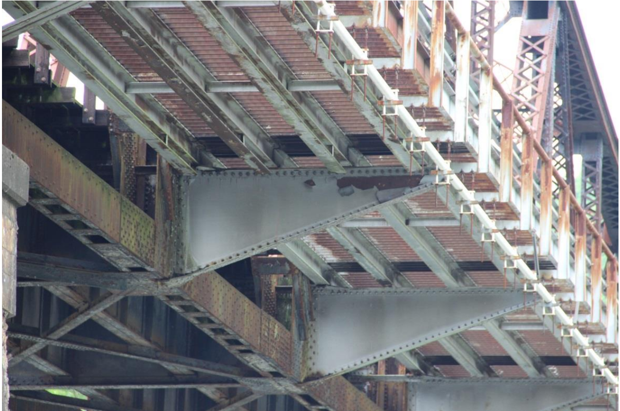
PHOTO 17: DETAIL OF SOLID WEB BRACKETS PROJECTING FROM TRUSS SPAN ONE, FACING NORTHWEST.
