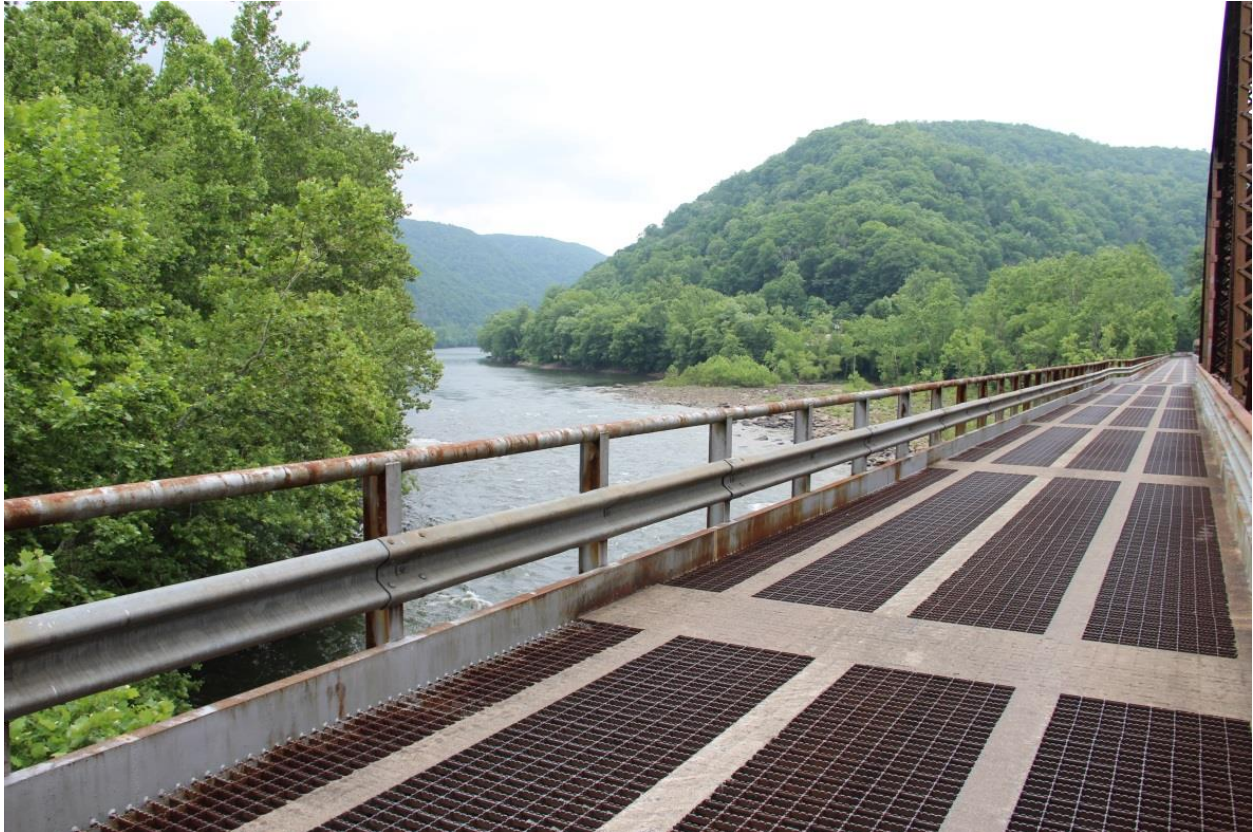
PHOTO 31: DETAIL OF ROADWAY DECK ALONG TRUSS SPAN ONE SHOWING OUTER GUARDRAIL, FACING SOUTHEAST.
