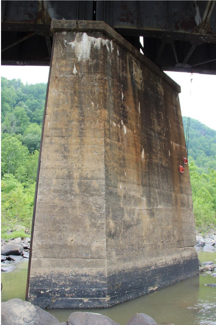
PHOTO 8: DETAIL OF PIER FOUR (1915-1916), SHOWING POURED CONCRETE CONSTRUCTION, FACING SOUTHWEST.
