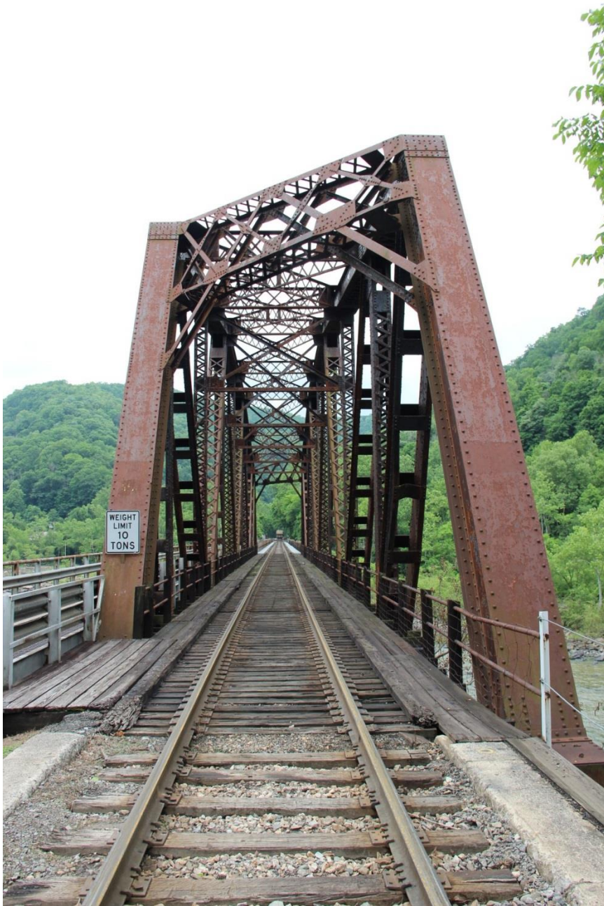
PHOTO 20: SKEWED NORTH PORTAL OF MAIN WARREN TRUSS SPAN, FACING SOUTH.
