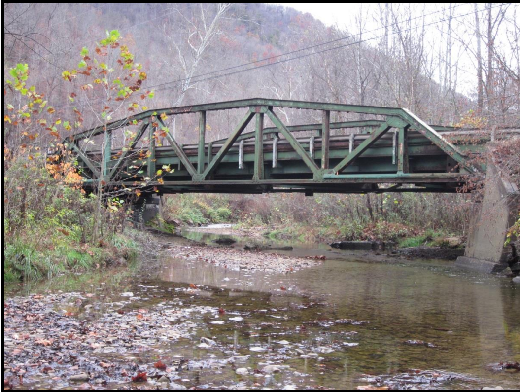
West (Downstream) Elevation. View NE (WVDOH 11-10-2015)
