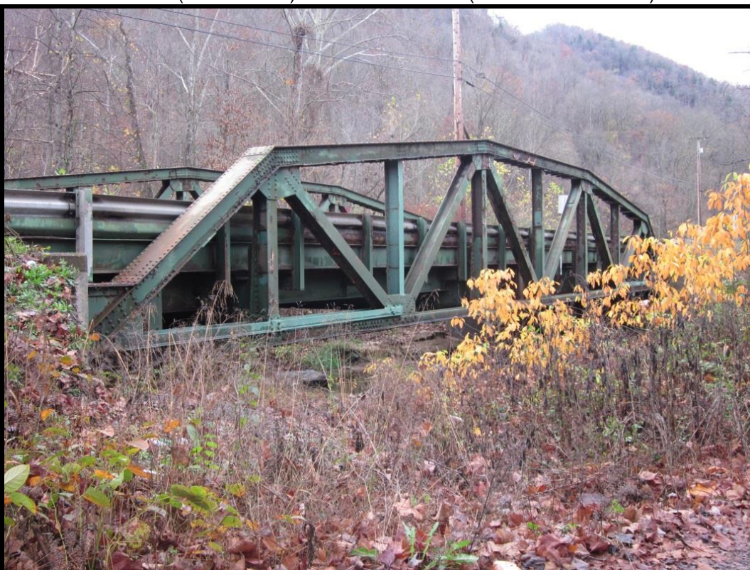
West (Downstream) Elevation. View SE (WVDOH 11-10-2015)
