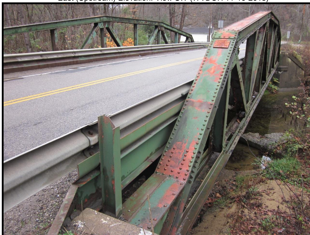
East Truss with Builder's Plaque. View NW (WVDOH 11-10-2015)
