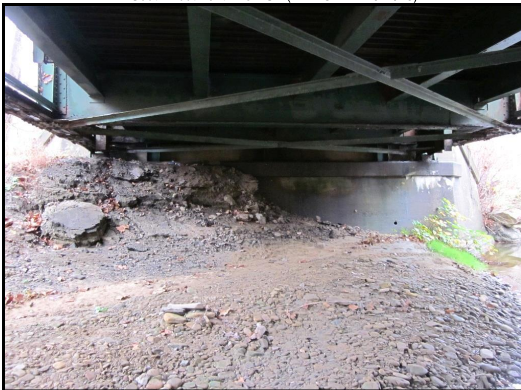
North Abutment. View N/NW (WVDOH 11-10-2015)
