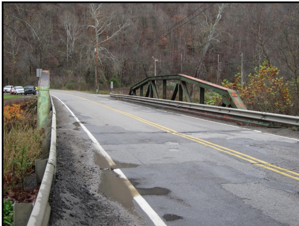
South Approach. View NE (WVDOH 11-10-2015)
