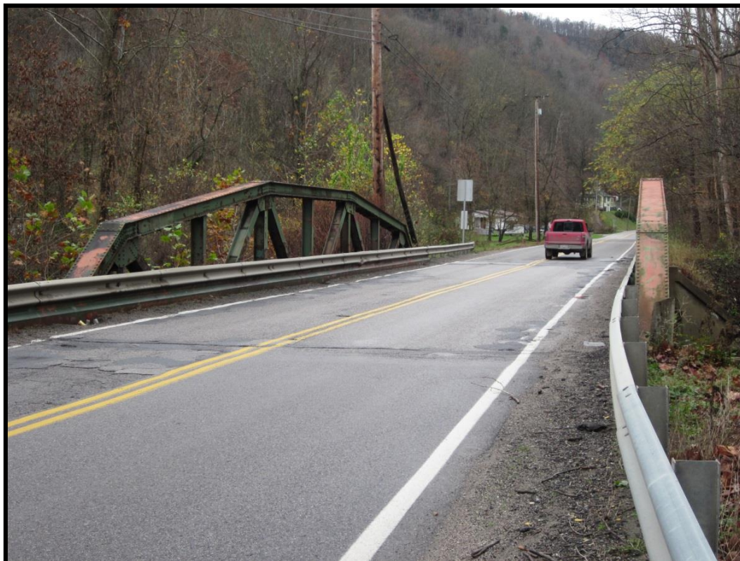
North Approach. View SE (WVDOH 11-10-2015)
