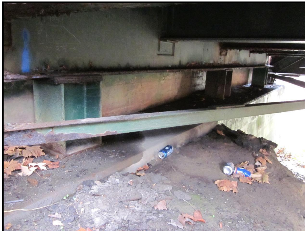
Typical End Floorbeam Support Posts at Bridge Seat; view is of North Abutment View NE (WVDOH 11-10-2015)
