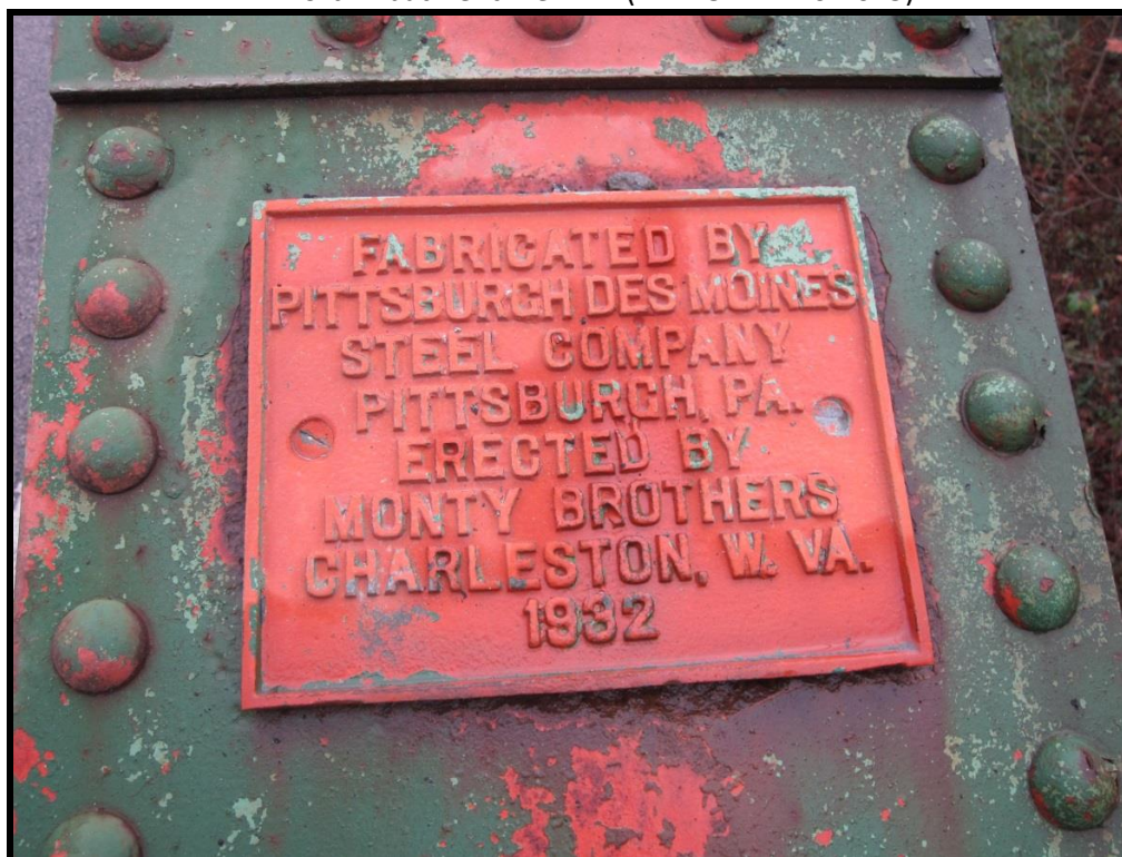
Bridge Builder's Plaque at South End Post of East Truss. View N (down; WVDOH 11-10-2015)
