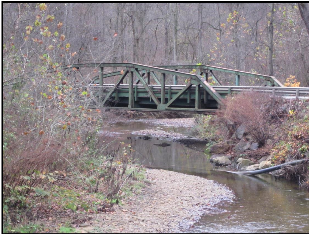
East (Upstream) Elevation. View SW (WVDOH 11-10-2015)
