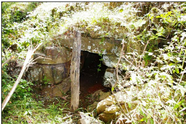
Inlet Side of Culvert
