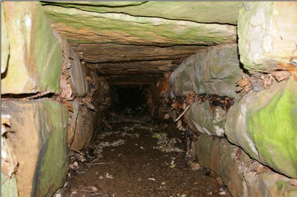
Inside of Culvert on the Inlet Side
