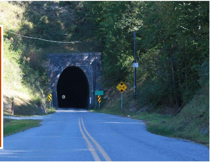
Location: County Route 3/5 in Mingo County Type: Stone Masonry Tunnel Year constructed: 1892 Length: 3,331 feet
