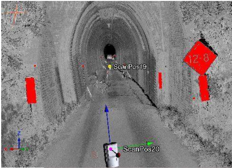
North Entrance of Tunnel
