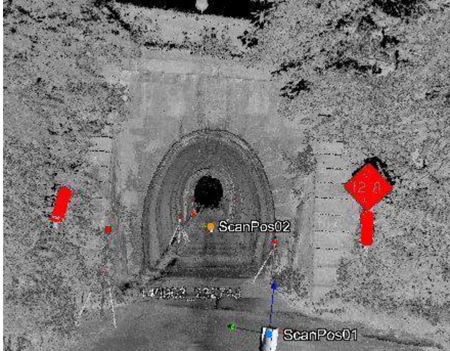
South End Tunnel Entrance
