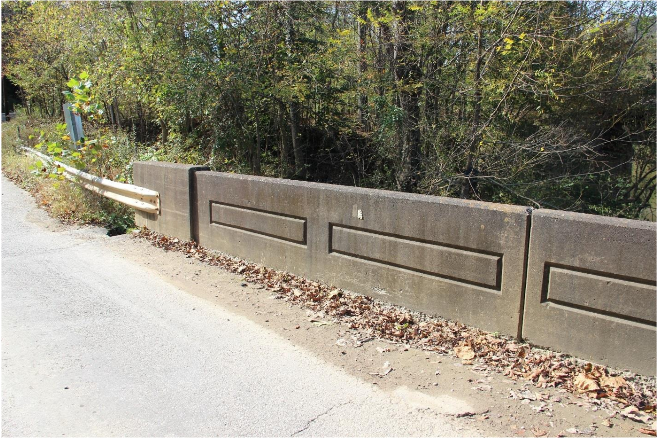
PHOTO 14 DETAIL OF SOUTHWEST PARAPET SHOWING PANELED PARAPET SECTIONS AND PLAIN END POST, FACING SOUTHWEST.
