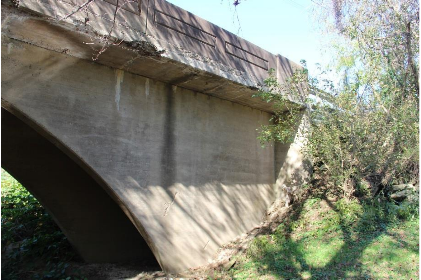
PHOTO 6 SOUTHEAST ELEVATION OF BRIDGE SHOWING DETAIL OF SPANDREL WALL AND NORTHEAST ABUTMENT, FACING NORTH.
