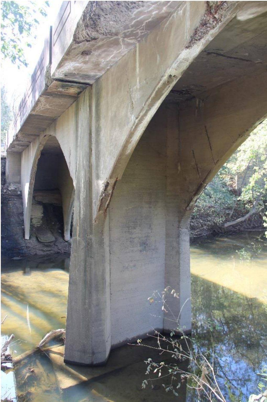
PHOTO 10 SOUTHEAST ELEVATION AND UNDERSIDE OF BRIDGE SHOWING DETAIL OF CENTER PIER AND CLOSED SPANDREL BRACED ARCHES, FACING SOUTHWEST.
