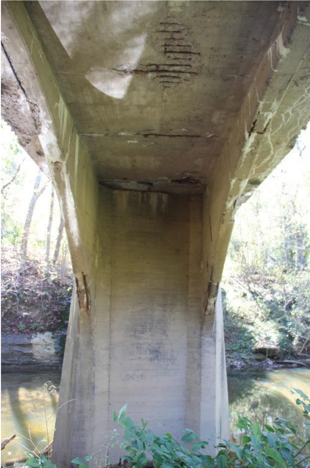
PHOTO 11 UNDERSIDE OF BRIDGE SHOWING DETAIL OF CENTER PIER AND CLOSED SPANDREL BRACED ARCHES FROM NORTHEAST ABUTMENT, FACING SOUTHWEST.
