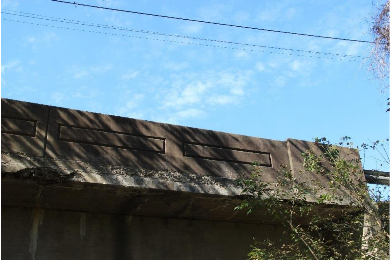
PHOTO 7 SOUTHEAST ELEVATION OF BRIDGE SHOWING DETAIL OF PANELED PARAPET AND CANTILEVERED DECK, FACING NORTHWEST.
