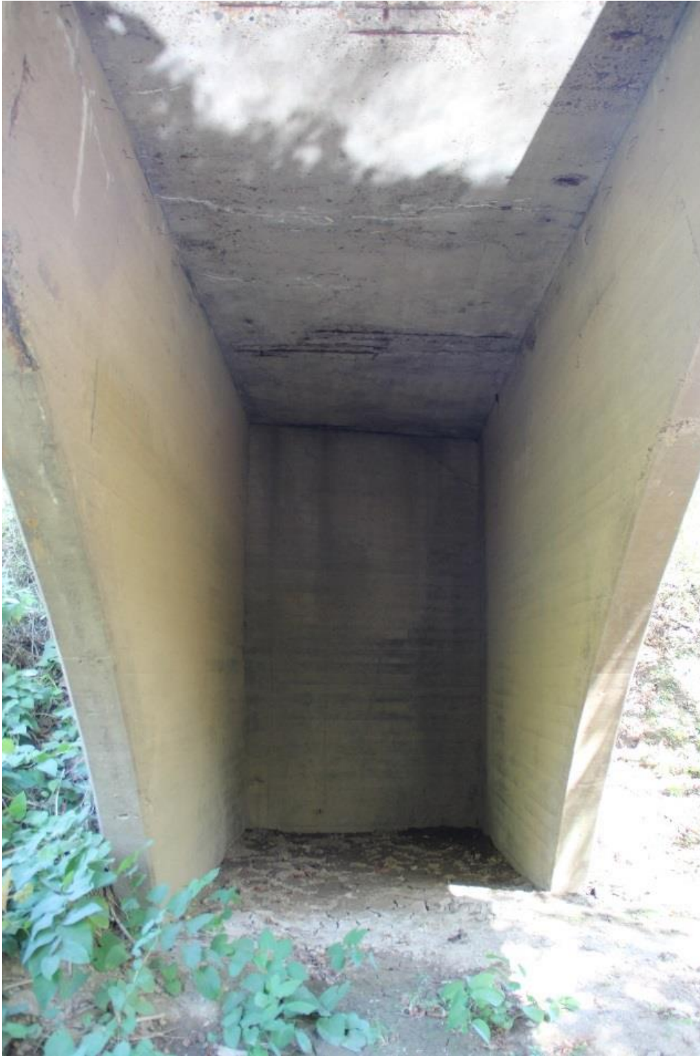
PHOTO 12 UNDERSIDE OF BRIDGE SHOWING DETAIL OF NORTHEAST ABUTMENT AND CLOSED SPANDREL BRACED ARCHES, FACING NORTHEAST.
