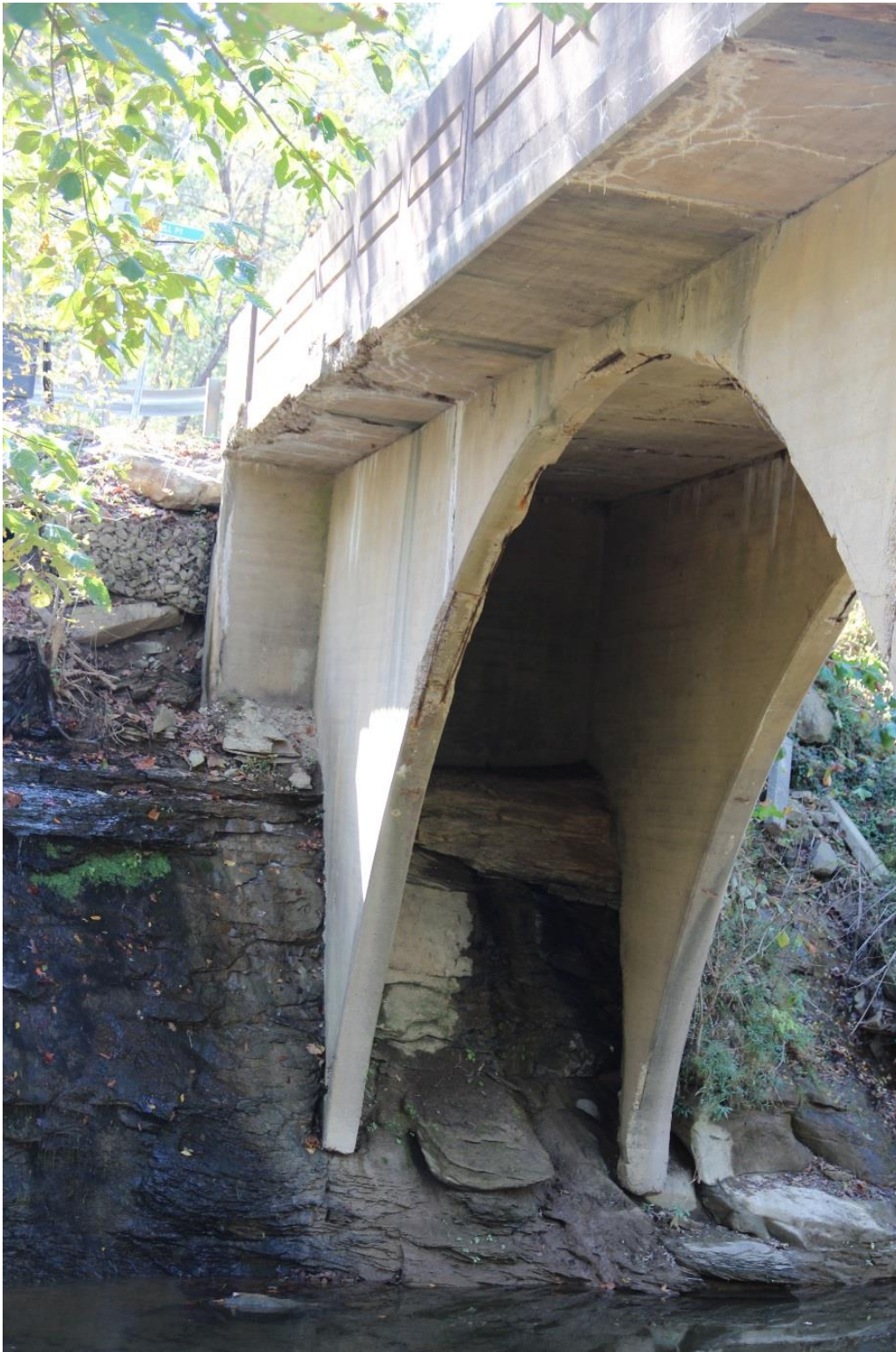
PHOTO 9 SOUTHEAST ELEVATION AND UNDERSIDE OF BRIDGE SHOWING DETAIL OF SOUTHWEST ABUTMENT, CANTILEVERED DECK, AND CLOSED SPANDREL BRACED ARCHES, FACING SOUTHWEST.
