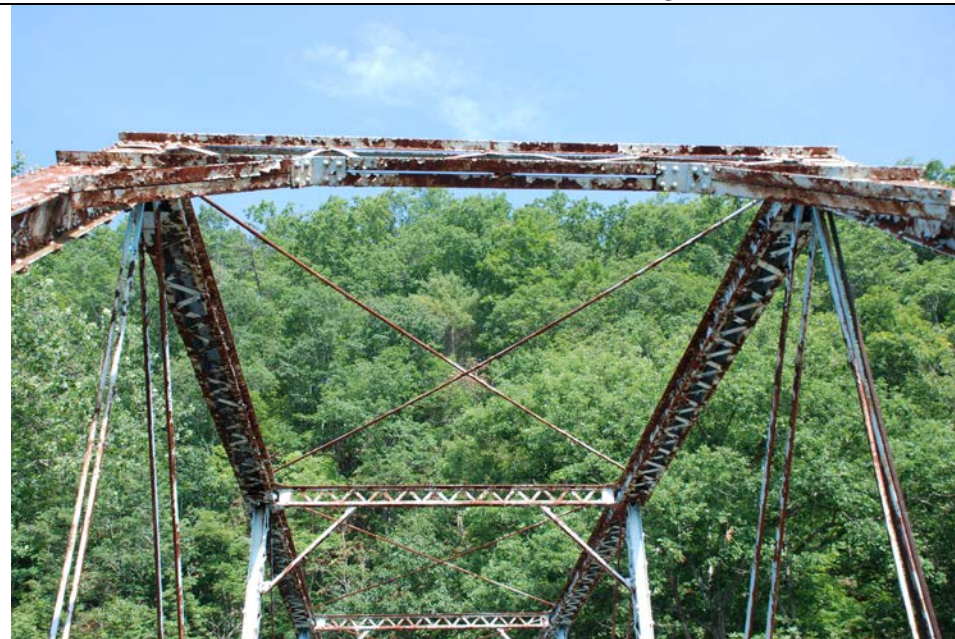
3. Overhead bracing
