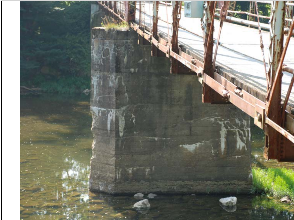
9. Center Pier and repaired lower eyebars
