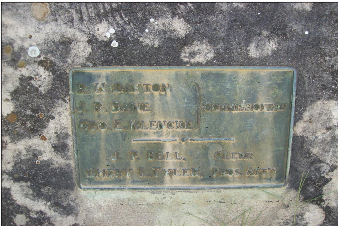
County commission plaque on downstream parapet.
