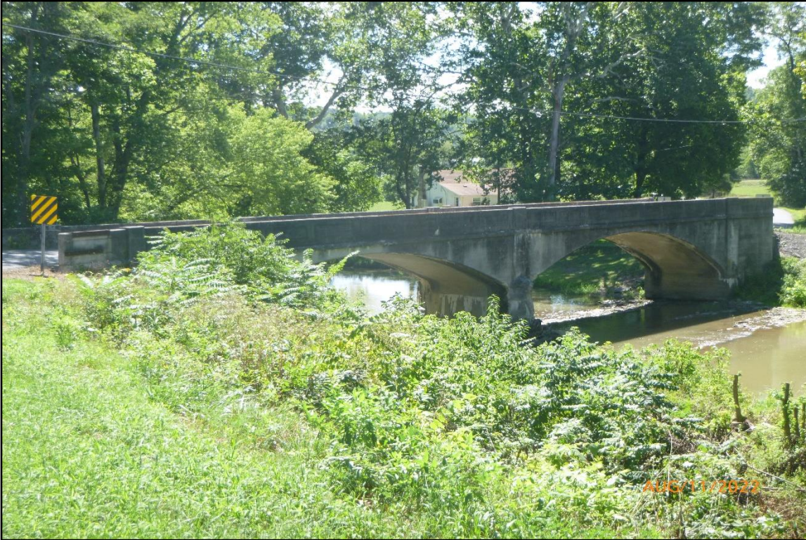
Upstream elevation of Charles Milar Bridge.
