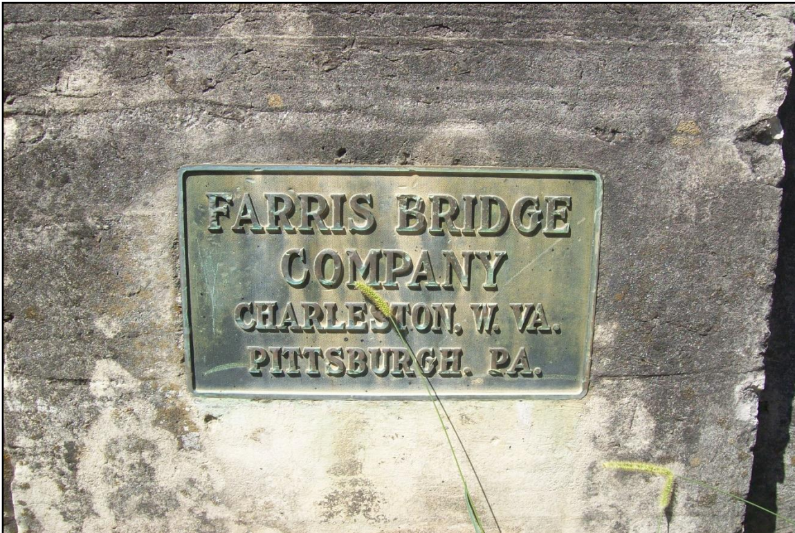
Construction plaque on upstream parapet.
