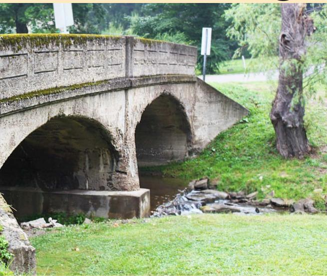
**Location:** County Route 1/7 at its intersection with County Route 1 Spanning Harmon Creek **Type:** Two Reinforced Concrete Arch Spans Supported by Two Stub Abutments and One Pier
