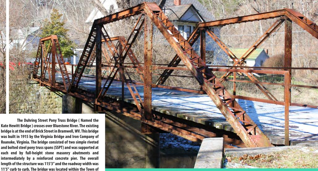
**Location:** Brick Street crossing over the Bluestone River **Type:** Two Simple Riveted and Bolted Steel Pony Truss Spans
