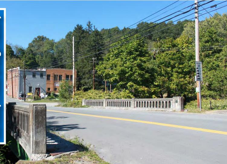
Location: Along WV Route 61 Alternate Type: Simple Span Wide Flange Beam with Concrete Abutments Year constructed: 1945 Length: 55 feet, 8 inches Contractor: Contractor is unknown
