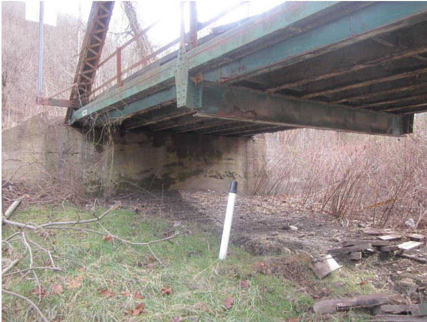
19. Looking toward East Abutment, Highlighting Truss/Bottom Chord/Floor Beam Gusset Connection, View Southeast
