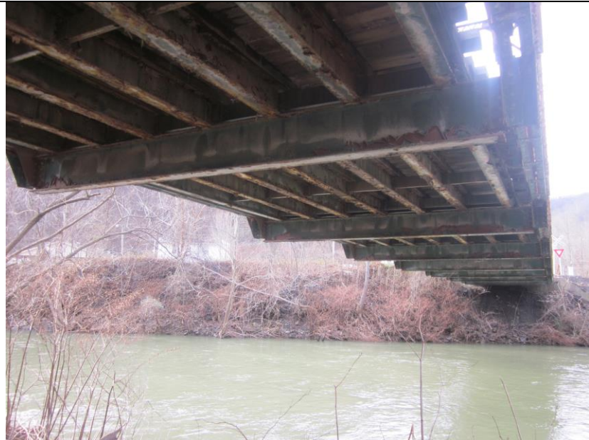
17. Underside of Bridge, View Southwest; Composed of steel floor beams, topped by steel stringers w. diaphragms (lateral bracing) between, top with wood nailing strips to which the wood deck boards are attached.
