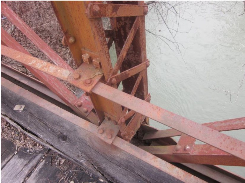
15. Detail – Main Vertical Post/Diagonal Bracing Connections to Lower Chord (So. Truss, 2nd Main Post from E. End), View SE; Post composed of two channels w/ Lattice bracing on both sides; Diagonal Bracing composed of two L-shapes.
