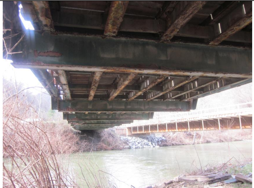
18. Underside of Bridge, View West/Southwest; Composed of steel floor beams, topped by steel stringers w. diaphragms (lateral bracing) between, top with wood nailing strips to which the wood deck boards are attached.
