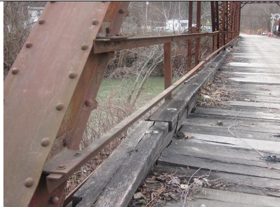
12. South Truss, Highlighting Railing and Curb, View Southwest
