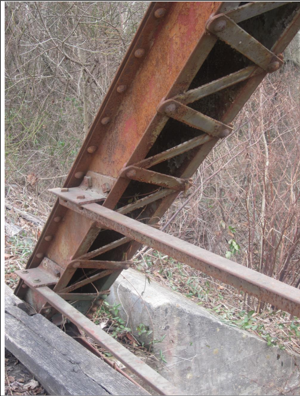
13. Detail – Lattice Bracing on Truss End Post (South Truss, East End), View SE; End post composed of two steel channels, steel plate on outward side and lattice bracing at underside.
