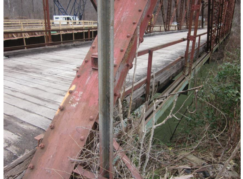
16. South Truss Showing Lower Chord (part that the vertical posts and diagonal bracing area gusseted to), View Northeast; Lower Chord composed of two original steel L-shapes, each topped by a steel L-shape installed in 1993.
