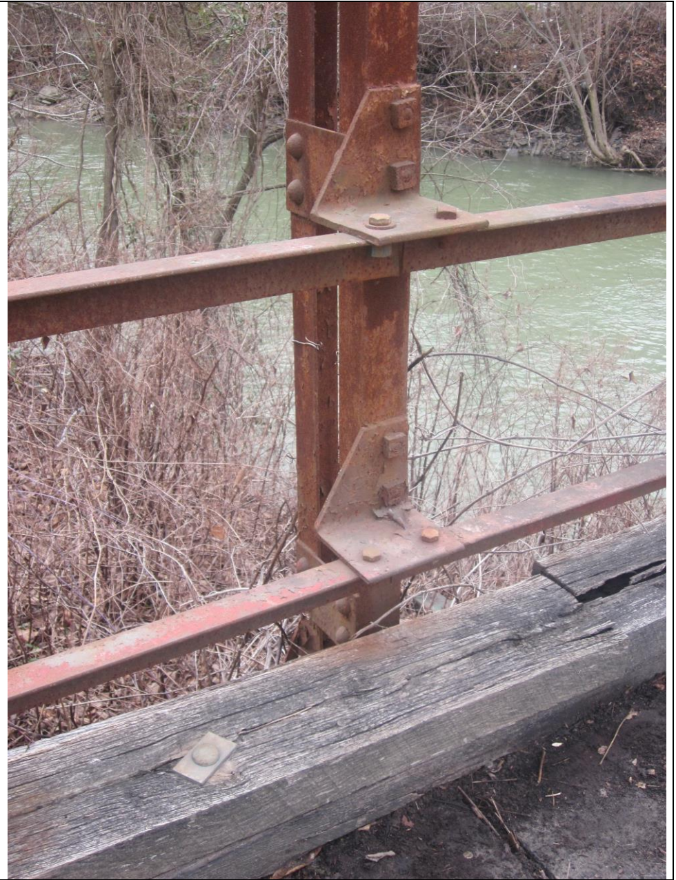
14. Detail – Connection of Railings at Vertical Hip Post (South Truss, East End Vertical), View Northeast; Post composed of two steel L-shapes
