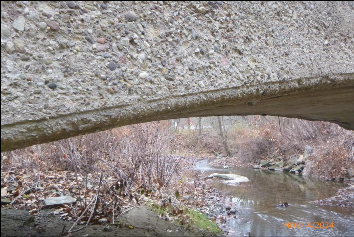
Detail of rounded arch ring feature.
