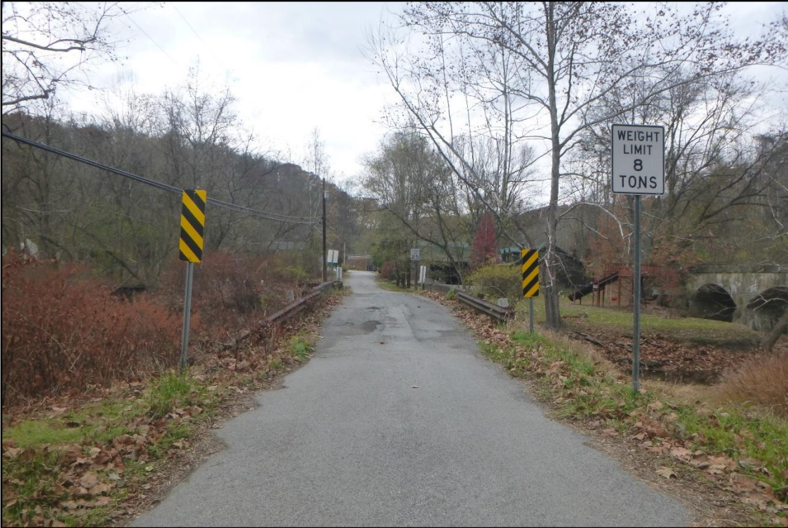
South approach to Log Cabin Bridge.
