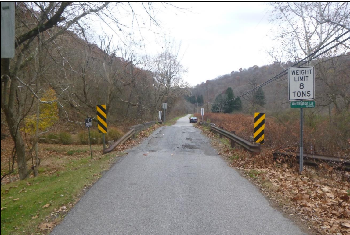
North Approach to Log Cabin Bridge.
