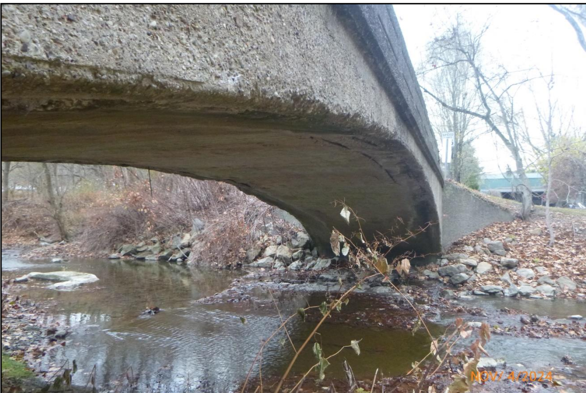
Detail of superstructure and reinforced concrete tie in streambed.
