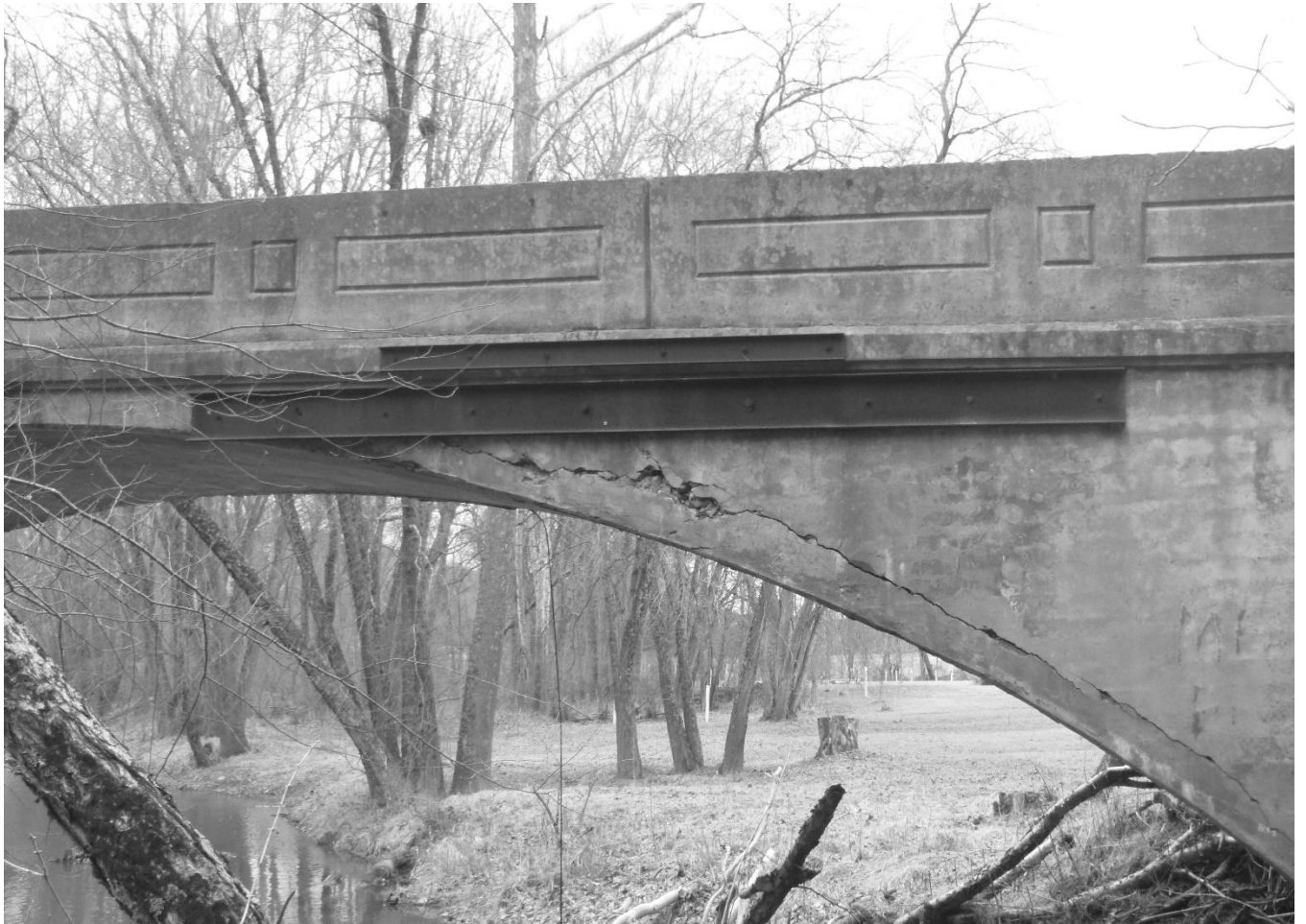
Photo 12 New Hope Bridge Morgan County County Route 8/1 spanning Sleepy Creek Repair to west end of downstream spandrel
