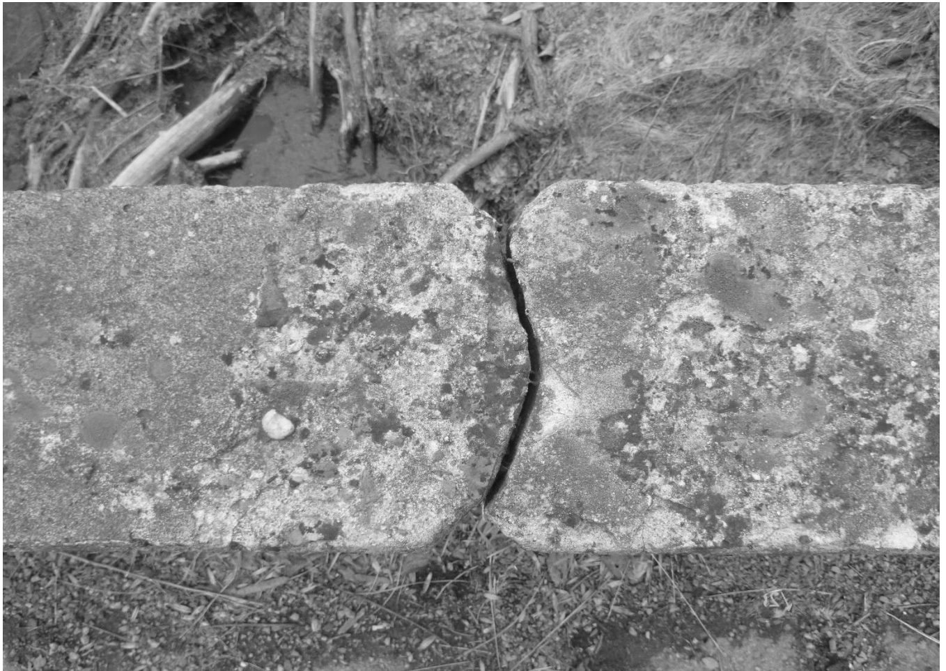
Photo 10 New Hope Bridge Morgan County County Route 8/1 spanning Sleepy Creek Detail of parapet connection
