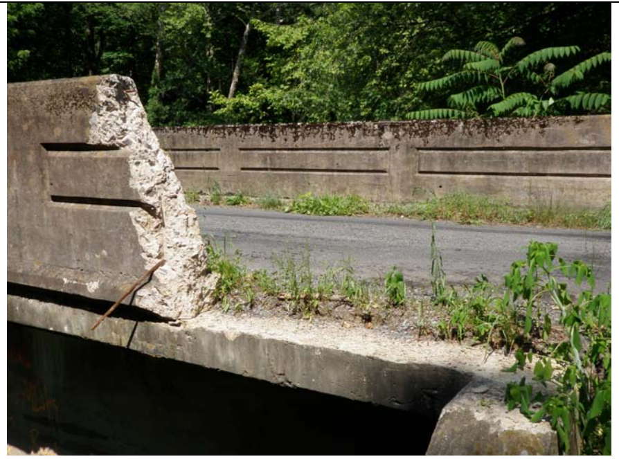
12. Missing parapet wall at abutment #2
