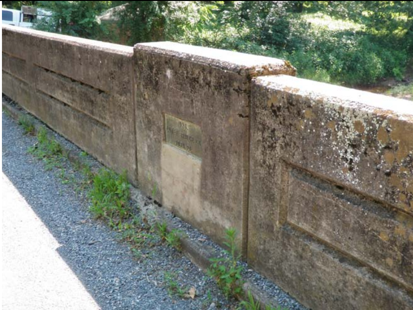
9. Parapet wall with bridge builder plate in place
