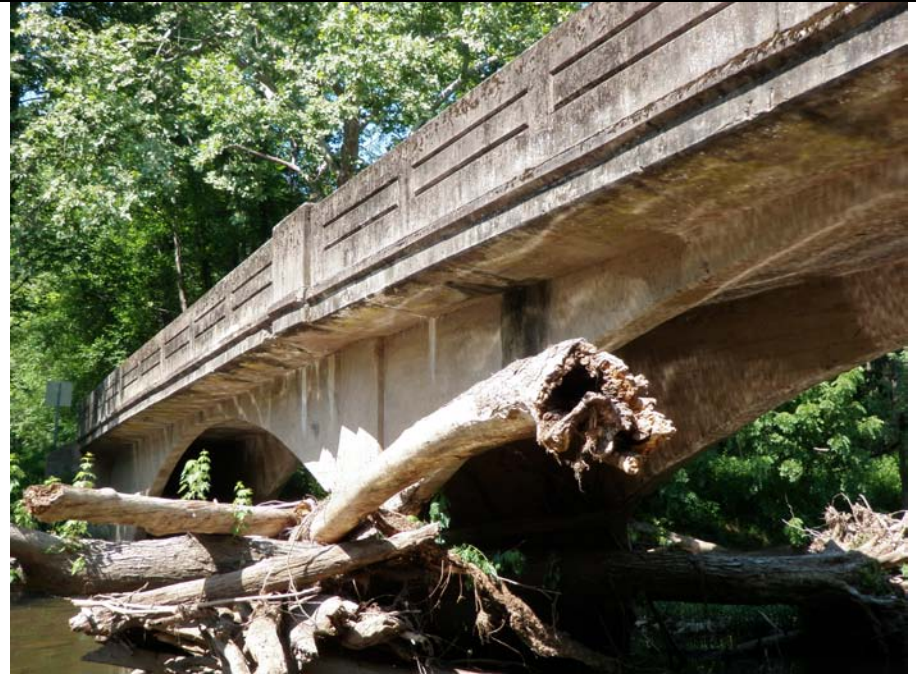
2. Large dead trees lodged against the upstream end of the pier
