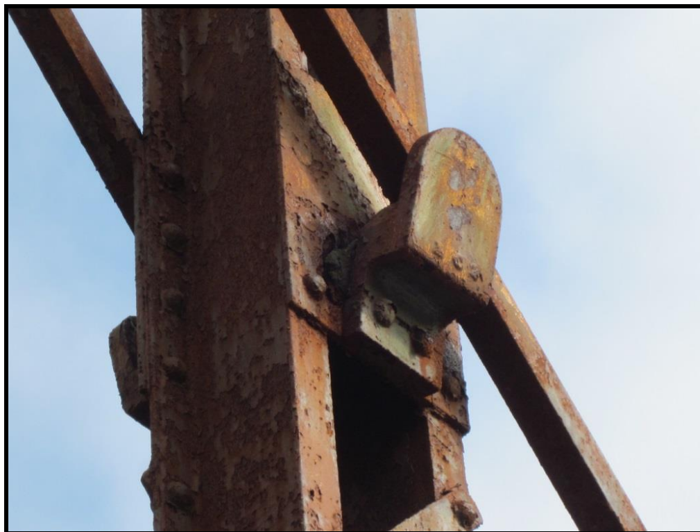
Typical Detail of a main vertical Post with retainer clps that attached to the hold the diagonal tension members in place (WVDOH Feb. 2, 2015).
