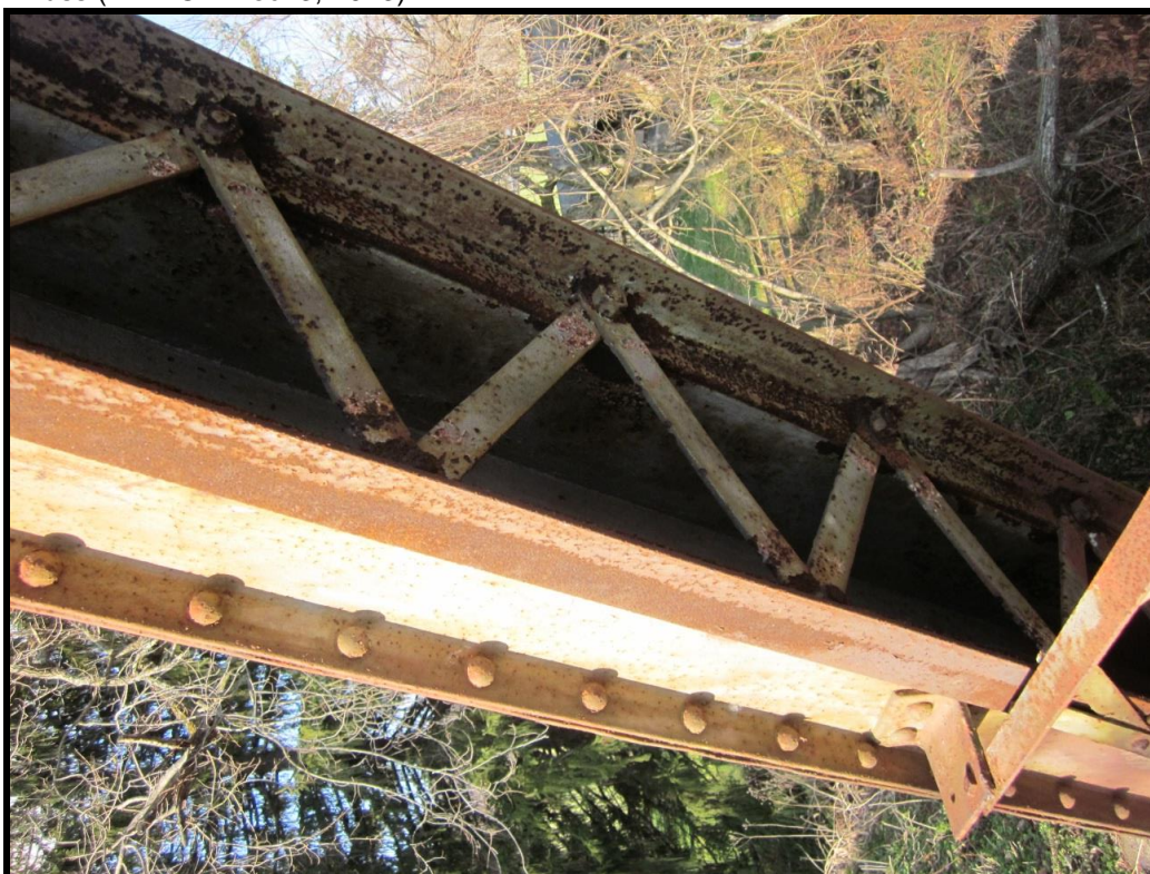
Typical Endpost Detail. View Northwest of North (Upstream Side) Truss, West Endpost (WVDOH Dec. 3, 2013).
