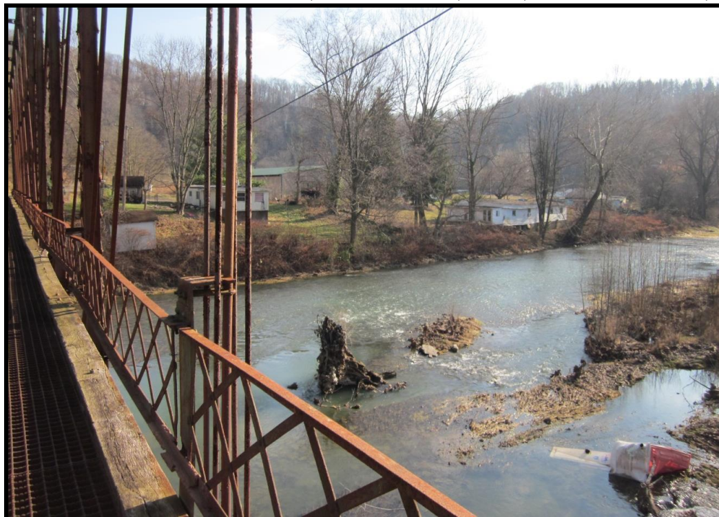
Detail View Highlighting the Hip Vertical Tension Member at the South Truss, West End. This member includes the original thicker diameter central eyebar with four later-added (1975) loop bar hangers around it. View SE (WVDOH Dec. 3, 2013).
