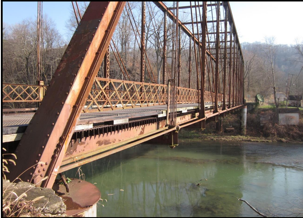
Detail View of Typical Truss Members, incl. Endpost, Lower Chord Eyebars, and Hip & Main Tension Verticals. View East of South (Downstream Side) Truss (WVDOH Dec. 3, 2013)
