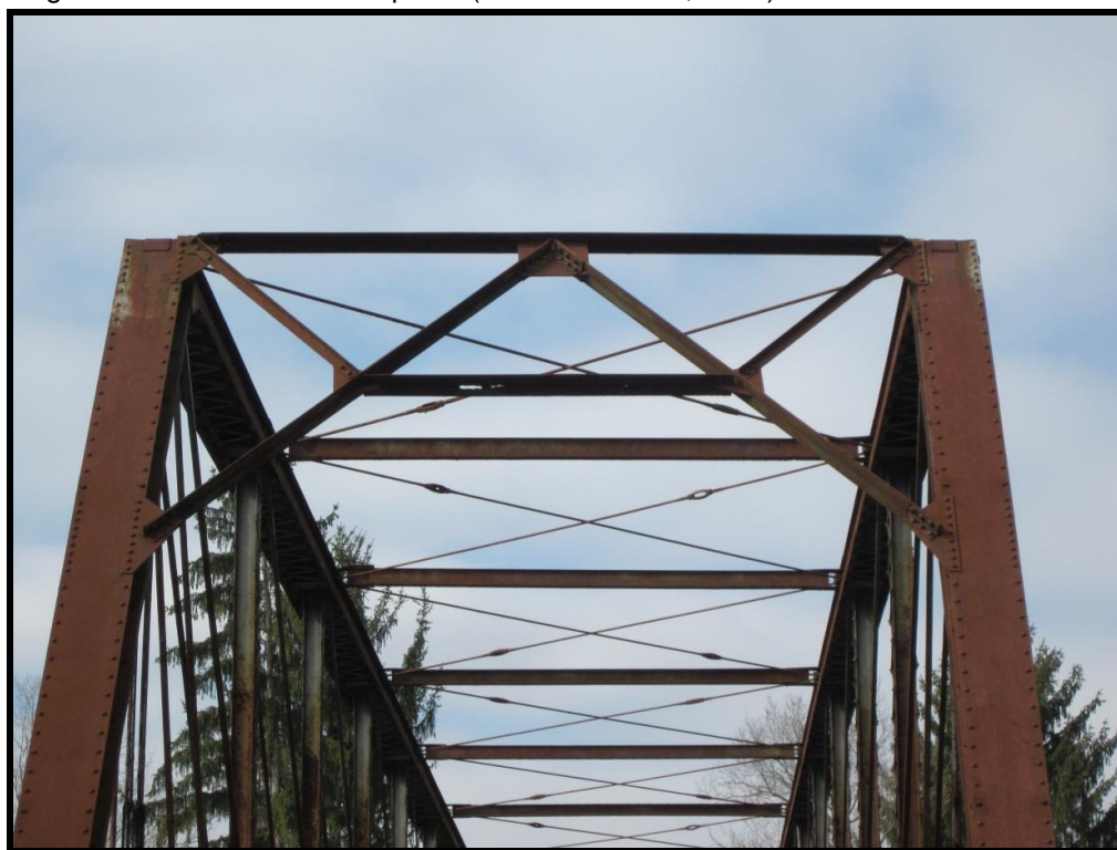
East end of bridge, Highlighting the typical Portal Strut/Bracing between Endposts, Sway Struts, and Top Lateral Bracing (crossed eyebars). View NE (WVDOH 2-10-2015)
