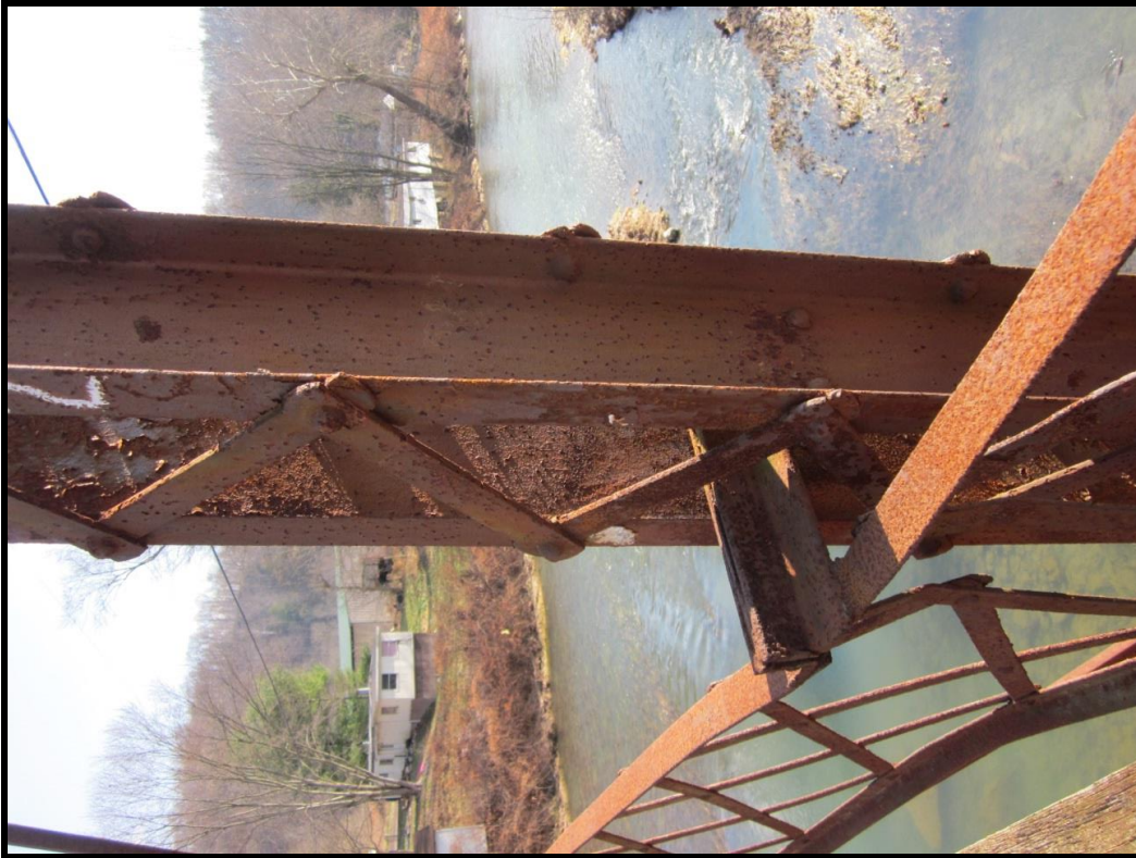
Typical Main Vertical Tension Member Detail. View Southeast of South (Downstream Side) Truss (WVDOH Dec. 3, 2013)
