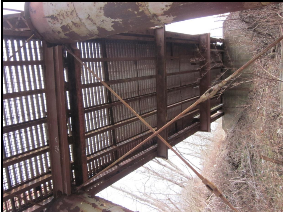
Deck Girder Span, Highlighting the understructure of Girders, Floorbeams and Stringers. East end Caisson Bent/Pier (with eyebar tension members in foreground) View SE (WVDOH Feb 10, 2015)
