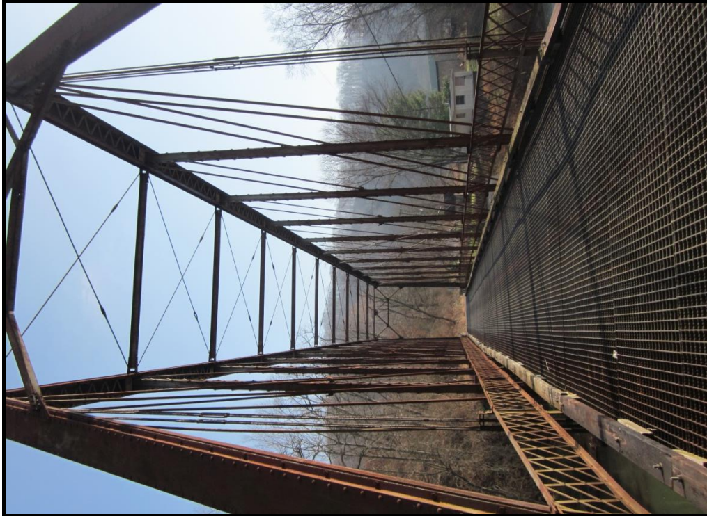
Interior of Bridge, Highlighting Sway Struts & Top Lateral Bracing (crossed eyebars) and extant steel grid decking (replaced timber decking in 1988). View SE (WVDOH Dec. 3, 2013)
