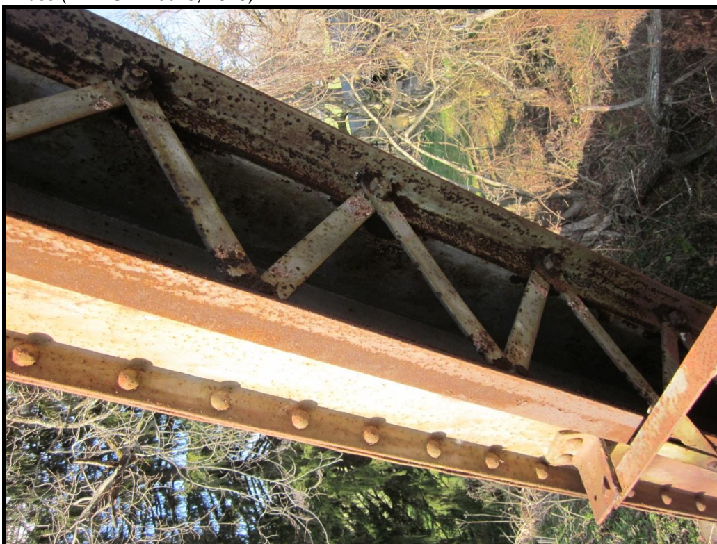
Typical Endpost Detail. View Northwest of North (Upstream Side) Truss, West Endpost (WVDOH Dec. 3, 2013).
