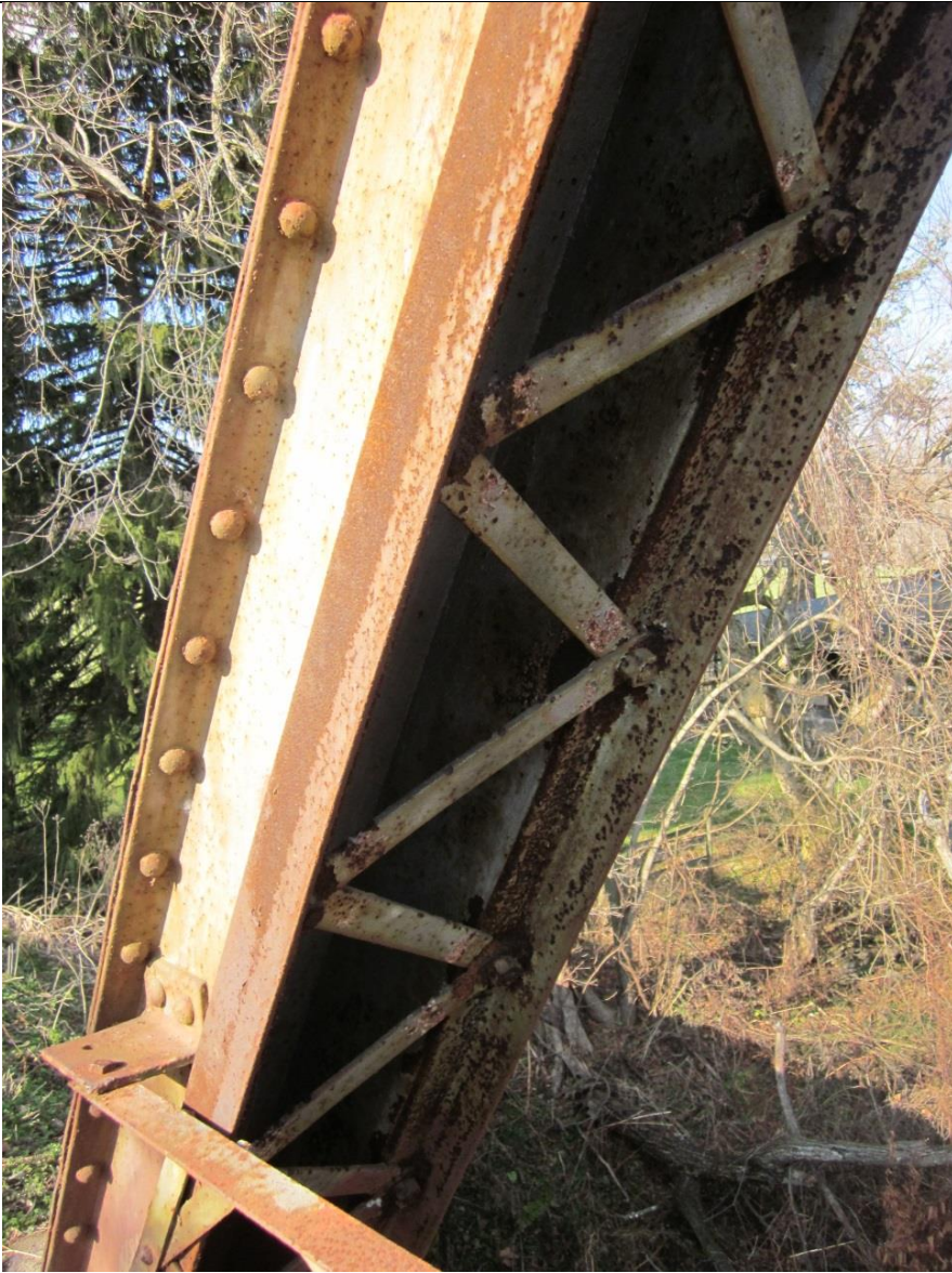
11. Typical End Post Detail. View Northwest of North Side Truss
