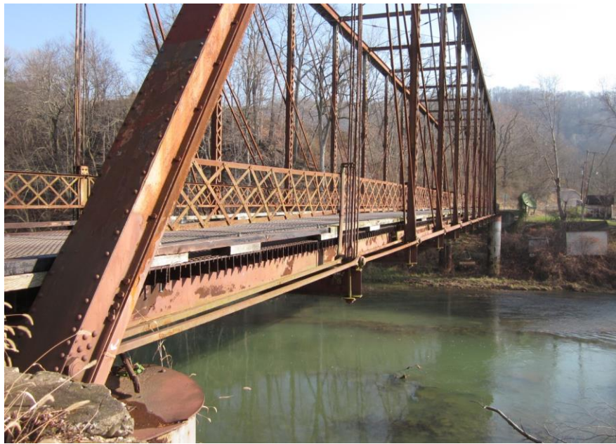
9. South Truss. Detail View of Typical Truss Members, incl. End Post, Lower Chord Eyebars, and Hip and Main Tension Verticals. View East
