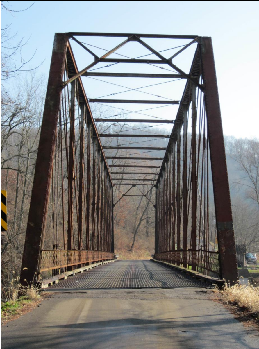
5. West End. View Southeast. Note Portal Strut/Bracing between End Posts
