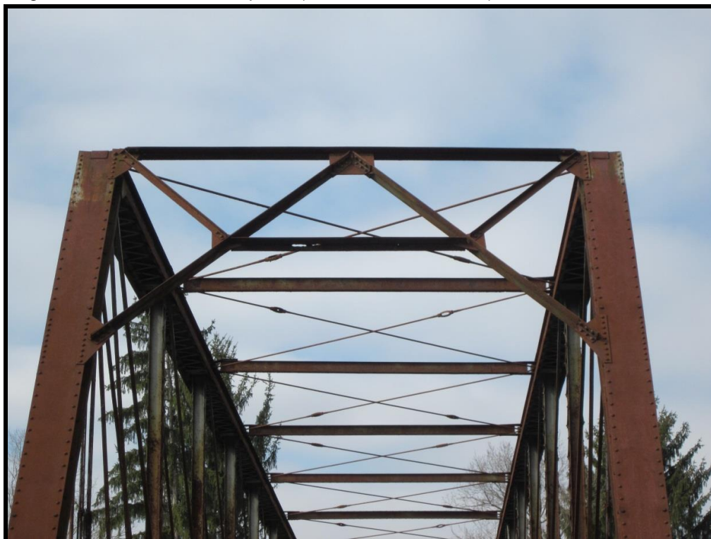
East end of bridge, Highlighting the typical Portal Strut/Bracing between Endposts, Sway Struts, and Top Lateral Bracing (crossed eyebars). View NE (WVDOH 2-10-2015)
