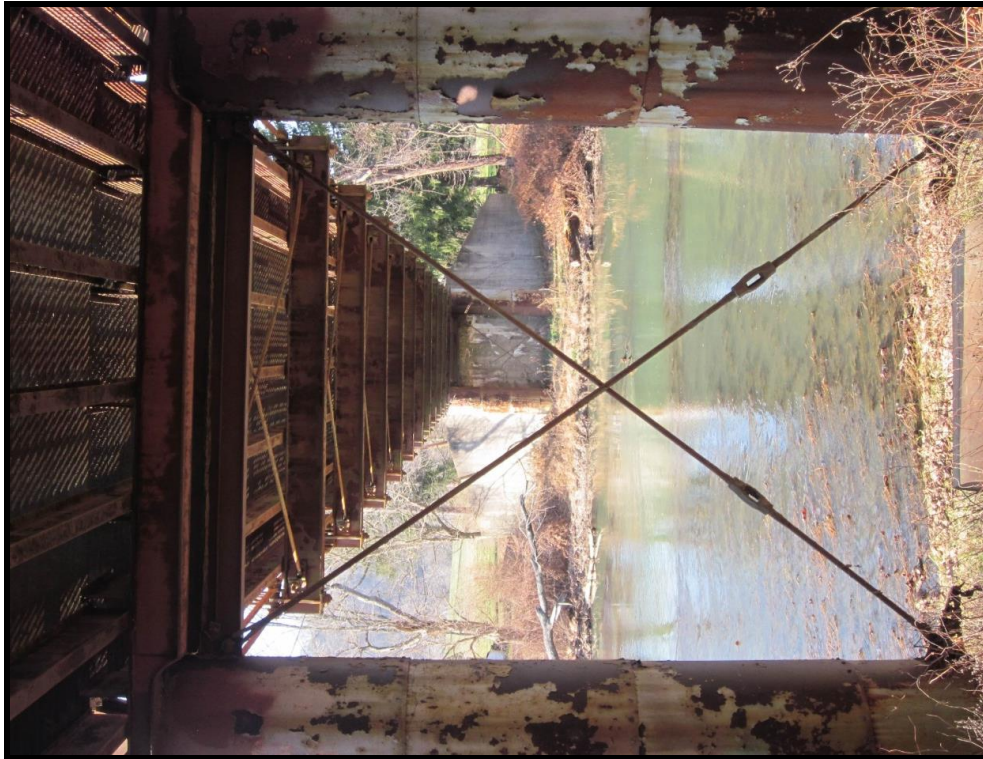
Underside of Truss Deck, Highlighting Floorbeams, Stringers and lateral bracing. View NW (WVDOH Dec. 3, 2013). East end caisson bent/pier (with eyebar tension members) is in foreground.
