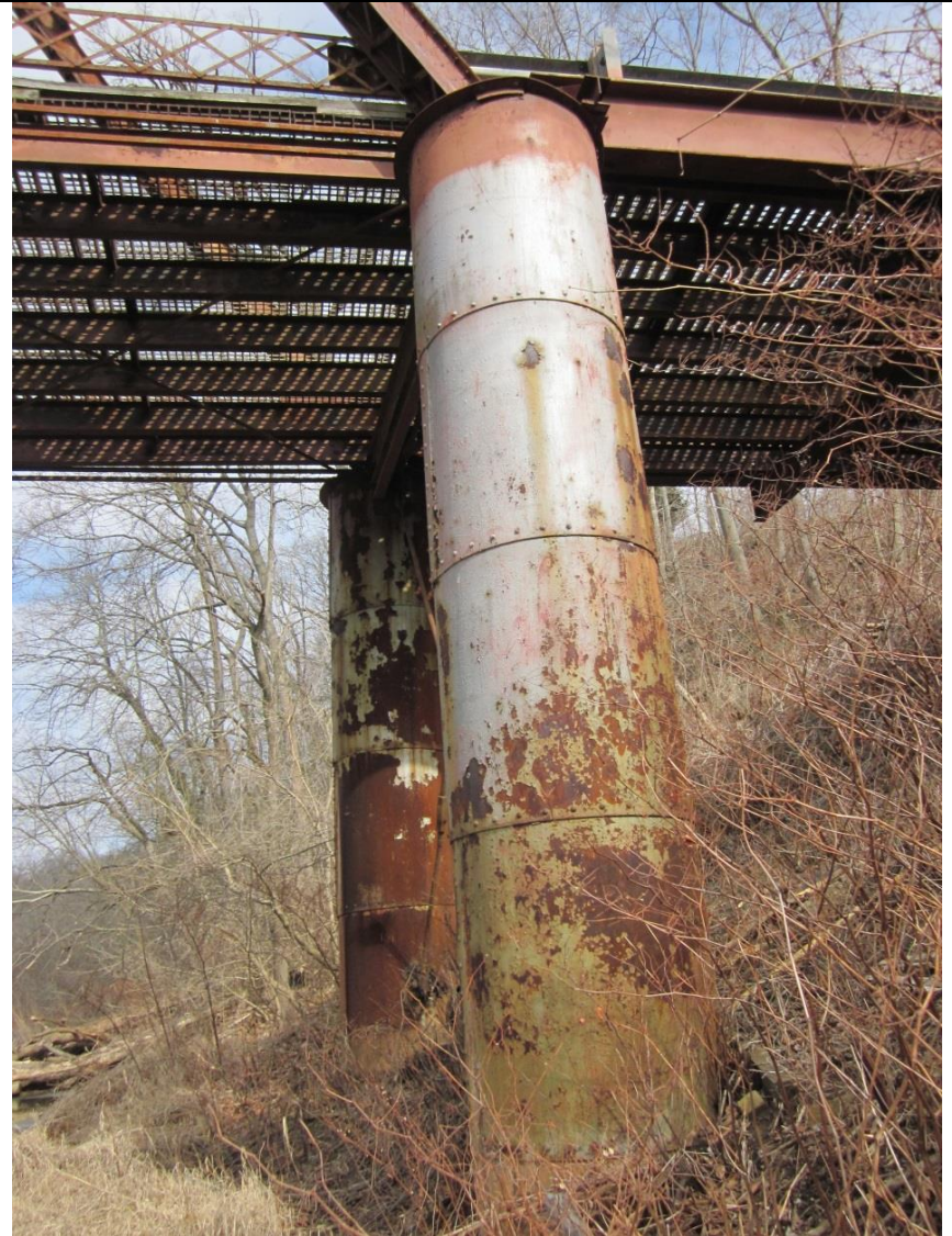
20. East End Caisson Bent. View North/Northeast
