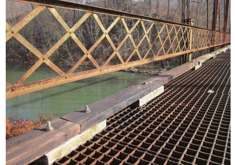
10. Typical Railing and Curb Detail. View East of North Side Truss
