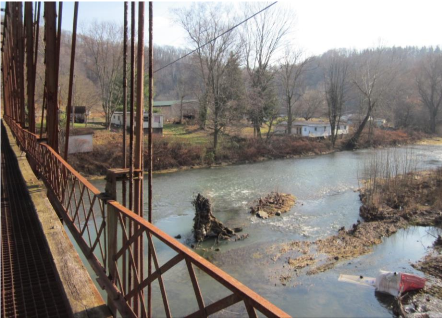
13. Detail View Highlighting the Hip Vertical Tension Member at the South Side Truss, West End. View Southeast
