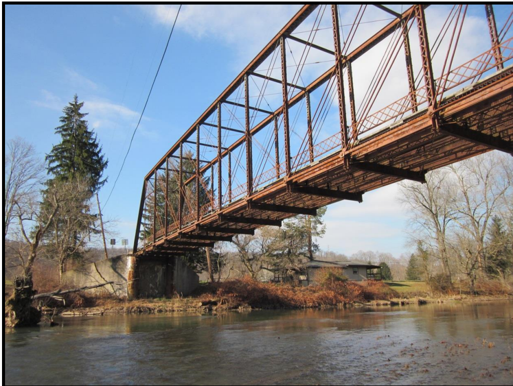
South (Downstream Side) Elevation, Highlighting Floorbeams between trusses. West pier/abutment is also in view. View Northwest (WVDOH Dec. 3, 2013).
