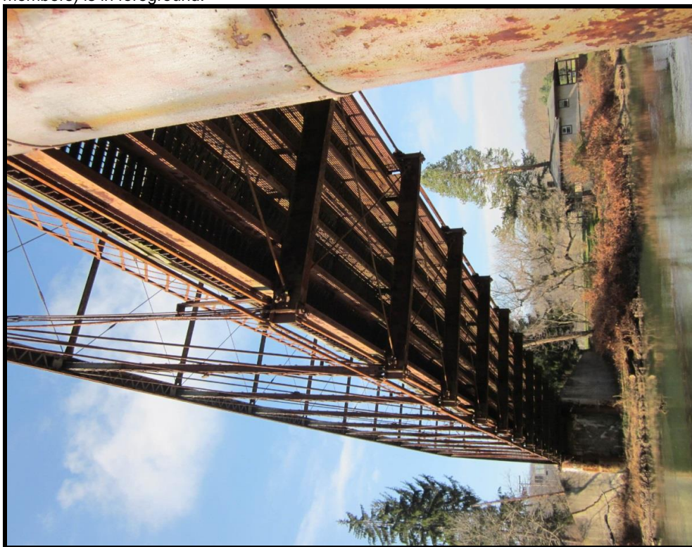
Underside of Truss Deck , Highlighting the floorbeams, stringer and lateral bracing. View NW (WVDOH Dec. 3, 2013).
