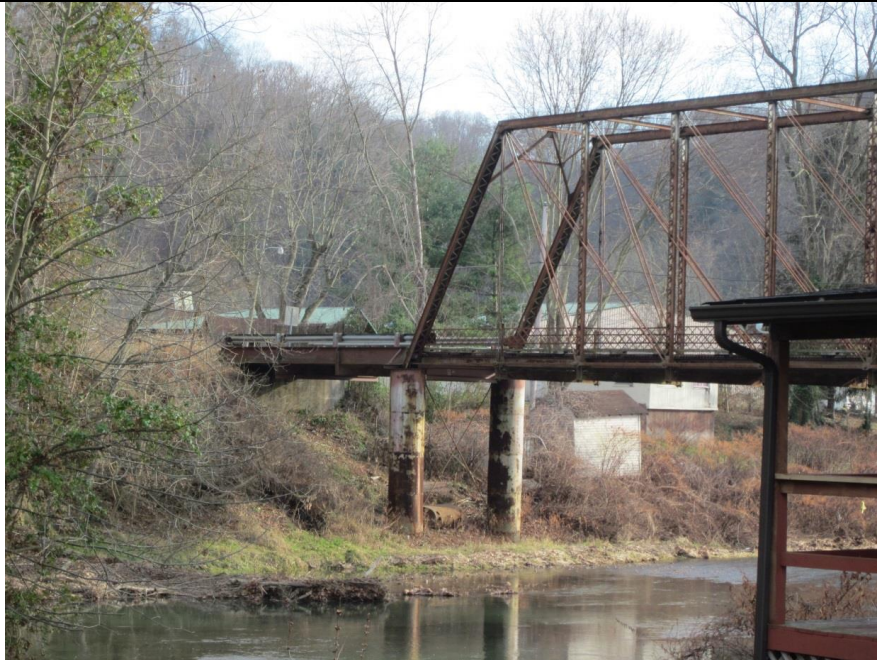
15. Caisson Bent at East End of Bridge. View Southeast
