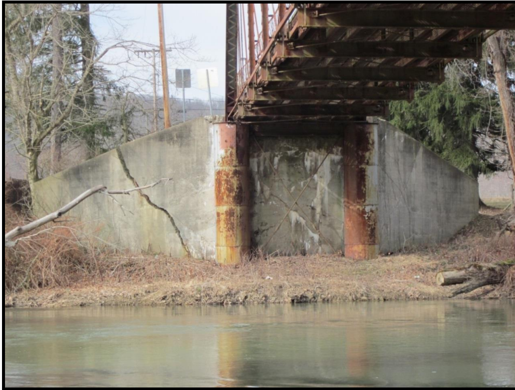
APE B1 - Rude Bridge. Caisson Bent & Abutment at West End of Bridge. View Northwest (WVDOH Feb. 10, 2015). Note cracks in abutment/wingwalls.
