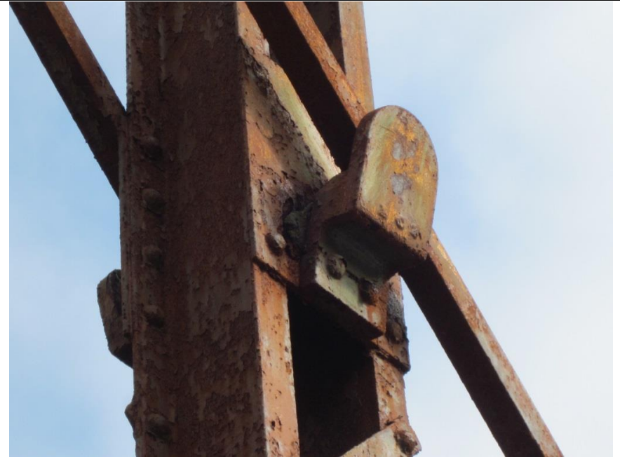
14. Typical Detail of a Main Vertical Tension Post with Retainer Clips for attachment of Diagonal Tension members.
