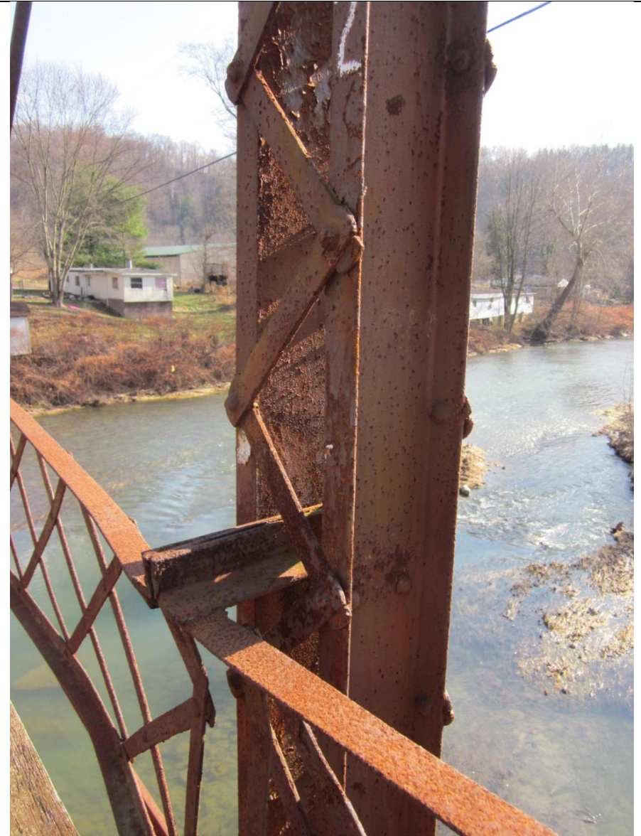
12. Typical Main Vertical Tension Member. View Southeast of South Side Truss
