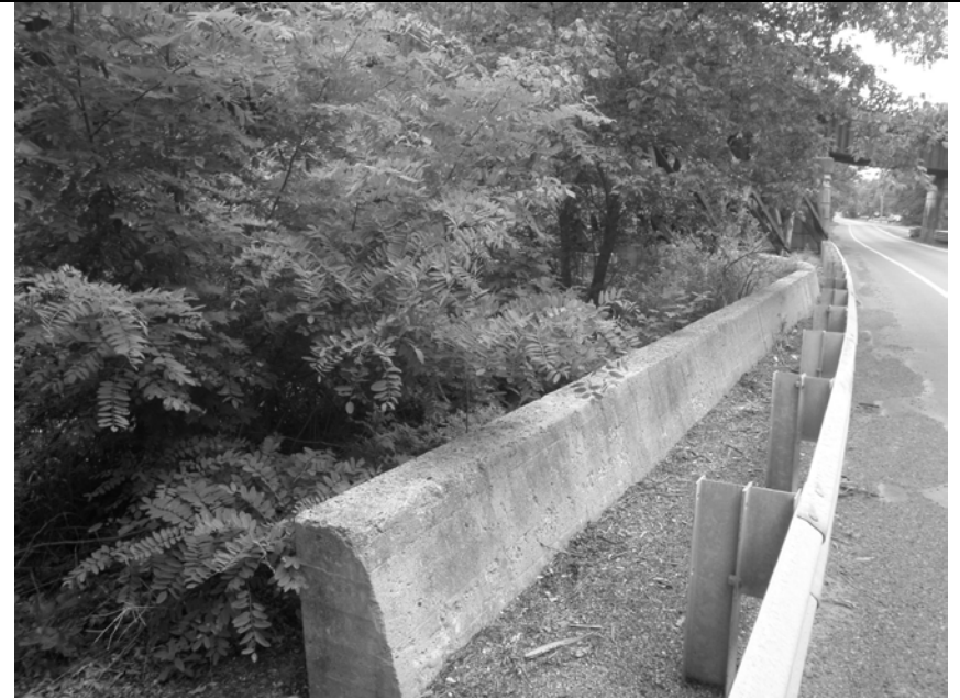
Photo 2- Concrete wall used as a pier
