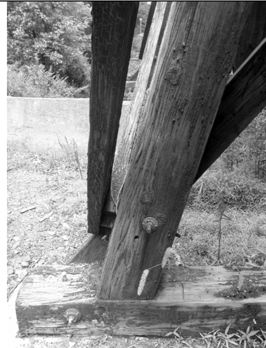
Photo 4- Bolt connections at footer
