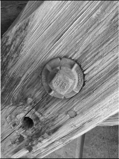
Photo 12- Bolt connection
