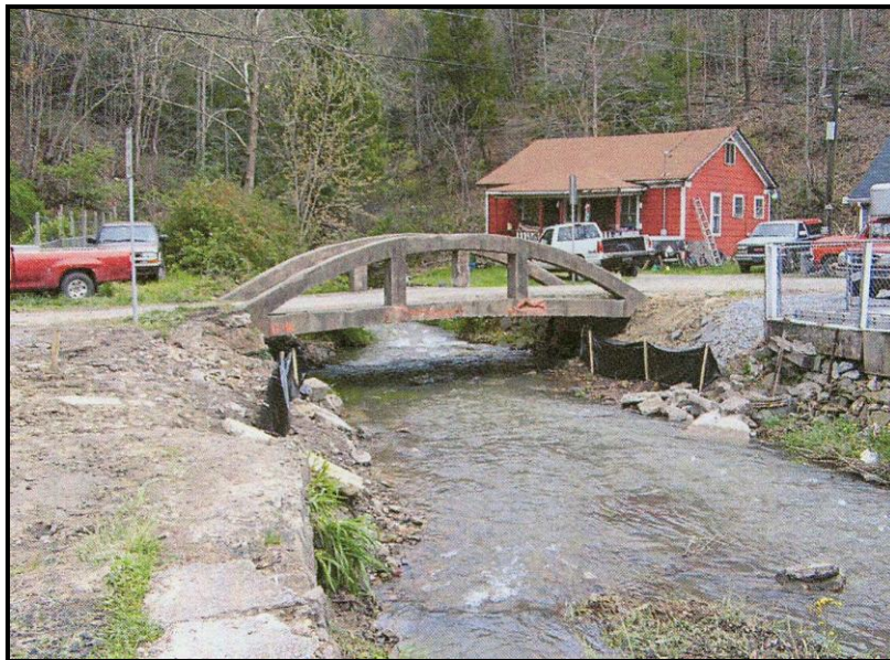
Figure 49. Wyco Hollow Arch Bridge (Bridge 55-012/01-001.10) in Wyoming County, constructed in 1920, illustrating a concrete through arch bridge (photograph courtesy of West Virginia Division of Highways)
