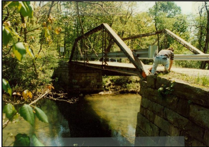
Figure 29. West Clifton Mills Bridge (Bridge 39-004/02-001.71) in Preston County, constructed in 1893, illustrating a steel pony truss bridge (photograph courtesy of West Virginia Division of Highways)
