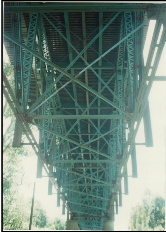
Figure 30. Gypsy Bridge (Bridge 17-019/00-023.26) in Harrison County, constructed in 1922, illustrating a steel deck truss bridge (photograph courtesy of West Virginia Division of Highways)
