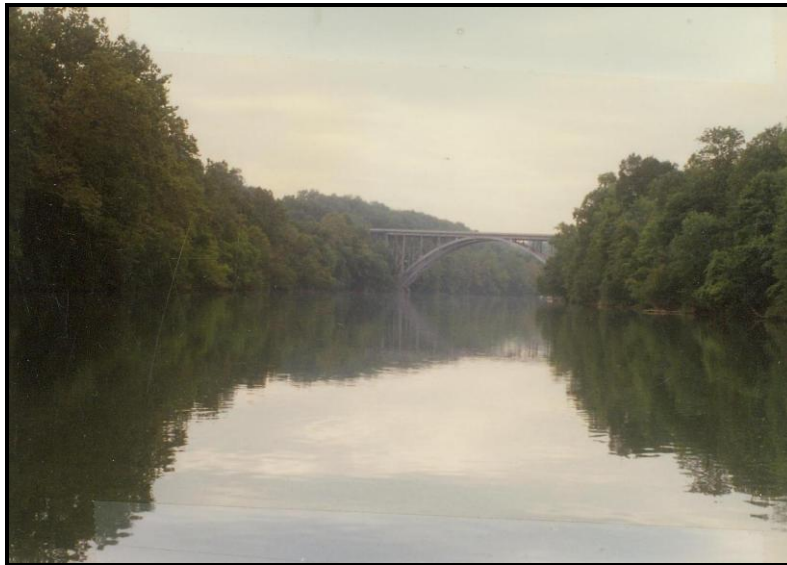
Figure 37. William Lee Prunty Bridge/Bentons Ferry Bridge (Bridge 25-079/00-132.84) in Marion County, constructed in 1960, illustrating a steel deck arch bridge (photograph courtesy of West Virginia Division of Highways)
