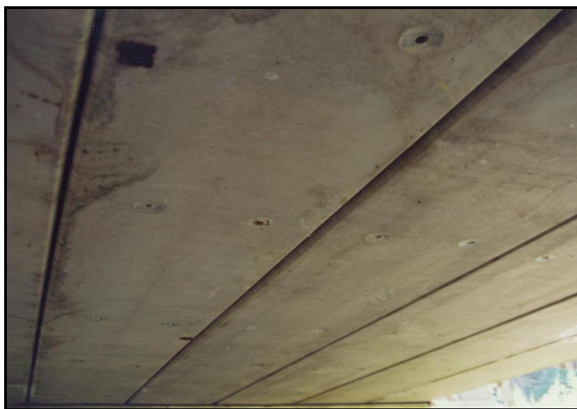
Figure 52. Kanawha Fork Road Bridge (Bridge 20-023/00-004.90) in Kanawha County, constructed in 1958, illustrating the underside of a prestressed concrete box beam bridge (photograph courtesy of West Virginia Division of Highways)
