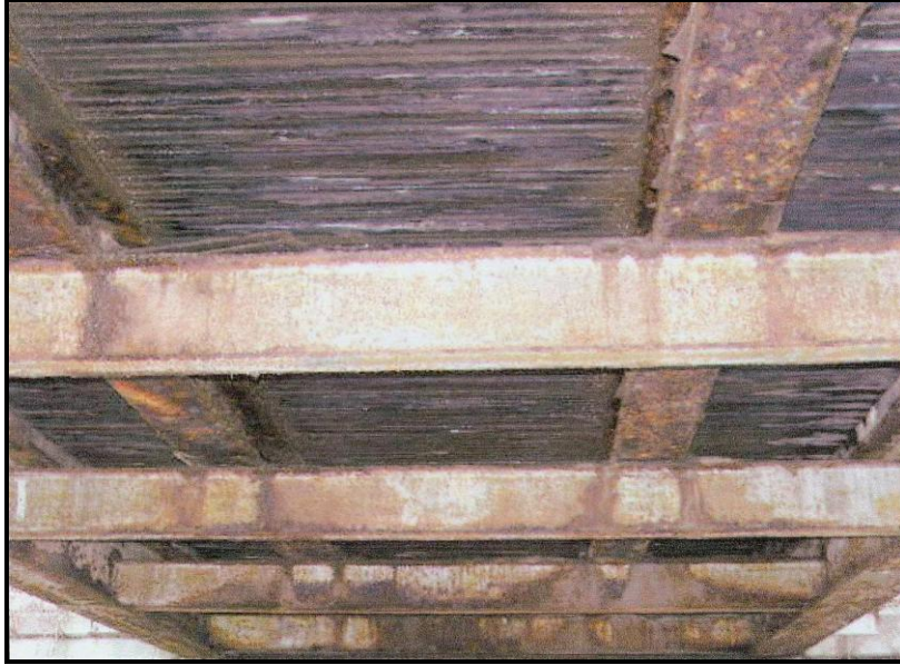
Figure 33. Joes Creek Bridge Number 0.01 (Bridge 03-003/05-000.01) illustrating flooring system (photograph courtesy of West Virginia Division of Highways)
