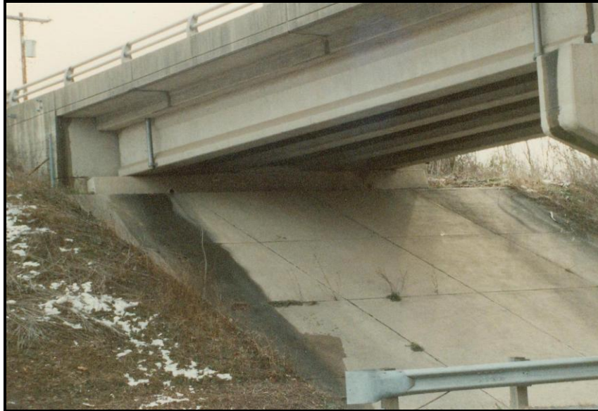
Figure 43. Broad Lane Overpass (Bridge 02-011/02-001.15) in Berkeley County, constructed in 1964, illustrating a prestressed concrete stringer bridge (photograph courtesy of West Virginia Division of Highways)
