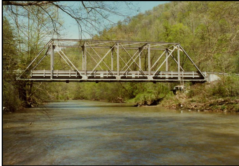
Figure 26. Gallagher Bridge (Bridge 20-083/03-001.06) in Monroe County, constructed in 1921, illustrating a steel through truss bridge (photograph courtesy of West Virginia Division of Highways)
