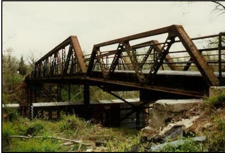
Figure 27. Grade Road Overpass (Bridge 02-001/00-001.57) in Berkeley County, constructed in 1900 illustrating a wrought iron pony truss bridge (photograph courtesy of West Virginia Division of Highways)
