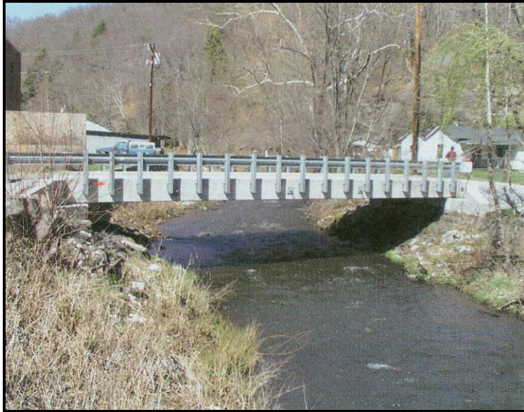
Figure 53. Pines Creek Bridge (Bridge 41-033/00-006.50) in Raleigh County, constructed in 1963, illustrating a prestressed concrete box beam bridge (photograph courtesy of West Virginia Division of Highways)
