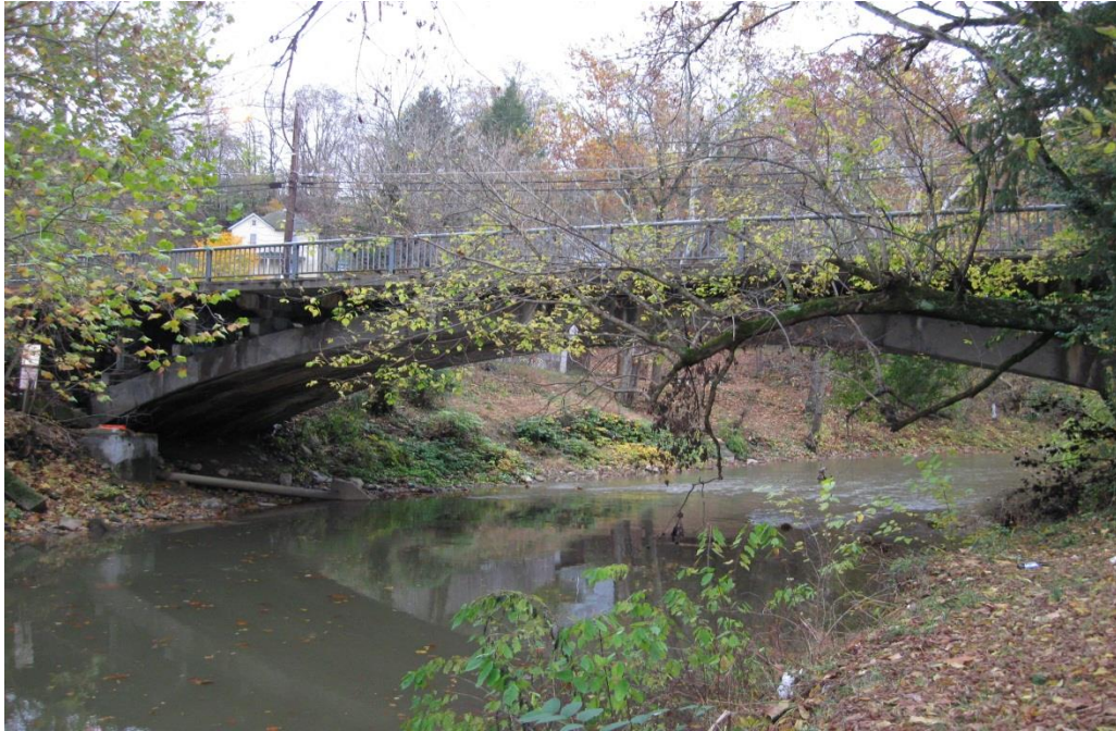
Photograph 2: Example of an open spandrel bridge with elliptical arch. (BARS #17A908, District 4, Harrison County)
