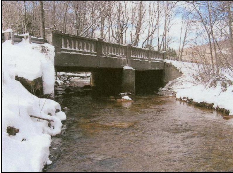
Figure 44. Birds Creek Bridge (Bridge 39-092/00-011.80) in Preston County, constructed in 1940, illustrating a concrete slab bridge (photograph courtesy of West Virginia Division of Highways)
