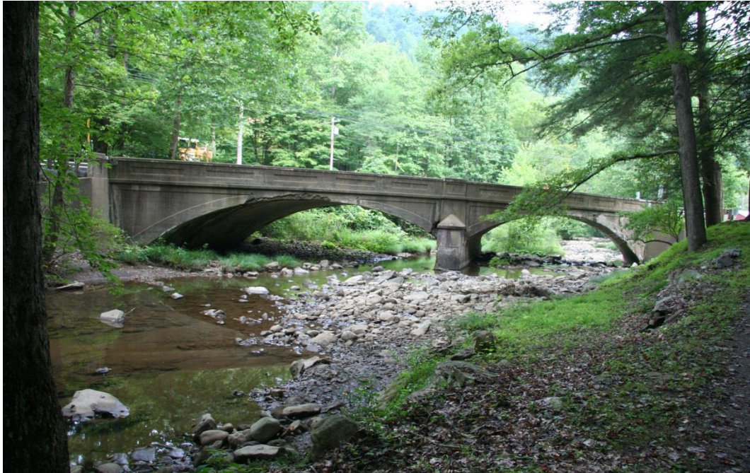
Photograph 6: Example of reinforced concrete arch with a nonsymmetrical arch design whereby the two arches are balanced against one another on the pier. (BARS #51A039, District 7, Webster County)
