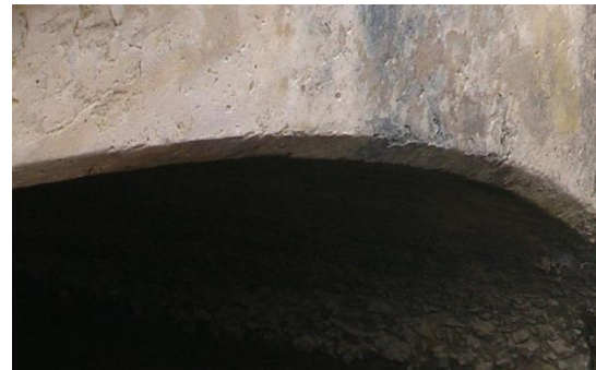
Photograph 5: Example of more typical bevel or flat edge not exclusive to Daniel Luten. (BARS #46A011, District 4, Taylor County)
