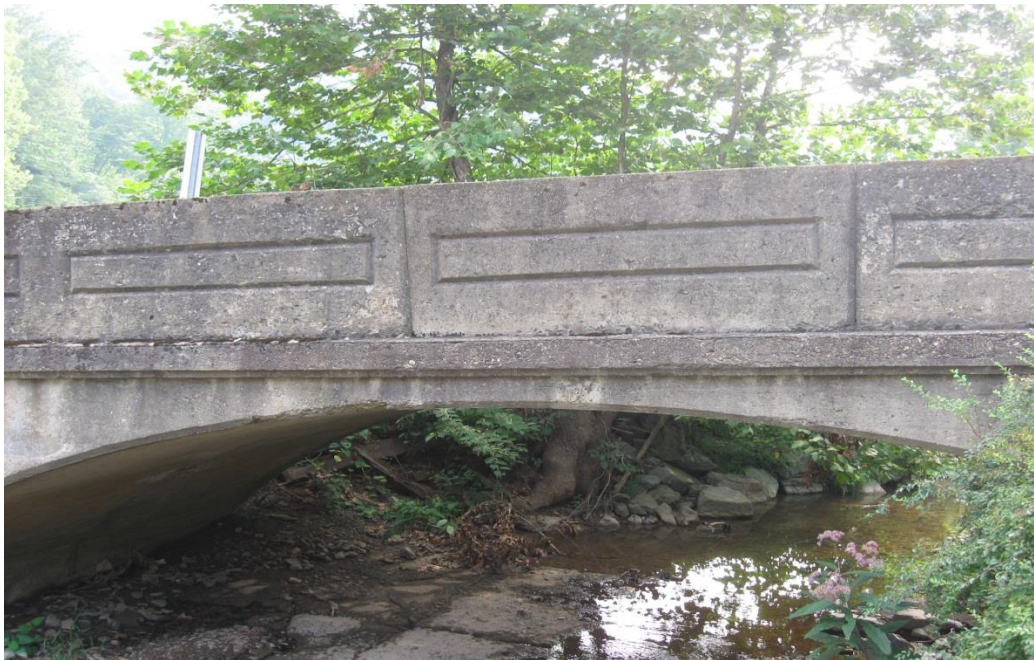
Photograph 3: Example of a tied arch. The concrete visible in the streambed is part of the bridge design and enables the arch to be unusually thin by providing additional reinforcement in conjunction with reinforcement in the arch ring and abutments. (BARS #52A072, District 6, Wetzel County)
