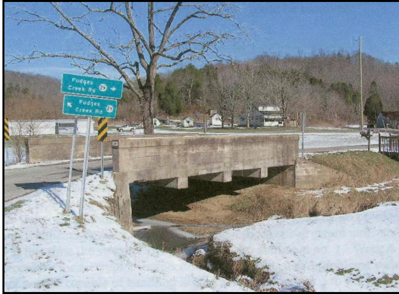
Figure 54. Prairietown Bridge (Bridge 06-029/00-001.68) in Cabell County, constructed in 1926, illustrating concrete girder/floorbeam bridge (photograph courtesy of West Virginia Division of Highways)
