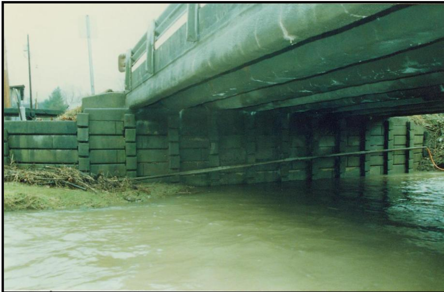
Figure 60. Copen Channel Bridge (Bridge 04-002/02-002.94) in Braxton County, constructed in 1950, illustrating a prestressed concrete channel bridge (photograph courtesy West Virginia Division of Highways)
