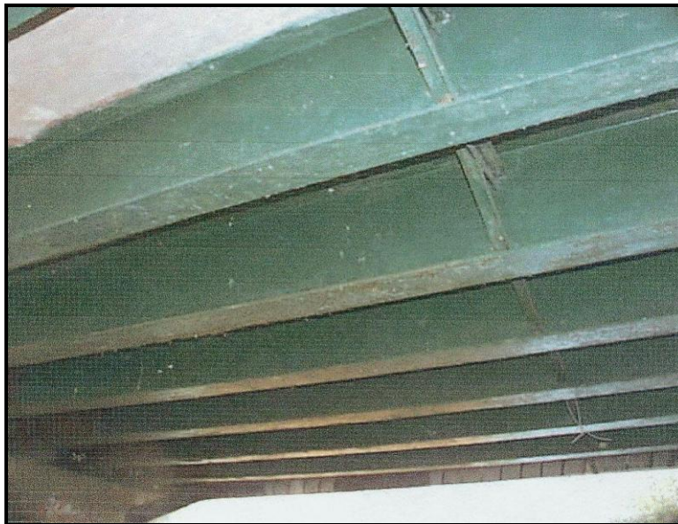
Figure 34. Homestead Avenue Bridge (Bridge 35-N16/90-000.04) in Ohio County, constructed in 1958, illustrating a steel stringer bridge (photograph courtesy of West Virginia Division of Highways)
