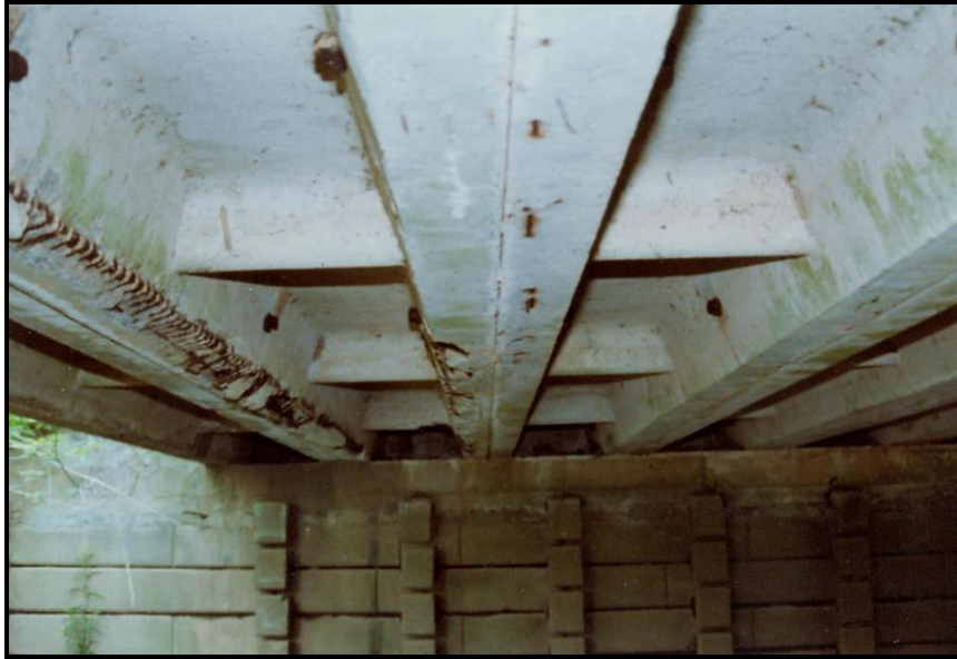
Figure 59. Turkey Branch Bridge (Bridge 40-007/00-006.31) in Putnam County, constructed in 1950, illustrating the underside of a prestressed concrete channel (photograph courtesy of West Virginia Division of Highways)
