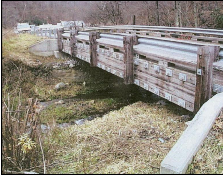
Figure 7. Ashland Timber Bridge (Bridge 24-017/00-006.03) in McDowell County illustrating a timber box beam bridge (photograph courtesy of West Virginia Division of Highways)
