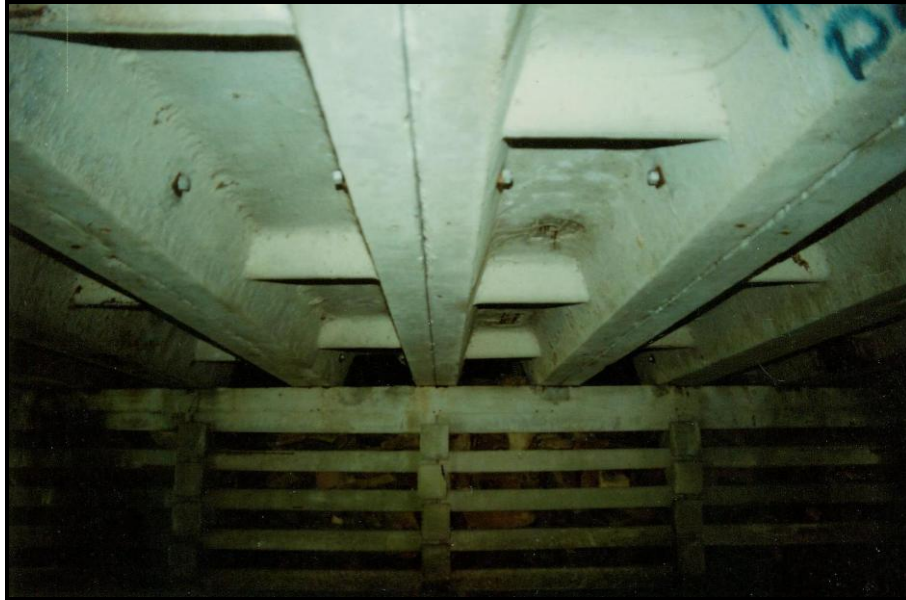
Figure 58. Leadmine Bridge (Bridge 47-007/00-005.35) in Tucker County, constructed in 1957, illustrating a concrete channel bridge (photograph courtesy of West Virginia Division of Highways)
