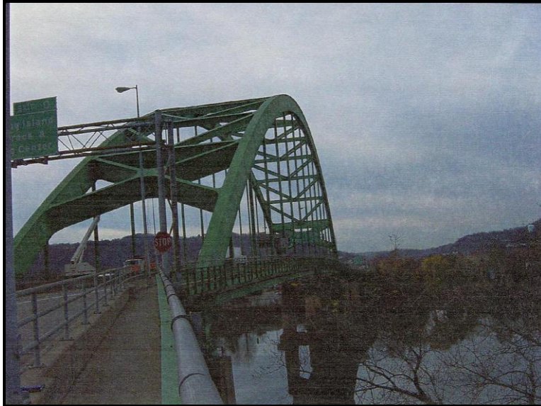
Figure 38. Fort Henry Bridge (Bridge 35-070/00-000.40) in Ohio County, constructed in 1955, illustrating a steel through arch bridge (photograph courtesy of West Virginia Division of Highways)
