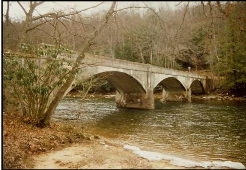
Figure 48. Shavers Fork Arch Bridge (Bridge 42-009/03-000.02) in Randolph County, constructed in 1914, illustrating a closed spandrel concrete deck arch bridge (photograph courtesy of West Virginia Division of Highways)
