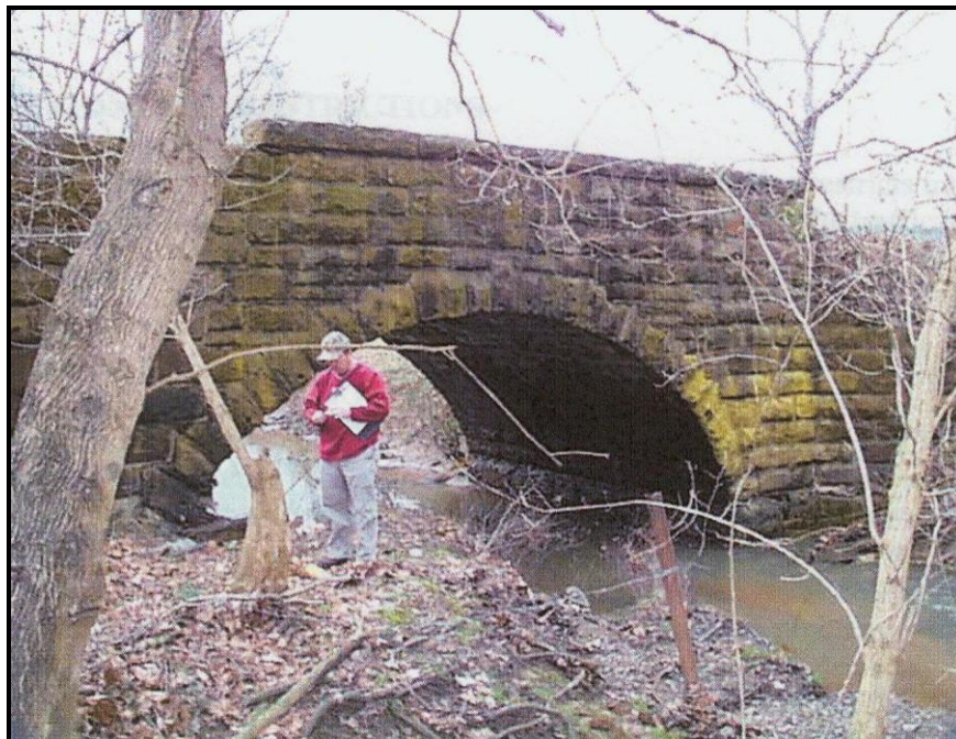
Figure 4. Morris Memorial Arch Bridge (Bridge 06-060/39-000.31) in Cabell County, constructed in 1935, illustrating a stone arch bridge (photograph courtesy of West Virginia Division of Highways)
