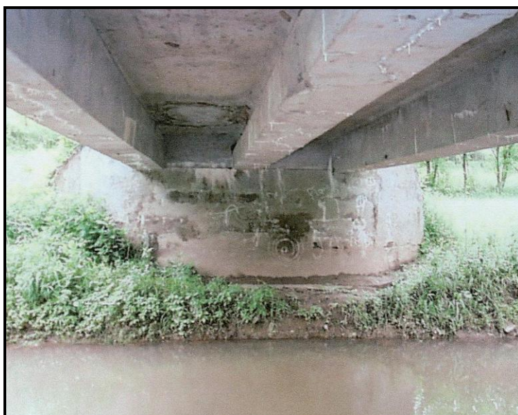
Figure 51. Brush Run Bridge (Bridge 48-006/05-001.34) in Tyler County, constructed in 1920, illustrating a concrete box beam bridge (photograph courtesy of West Virginia Division of Bridges)
