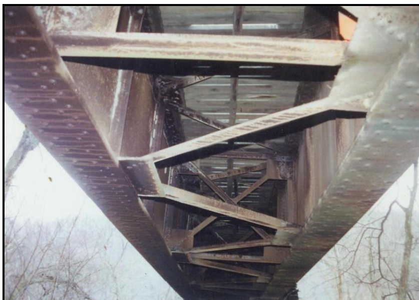
Figure 35. Radnor Railroad Overpass (Bridge 50-052/56-004.64) in Wayne County, constructed in 1911, illustrating a steel box beam girder bridge (photograph courtesy of West Virginia Division of Highways)
