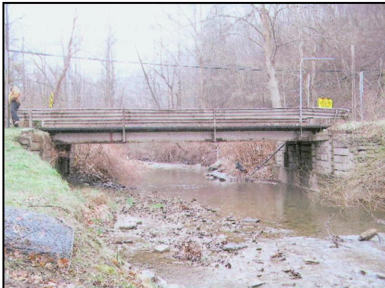
Figure 32. Joes Creek Bridge Number 0.01 (Bridge 03-003/05-000.01) in Boone County, constructed in 1948 illustrating a steel girder/floorbeam (photograph courtesy of West Virginia Division of Highways)
