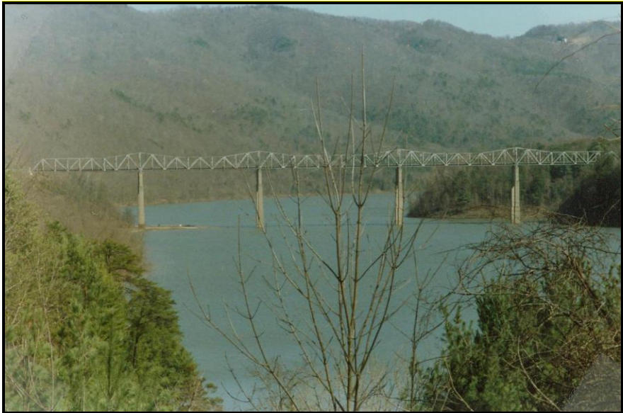
Figure 40. Lilly Bridge (Bridge 45-020/00-009.08) in Summers County, constructed in 1950, illustrating a cantilever bridge (photograph courtesy of West Virginia Division of Highways)
