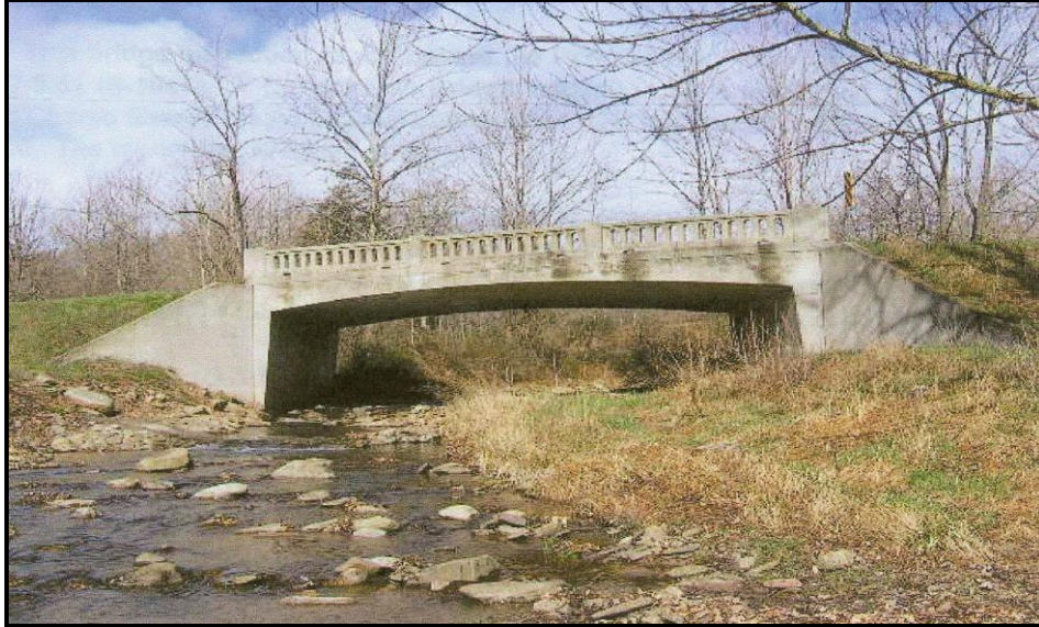
Figure 57. Star Run Bridge (Bridge 12-028/07-008.51) in Grant County, constructed in 1950, illustrating a concrete rigid frame bridge (photograph courtesy of West Virginia Division of Highways)
