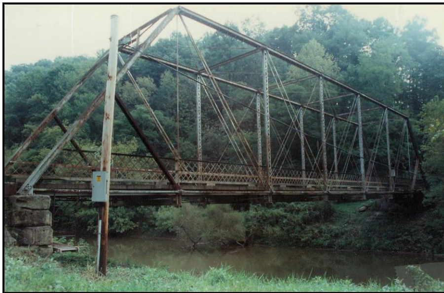
Figure 25. Spruce Run Truss (Bridge 11-119/02-004.34) in Gilmer County, constructed in 1898, illustrating a wrought iron through truss bridge (photograph courtesy of West Virginia Division of Highways)
