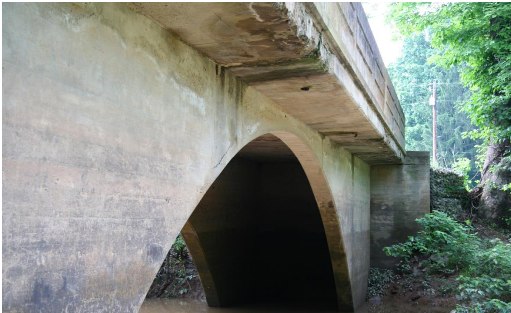
Photograph 1: Example of a spandrel-braced arch with arch ribs that support the deck. (BARS #40A043, District 1, Putnam County)
