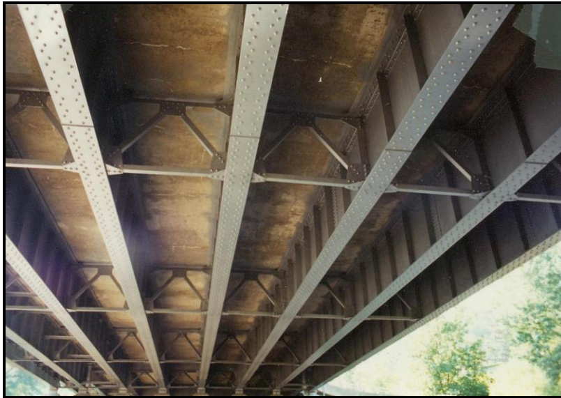
Figure 41. Elbys Bridge (Bridge 35-040/00-000.04) in Ohio County, constructed in 1958, illustrating a steel channel bridge (photograph courtesy of West Virginia Division of Highways)
