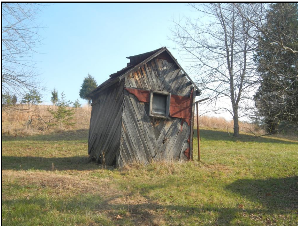
View SE. Wood-framed, Gable-roofed Outbuilding located behind house. Structure has: seamed metal roof surfacing, diagonal wood board sheathing, and remnants of Insulbrick siding (faux-brick, tar-impregnated sheeting used ca. 1930-1960s). Photo Taken 12-4-2013.
