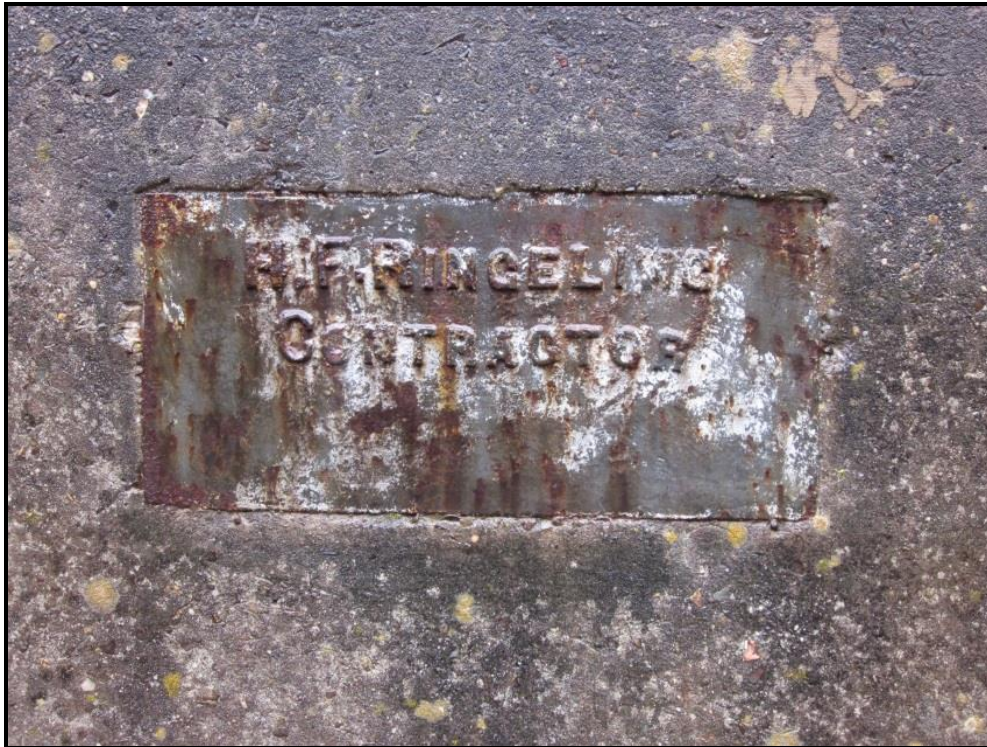
Inset Metal Plaque (approx. 14" x 6.5") at Northeast Wing Wall that reads "H. F. RINGELING / CONTRACTOR." View Northwest. Photo taken 10-11-2013.
