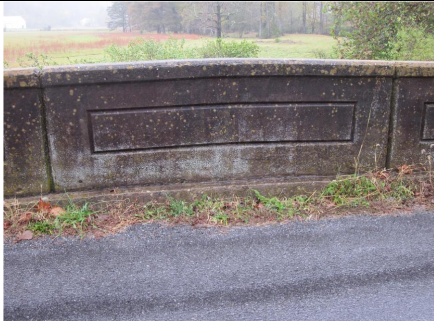
7. Bridge - Railing/Parapet at North Side, Highlighting Typ. Peaked Central Panel of Railing with Incised Rectangular Motif; View North/NE
