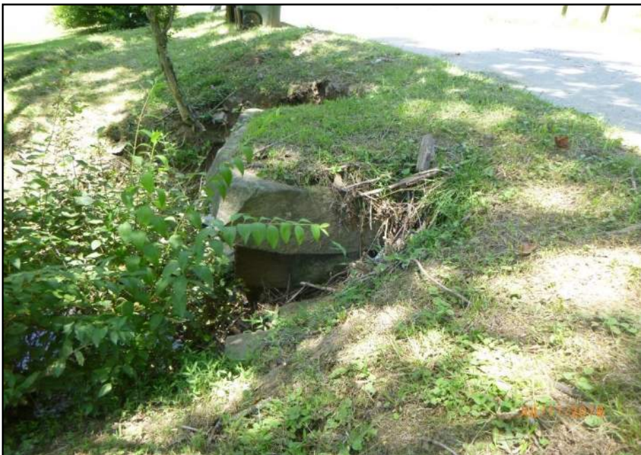
Detail of top and east elevation of the stone culvert.
