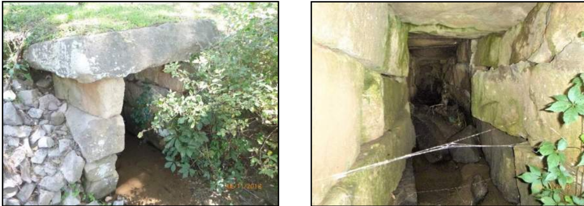
Image 1: Hallsburg Road Stone Culvert, exterior, outlet side, and interior.
