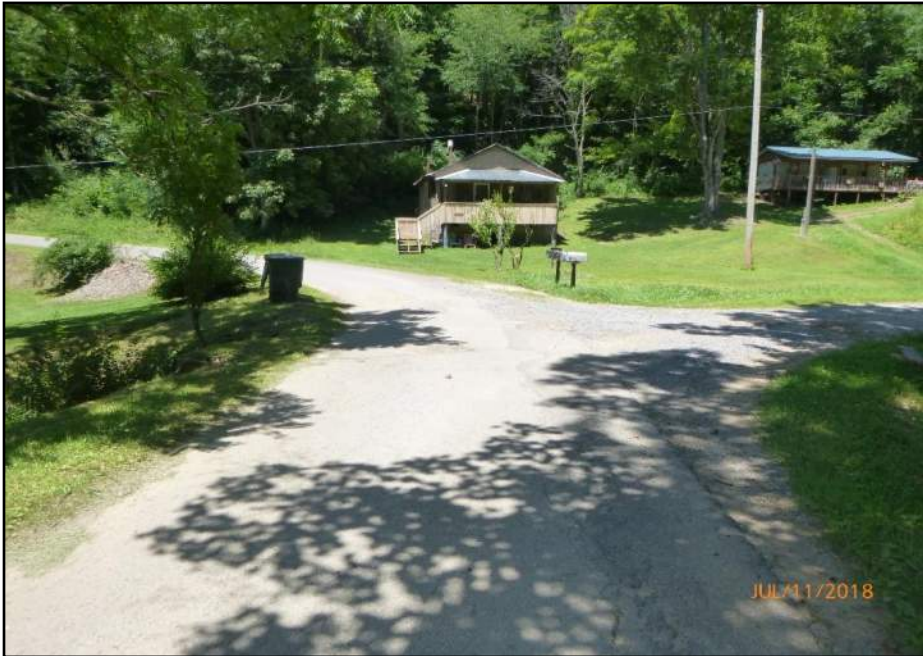
East approach to culvert on CR 42.
