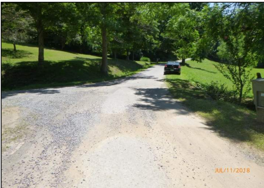
West approach to culvert on CR 42.
