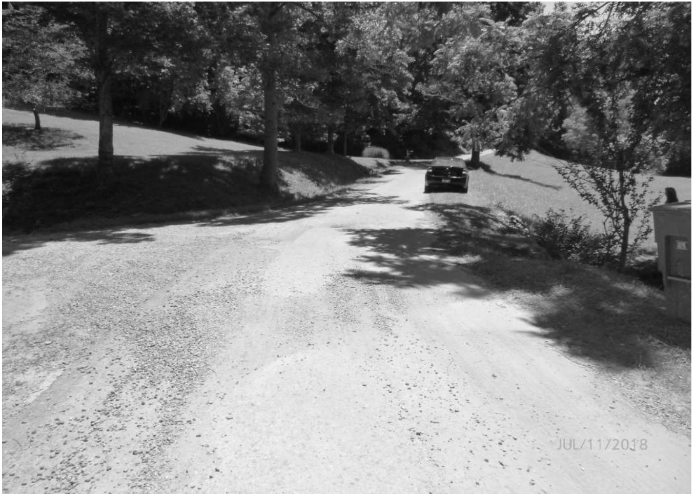
Photo 1 Hallsburg Road Culvert Clay County County Route 42 over tributary of Big Otter Creek South approach to culvert
