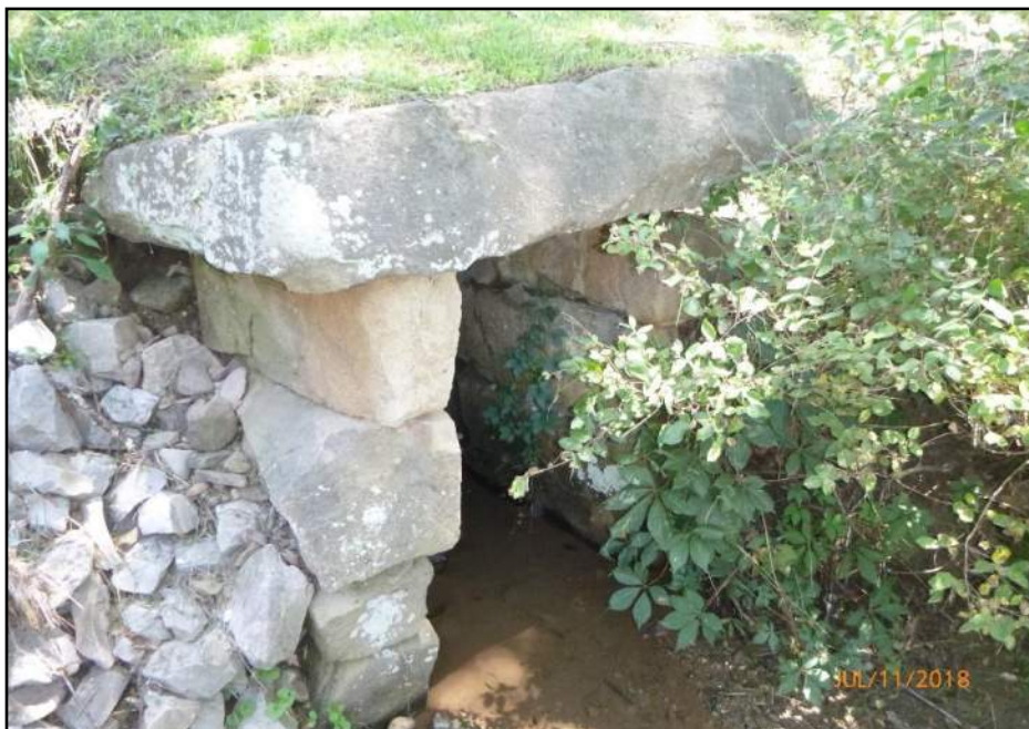
South outlet of Hallsburg Road Culvert.
