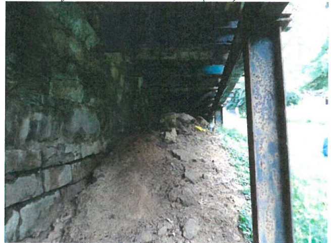
Metal support beams added to underside of sidewalk for additional support. (2016)
