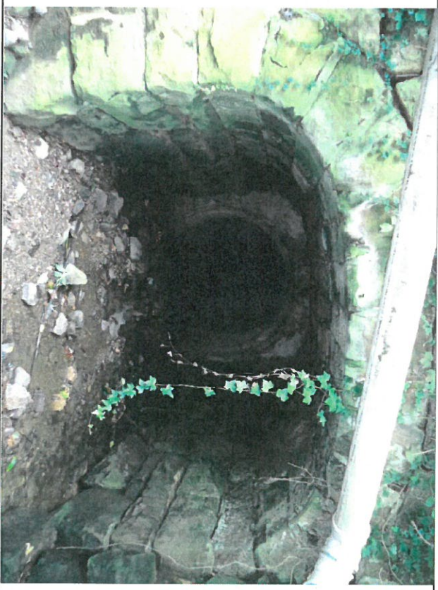
12. Stone arch drainage inlet on eastern side of National Road/US40.
