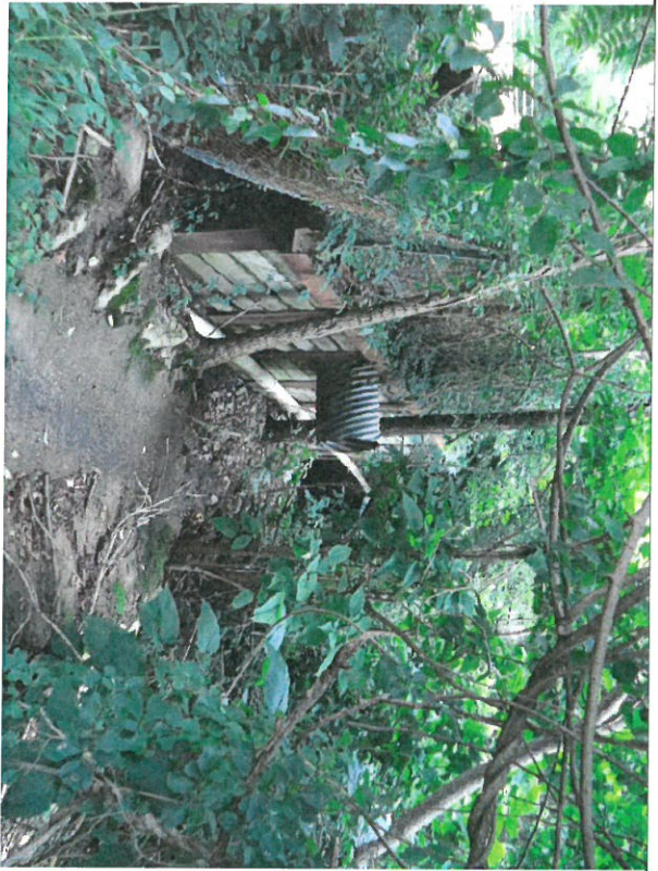
9. Steel/timber retaining wall, eastern side of roadway.
