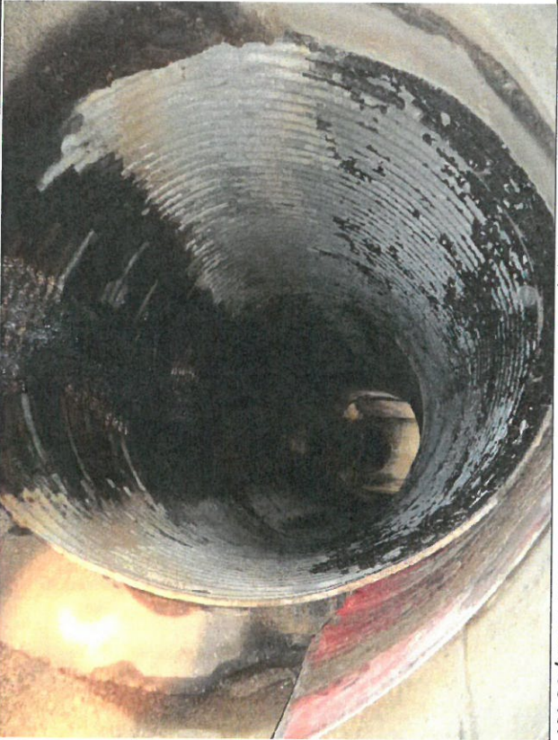
15. Concrete pipe- corrugated metal pipe connection under cantilevered sidewalk & fill material.
