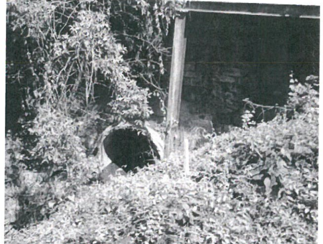
Concrete pipe that replaced stone arch culvert. (1983)
