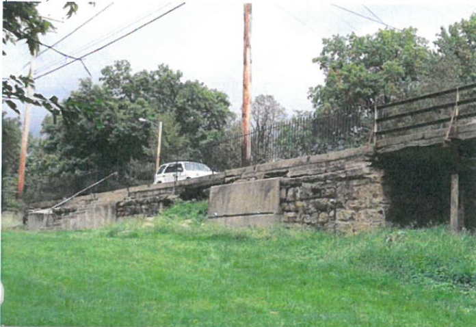
Concrete reinforcement, drainage, and stairs on northern end of wall. (2016)
