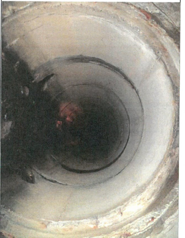
14. Concrete pipe under National Road/US40.
