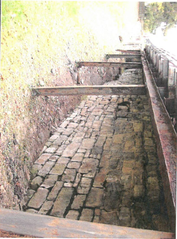
5. Detail of cantilevered sidewalk connection with stone wall.
