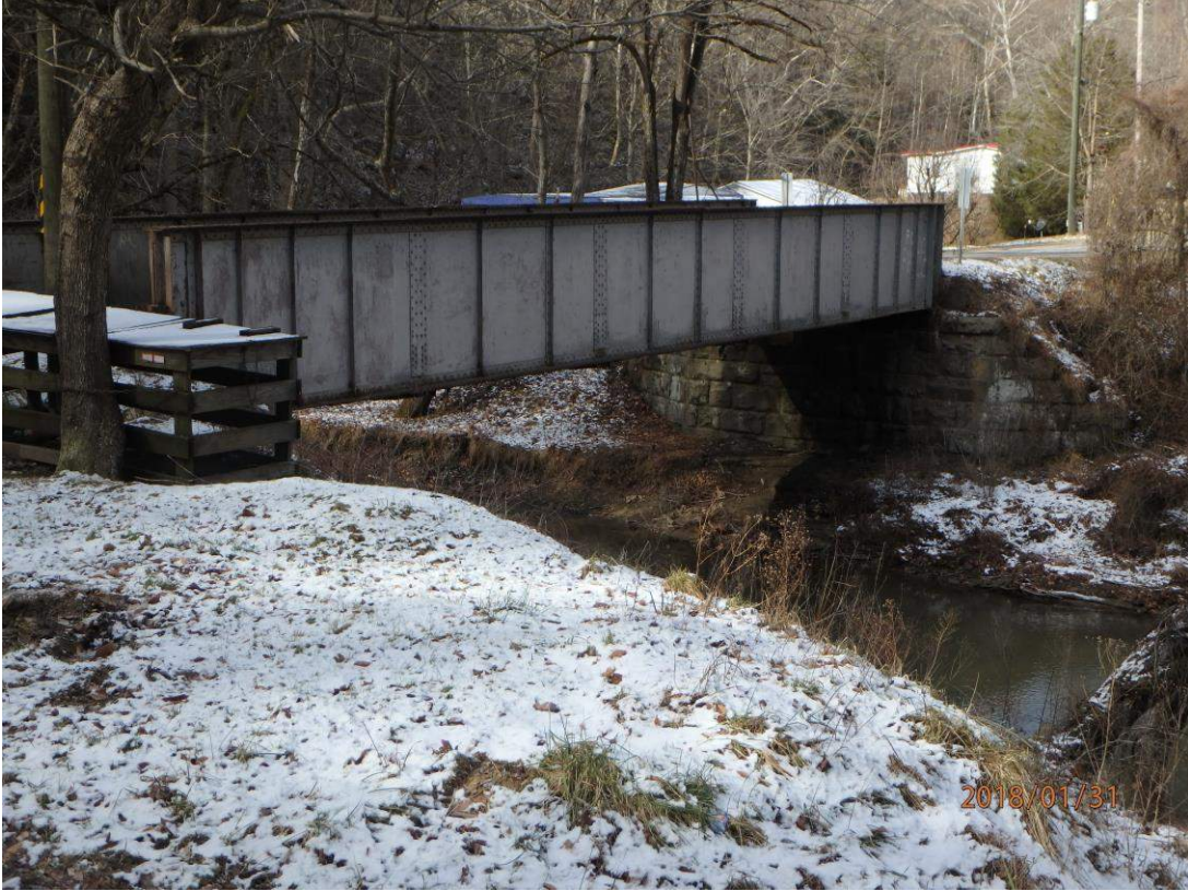
Photo #9: Breedon Tunnel Girder
