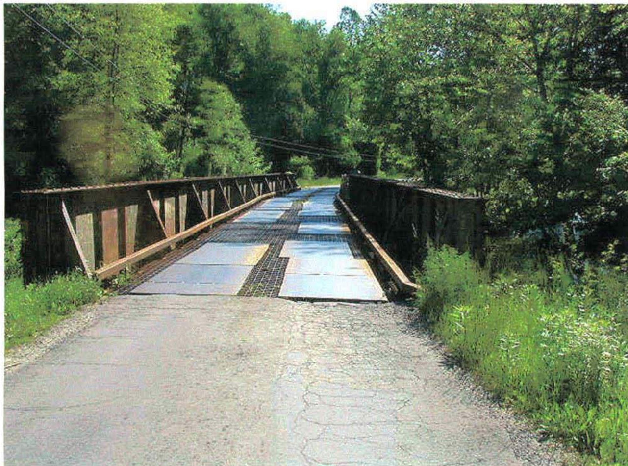
deck condition from eastern approach on CR 3/5
