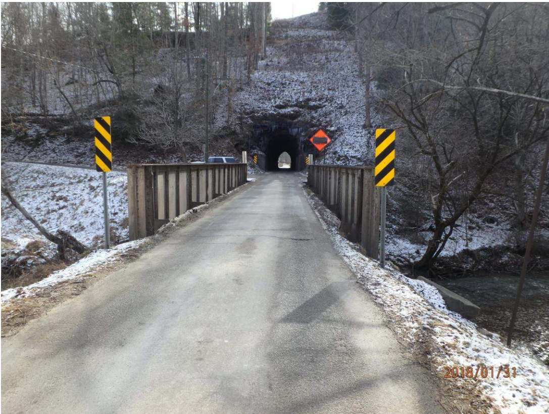
Photo #10: Breedon Tunnel Girder and Breedon Tunnel
