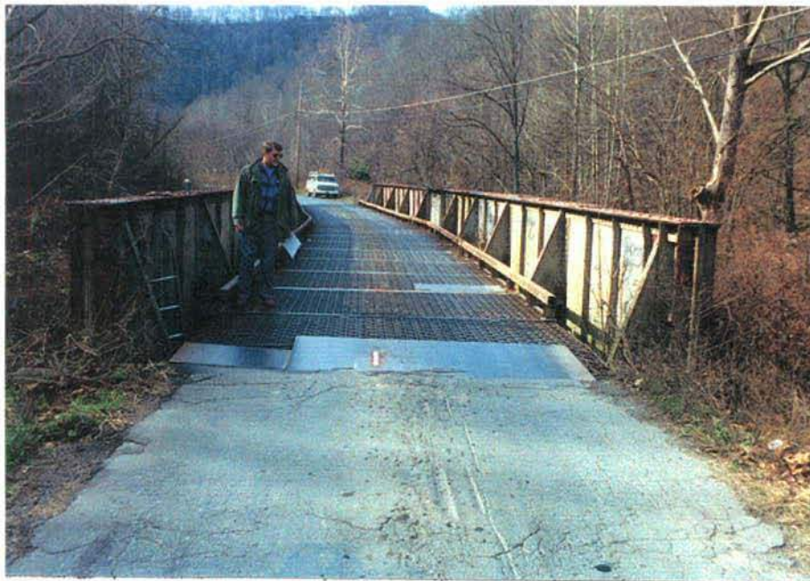
ROADWAY VIEW FROM ABUTMENT NO. 1
