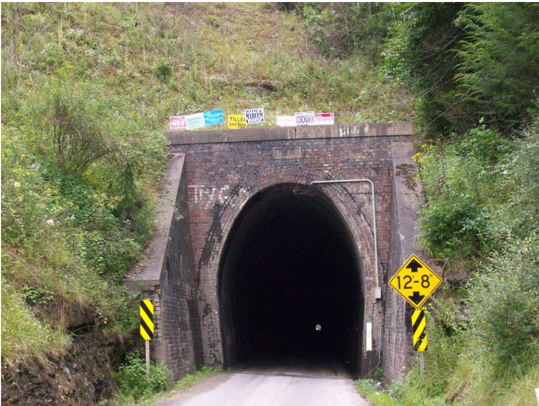
Photo #2: Dingess Tunnel, South End
