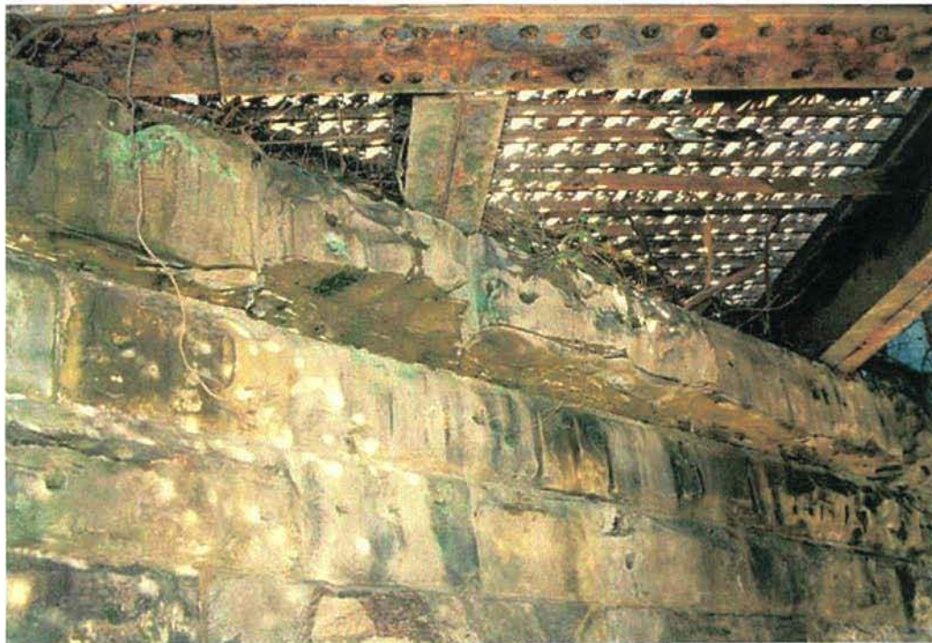
STONE DELAMINATION PIER CAP- P-1 ABUTMENT NO. 2 SIDE
