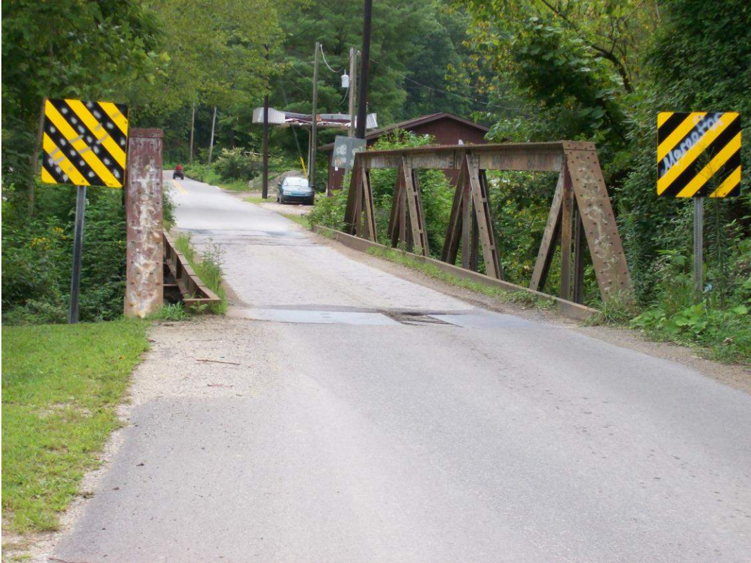
Photo #5: Big Rock Pony Truss
