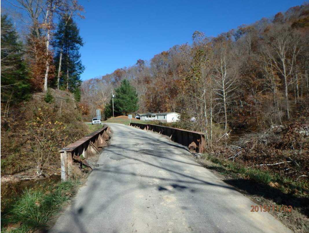
Photo #7: Breeden Through Girder
