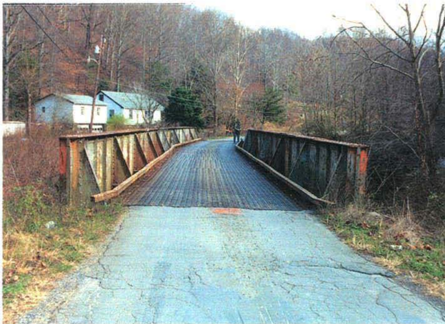
ROADWAY VIEW FROM ABUTMENT NO. 2
