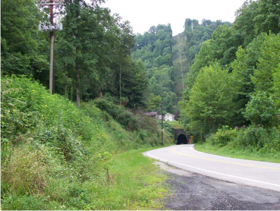
Photo #3: Dingess Tunnel, North End
