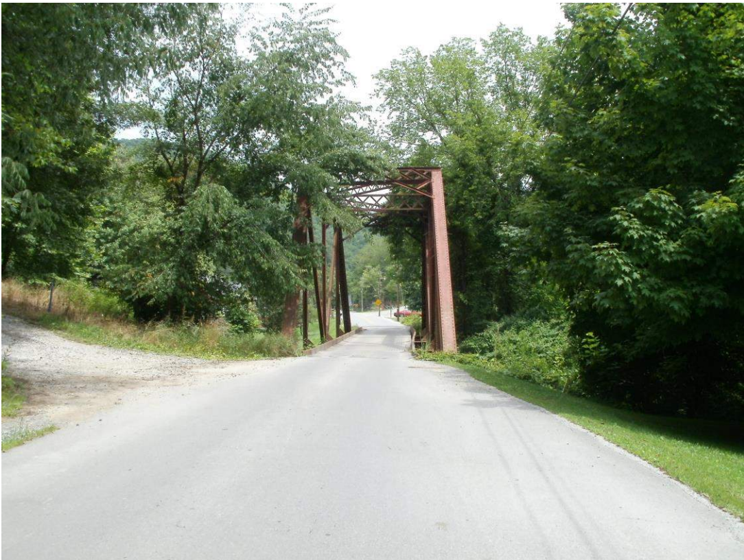
Photo #6: Kirk Thru Truss
