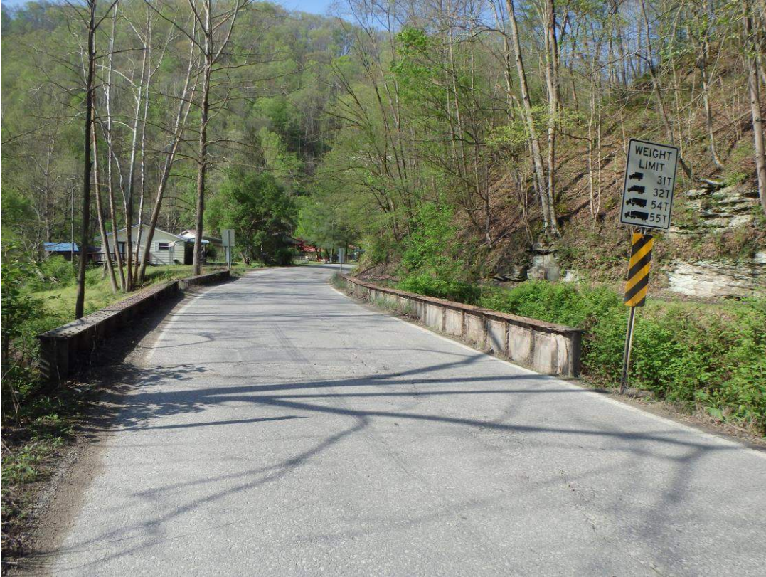
Photo #1: Laurel Creek Girder
