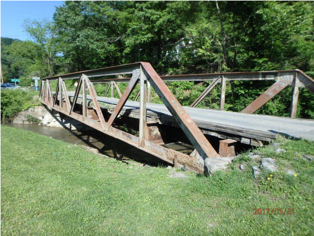
Photo #4: Bailey Branch Pony Truss
