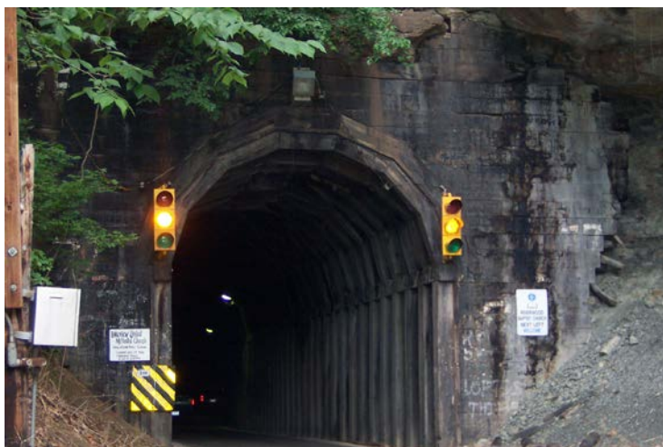
Southern End of Tunnel
